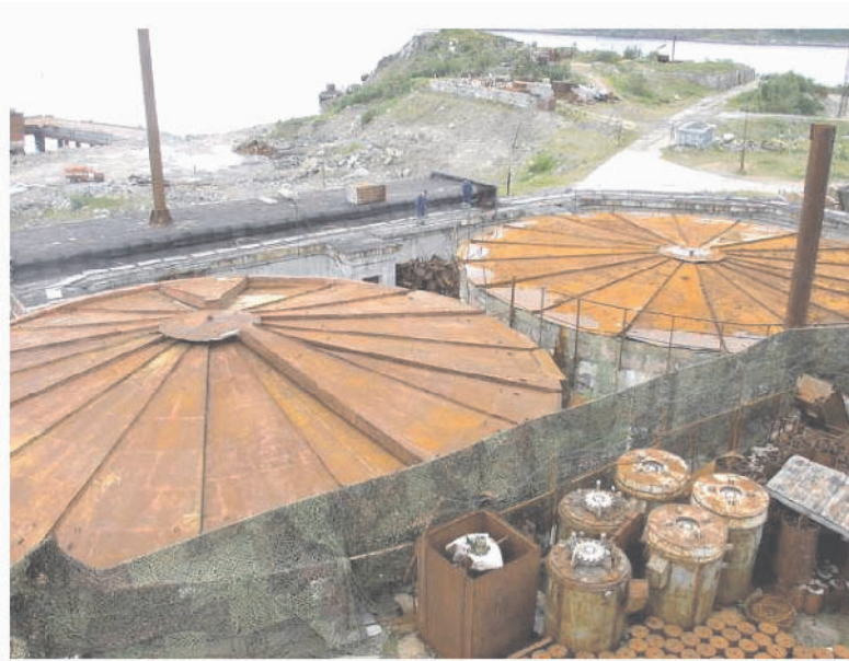
Figure 13. SNF storage facilities at CMB in Andreeva Bay
