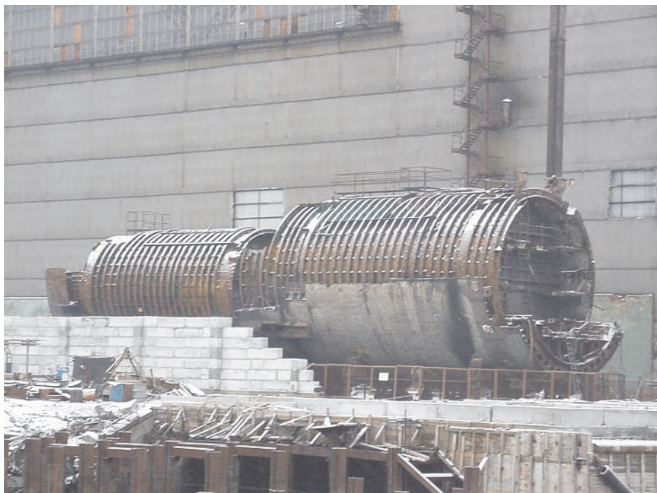
Figure 10. One-compartment RC units on slip-way
