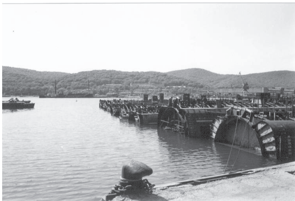
Figure 9. Three-compartment RC units of dismantled NSs afloat in Razboinik Bay
