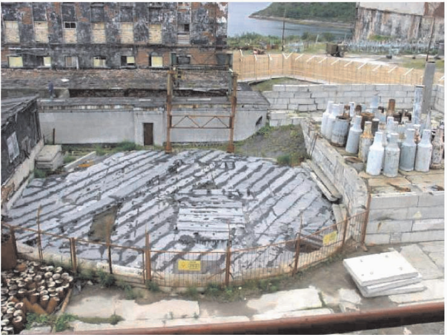
Figure 2. Dry Storage Unit 1 (facility 3A)
