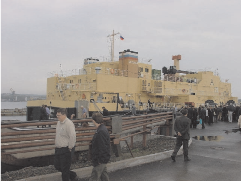
Figure 12. LRW processing barge “Landysh”
