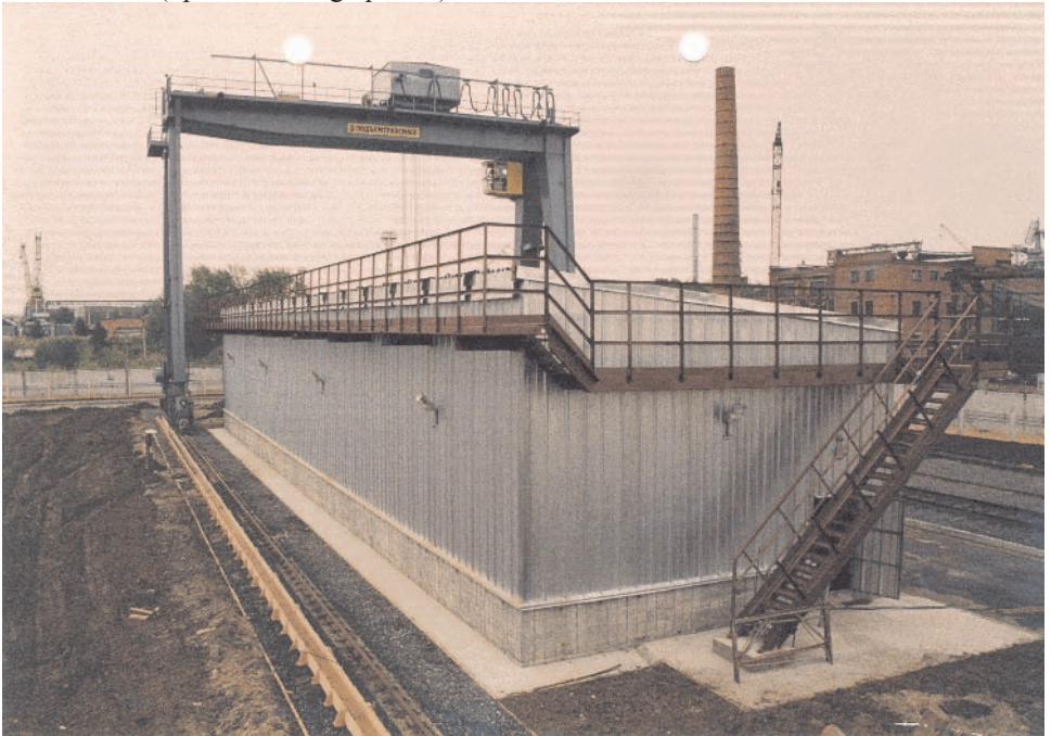
Figure 6. Interim-storage pad for containers with SNF at “On-shore Defueling Facilities”
