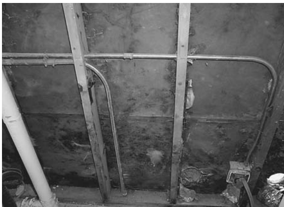
Figure 7.3 Mold growing on and into wood. (Courtesy of Aerotech Laboratories, Phoenix, AZ.)
