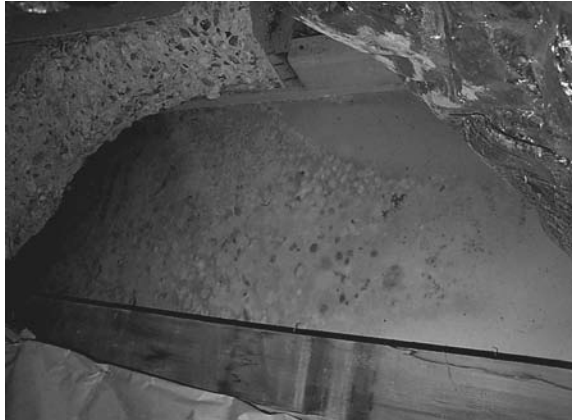
Figure 7.7 Material under carpet is difficult to clean. (Courtesy of Aerotech Laboratories, Phoenix, AZ.)
