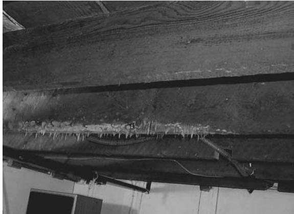
Figure 7.4 Mold growing on and into wood. (Courtesy of Aerotech Laboratories, Phoenix, AZ.)
