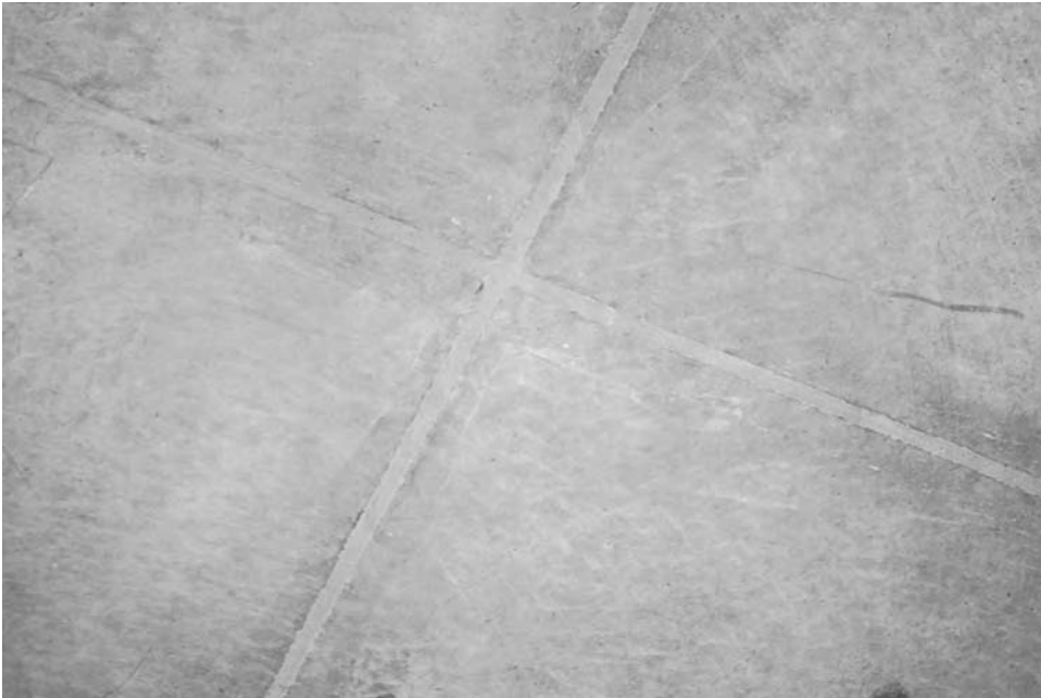
Figure 15.6 Warehouse floor joints filled with semi-rigid epoxy
