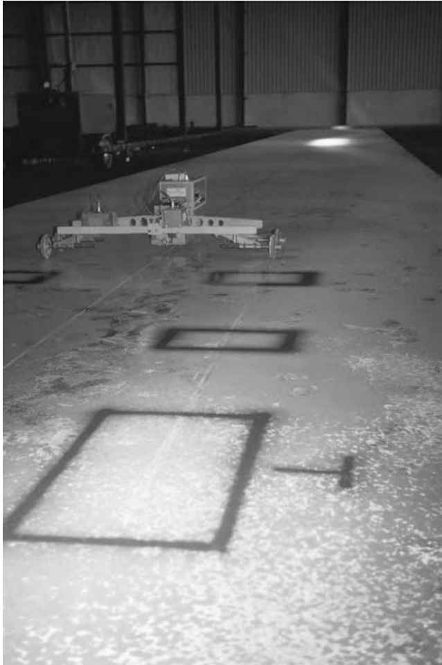
Figure 19.9 Superflat construction – marking a new slab for grinding, after testing with a profileograph
