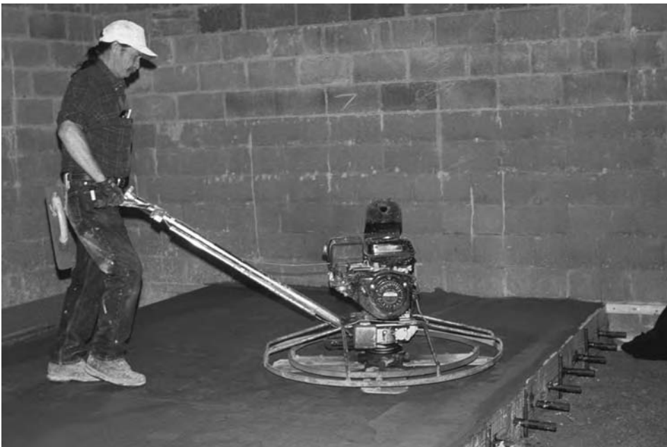
Figure 17.6 Walk-behind power trowel machine
