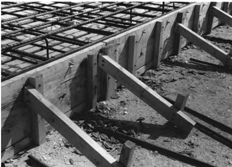
Figure 11.13 Heavily braced timber form
