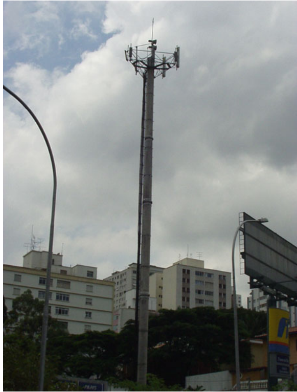
Fig. 1 Typical pre-cast RC telecommunication tower
