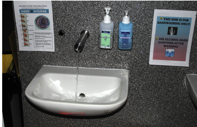
Figure 17.1 Stainless steel water tap outlet. This type of outlet can be easily removed from the wall mounting for cleaning, decontamination or sterilisation.
