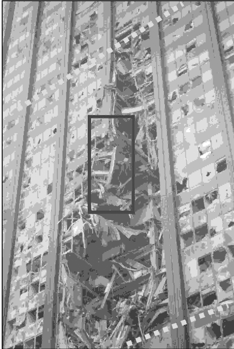
Figure 12a. Damage to the northern face of the building between tenant levels 23 and 10—view of damage zone between levels 23 and 10.
