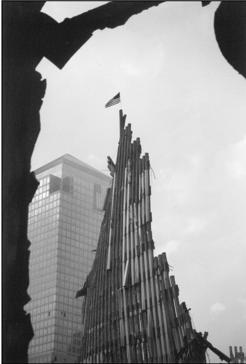
Figure 14. View of the tower 2 façade looking northwest from the foyer of the building.
