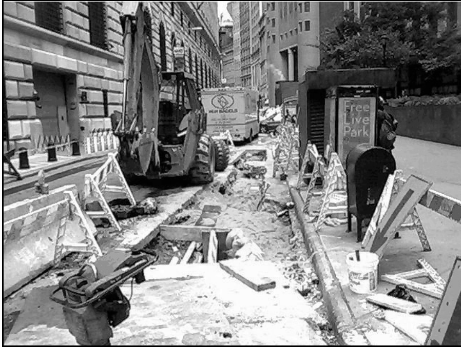
Figure 3. Work to restore public infrastructure was much in evidence.
