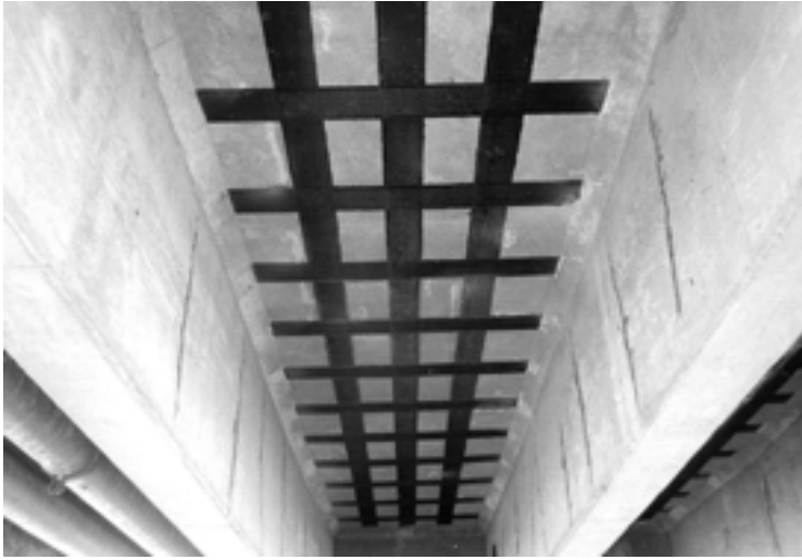
5.2 Application of composite strips to the soffit of a bridge deck.
