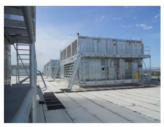
**FIGURE 25.8** 160,000 cfm IASEs with heat wheels removing a total of 10 mW of heat from a data center.
