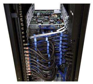
FIGURE 26.10 Water pipes and manifolds. Courtesy of Asetek.
