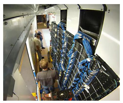
FIGURE 4.12 Front-cabled racks being installed in an MDC at IT factory. Courtesy of Hewlett-Packard Company.
