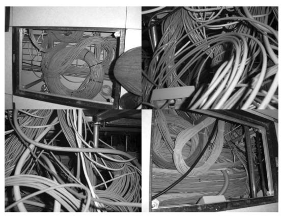
FIGURE 17.12 Classic unstructured cabling. Courtesy of Future Facilities.
