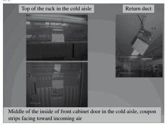
**FIGURE 16.4** Photos of different coupon placements: (a) examples of inside outdoor air and (b) example of inside indoor air [10].
