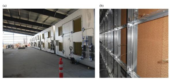
**FIGURE 25.3** (a) Cooling system using bank of direct evaporative cooler units at the end wall of a data center; (b) The array of evaporative cooling media.
