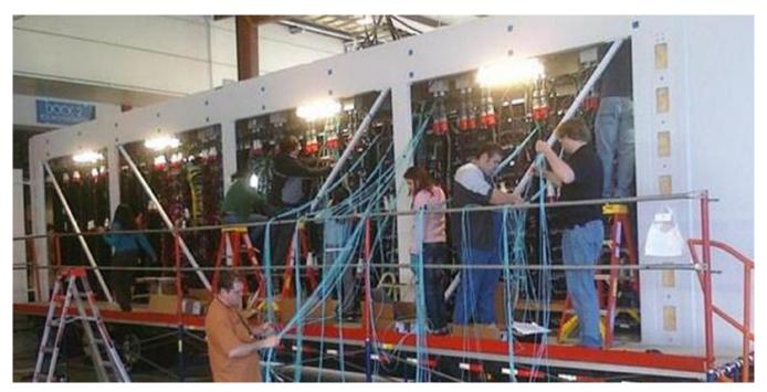
FIGURE 4.15 Complex IT wiring could be much faster in an MDC factory environment. Courtesy of Hewlett-Packard Company.
