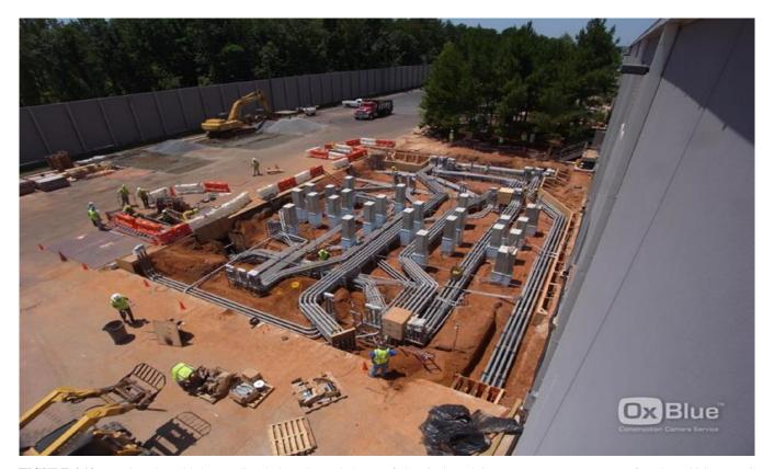
**FIGURE 4.19** It takes about 30 days to dig a hole and prep 2.5 MW of electrical conduit to prepare to pour concrete for a 2 N 700 kW MDC expansion to an existing data center. Courtesy of Hewlett-Packard Company.
