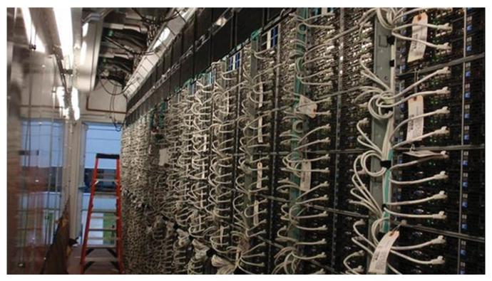
**FIGURE 4.2** An MDC being configured and pretested with IT. This example shows twenty 18 kW racks all with their own UPS. This IT module can be fed by site chilled water, or is supported by another module specifically configured to deliver chilled water, or simply condenser temperature water for additional energy savings. Courtesy of Hewlett-Packard Company.
