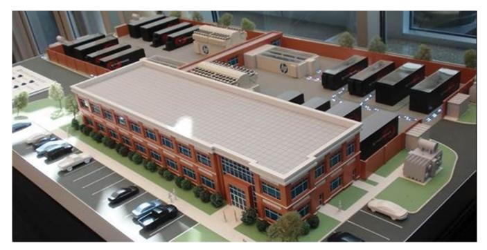
**FIGURE 4.1** Example of an MDC. Each of the *white* and *black boxes* behind the office space is a manufactured module, and some are totally preassembled. Any one white IT module with its integrated cooling is powered by the four black modules, providing continuous redundant power. That row of five boxes is one 500–1000 kW complete MDC. Courtesy of Hewlett-Packard Company.
