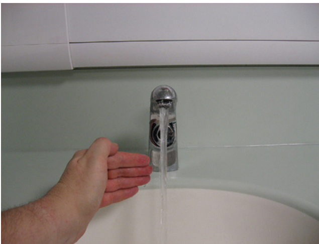
Figure 8.2 Sensor-operated tap fitted on a handwash basin; note there is no overflow.
