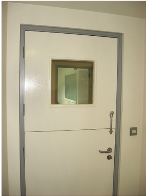
Figure 7.5 Two-part stable door for controlled access. The top part of the door can be opened and used as a pass-through instrument hatch.
