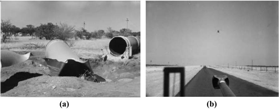
Photo 1. The Cunene River Basin was a theatre of military action during the Namibian War of Independence, and the Angolan Civil War. The water transfer pipe from the Cunene to the Cuvelai system was bombed on occasion (a), necessitating protection by combat patrol in the Ruacana area (b).
