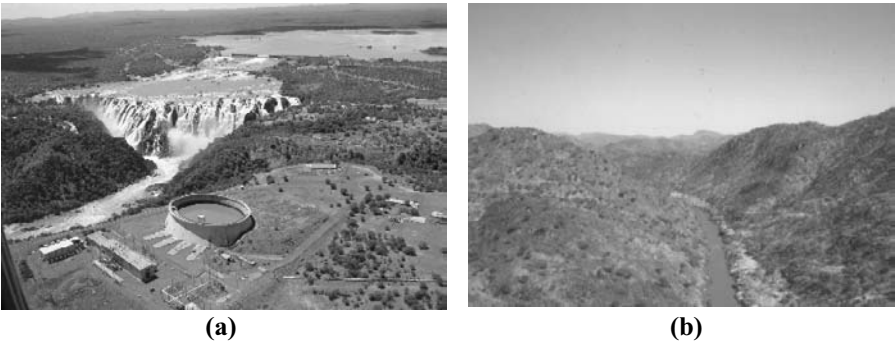
Photo 4. Shared water resources play a major role in developing both Angola and Namibia, particularly during post-conflict reconstruction. The Cunene river flows over the Ruacana Falls (a) and makes its way down to the future site of the Epupa Falls Dam (b), where it becomes a linear oasis in the desert.
