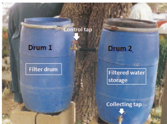
Fig. 9.6 Sand filter drums. Source: Yongabi and Lewis (2011b)
