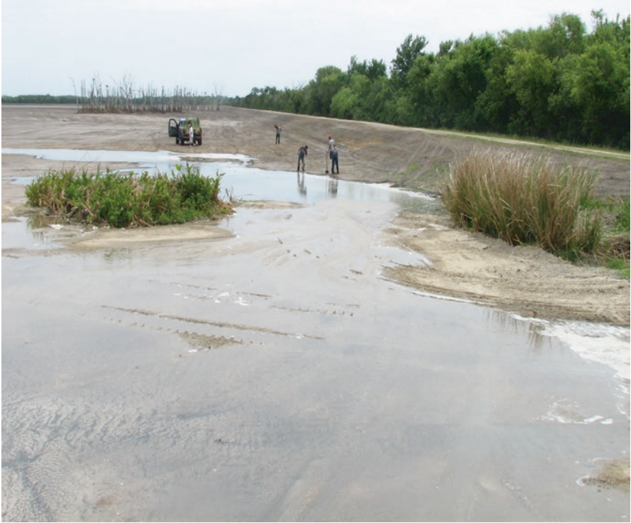
Fig. 4.8 Crews plant vegetation in the now de-mucked cells
