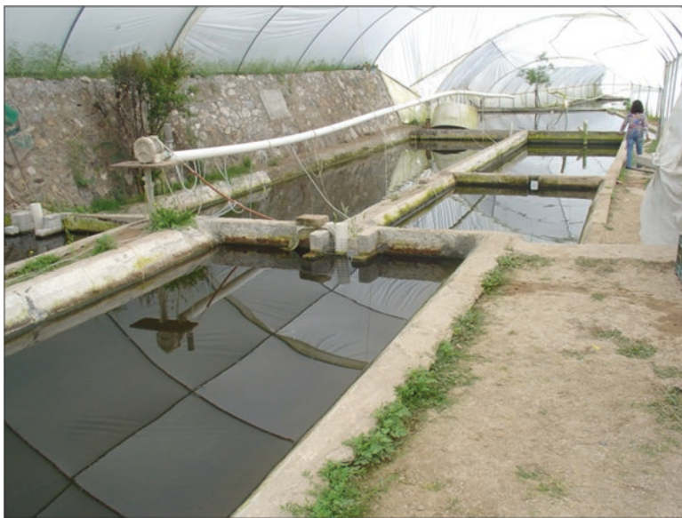
Fig. 8.4 Stabilization ponds (foreground) and holding tanks for pisciculture at the La Coralilla treatment wetland during Stage IV of the project. Photo by Eliseo Cantellano
