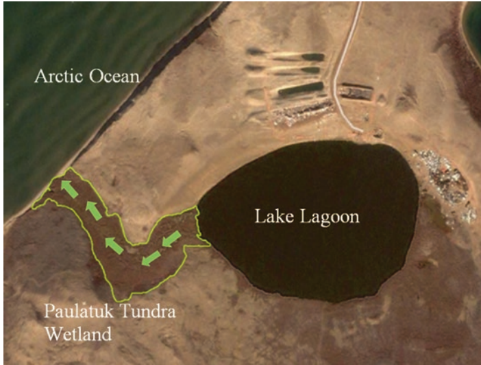
Fig. 3.7 A Google Earth image of the wastewater treatment area located in Paulatuk, NU, and the lake lagoon that receives the hauled truck raw wastewater
