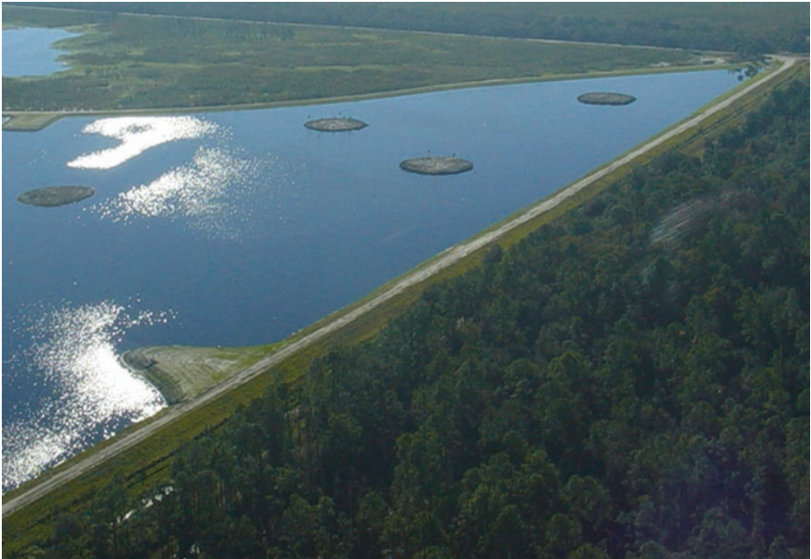
Fig. 4.9 The northern flow train back in operation after de-mucking operation
