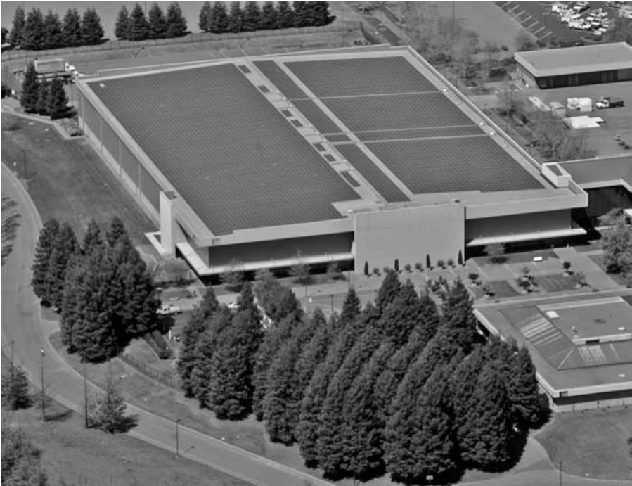
Figure 8.3 A large 1.14-MW solar (photovoltaic) panel array in 2006 at Sonoma Mountain Valley (California) was installed as a start to achieve 100% of power with renewable energy and zero carbon emissions One Planet Living (OPL) goals. Courtesy Sonoma Mountain Village -SOMO.
