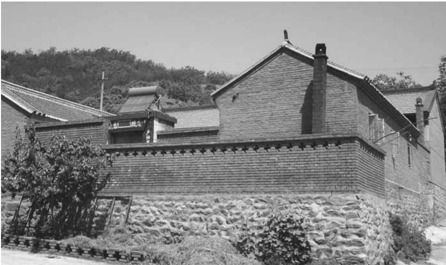
Figure 8.9 Installation of concentrated solar water heater on a rural home in Beijing province, China. The water heaters were provided by the government. Photo V. Novotny.
