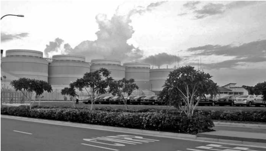
Figure 8.21 Sludge digesters in the Changi Water Reclamation Plant in Singapore, designed by CH2M HILL (photo V. Novotny).
