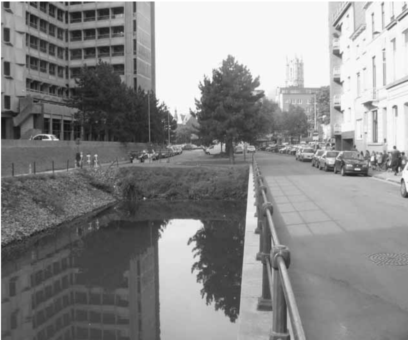
Figure 9.7 A partially covered historic canal in Ghent, Belgium. Photo V. Novotny.
