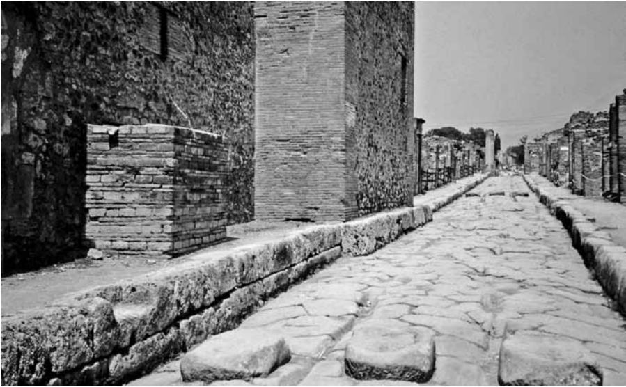
Figure 1.3 The Via Abbondanza in the Roman city of Pompeii near Naples in Italy. Stepping stones document that the street was used for drainage. The street also had water fountains conveniently located along the street so citizens and merchants did not have to go far for water. Overflow from the fountains washed the streets (Photo V. Novotny).
