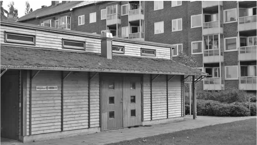
Figure 3.14 The Augustenborg neighborhood has 1450 square meters of green roofs for stormwater management and to express the project’s ecological aesthetic and commitment to sustainability. Here, the green roof is added to a “resource house” to support organic composting and material recycling. Photo: Jack Ahern.
