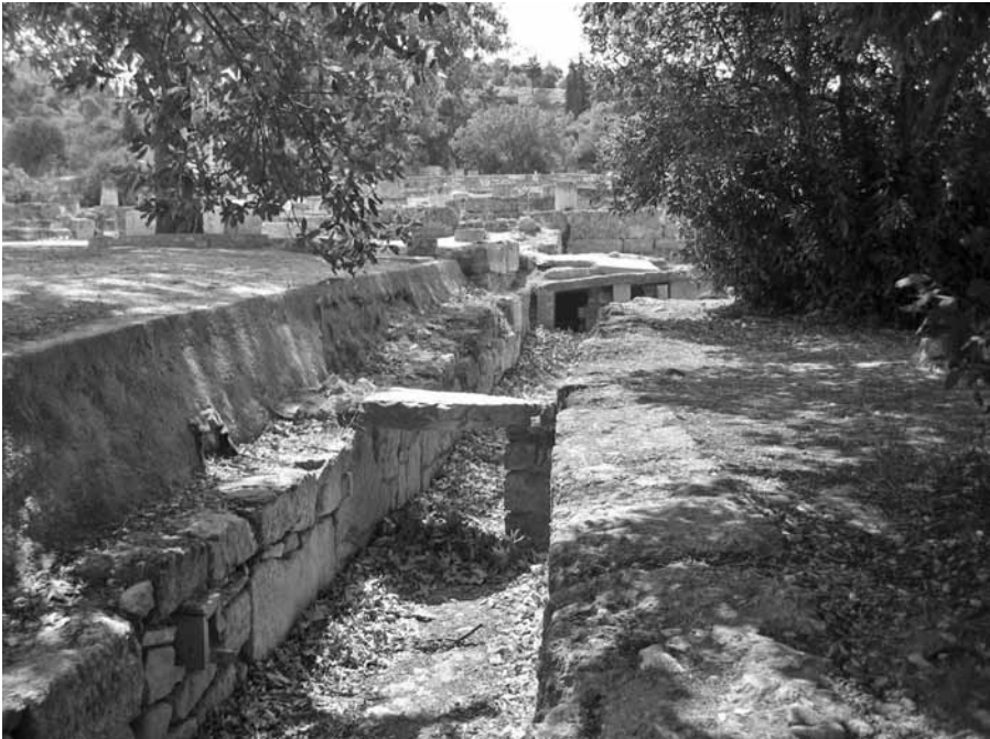
Figure 1.2 Drainage systems in ancient Athens (ca. 500 B.C.). This 1 m x 1 m surface drainage channel is located in the agora (gathering place) of the ancient Greek metropolis (Photo V. Novotny).
