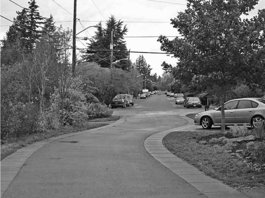
Figure 3.9 The Street Edge Alternative (SEA Street) in Seattle, Washington, is a natural drainage system (NDS) designed to direct street runoff from a narrowed street pavement to planted infiltration swales. Note the adjacent street in the background showing the pre-SEA Street condition with wider road pavement and conventional stormdrains. Photo: Jack Ahern.
