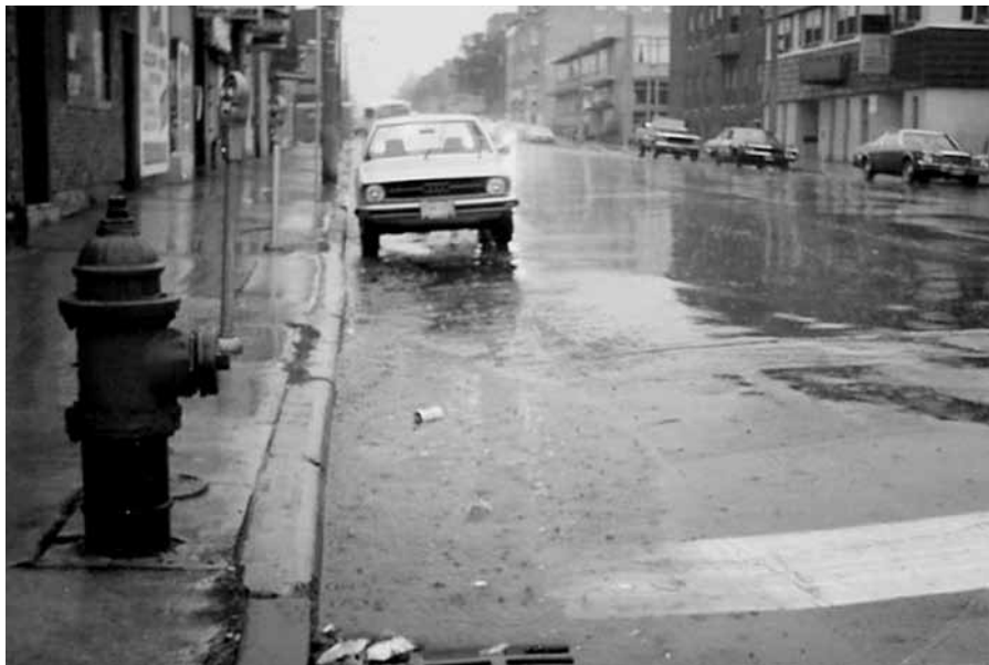
Figure 4.4 Curb and gutter installation on urban streets and roads results in accumulation of pollutants near the curb and subsequent washoff into catch basins. With such practices in highly impervious urban neighborhoods, there is no attenuation of pollutants or reduction of urban runoff rates. Photo V. Novotny.
