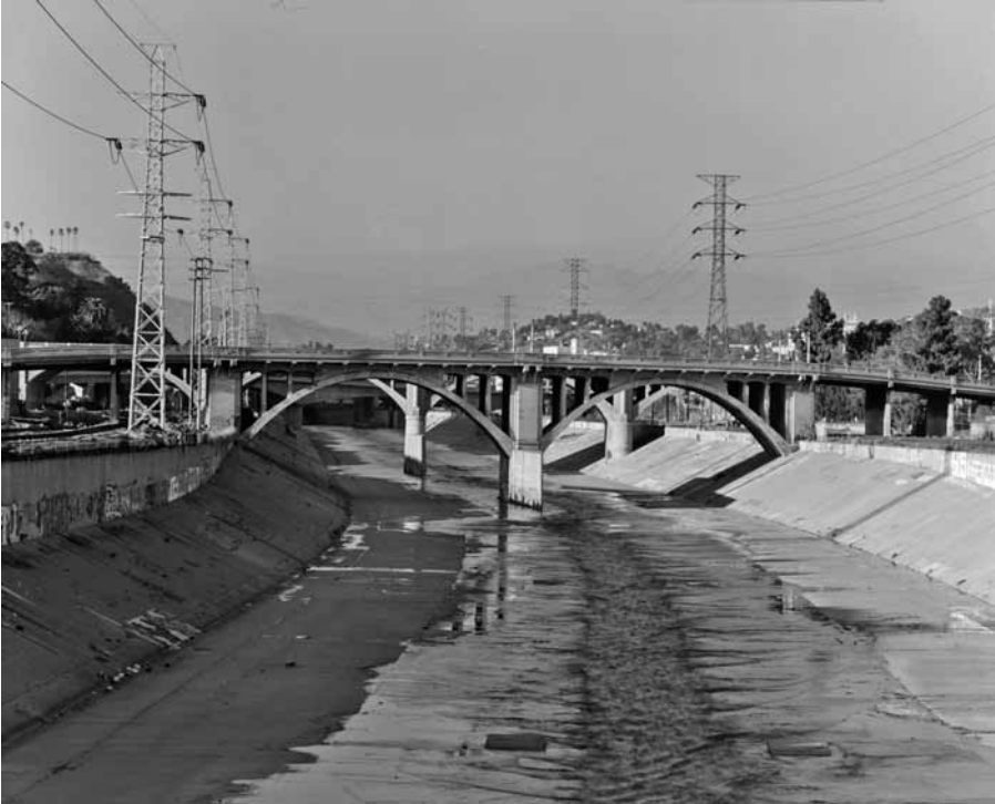
Figure 1.16 Los Angeles River. It was once a natural river, but it was converted into a lifeless flood conveyance channel with no connection to population living nearby. The river in some sections is a perennial effluent dominated channel; in some other sections, it has no dry-weather flow. Source: US Army Corps of Engineers.
