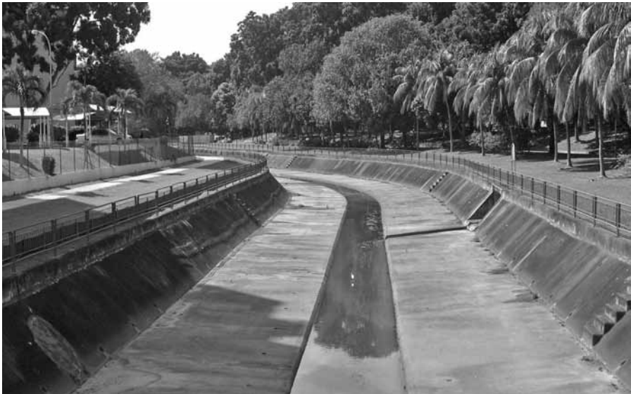
Figure 9.24 The Kallang River in Bishan Park in Singapore in 2009. Photo CDM.
