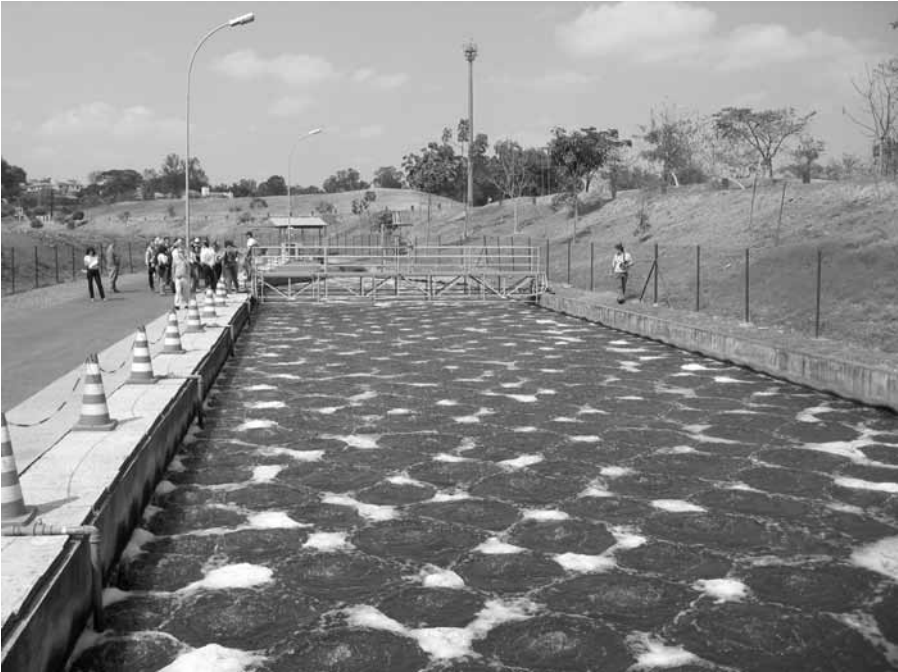
Figure 10.10 A flotation treatment plant (energy demanding) treating low flows of a local urban stream in Belo Horizonte, Brazil. Photo V. Novotny.
