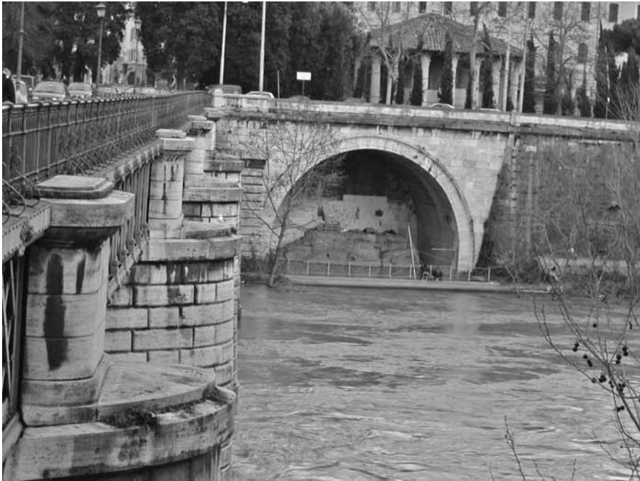
Figure 1.6 Outlet of the Roman sewer, the Cloaca Maxima (Largest Sewer) into the Tiber River. The sewer is functioning today, but a barrier was installed to prevent entry because of security concerns.
