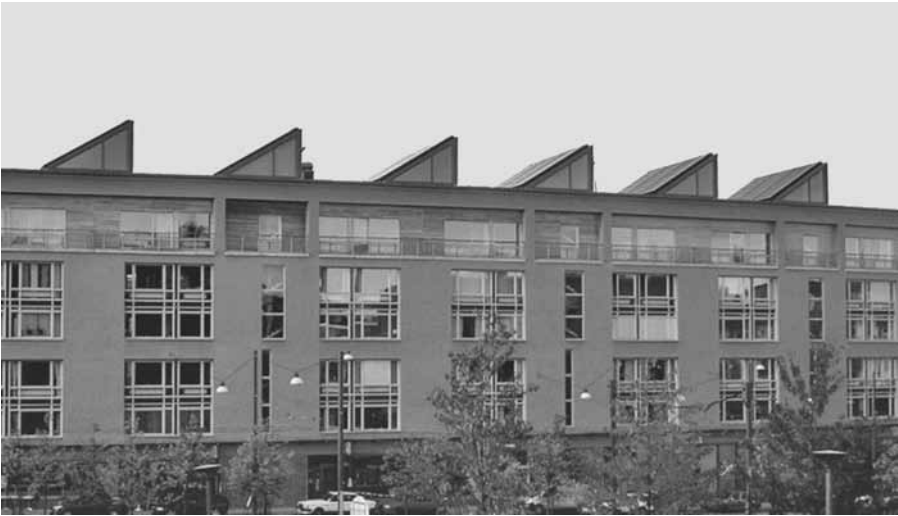
Figure 8.10 Solar panels in Hammarby Sjöstad in Stockholm. Picture credit Malena Karlsson, GlashusEtt, Stockholm
