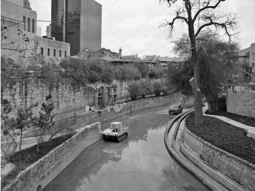
Figure 9.6 The beautified San Antonio River is a concrete impounded channel with very poor habitat and water quality (zero water environment benefits).
