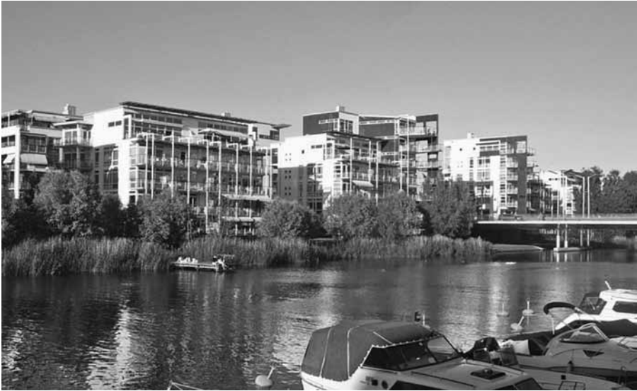
Figure 11.1 Hammarby Sjöstad with a central canal (Courtesy Malena Karlsson, GlashusEtt).
