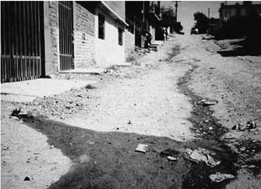
Figure 5.11 Gray water discharged into street drainage in Tijuana, Mexico. The dark color indicates foul anaerobic conditions, in contrast with still oxygenated fresh gray water input from the house on the left. Photo and credit Art Ludwig, 2009.
