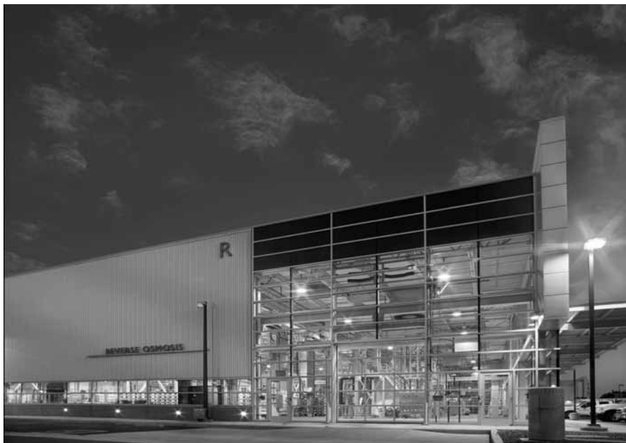
Figure 6.11 Reverse osmosis water reclamation plant, treating used water of the Orange County, California, GWR system (photo courtesy CDM).
