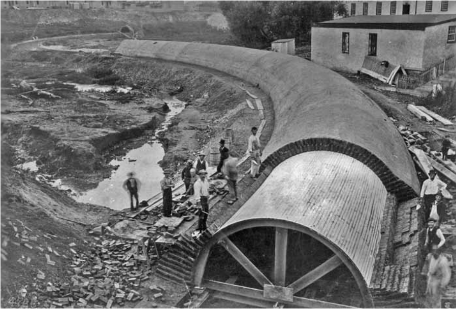
Figure 1.11 Converting Mill Creek into a sewer in Philadelphia (PA) in 1883 (photo provided by the Philadelphia Water Department Historical Collection).
