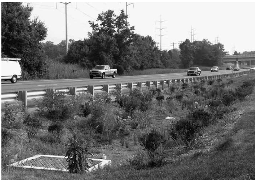
Figure 4.14 A simple extended dry/bioretention cell used for treatment of smaller flows. Courtesy Delaware Department of Transportation
