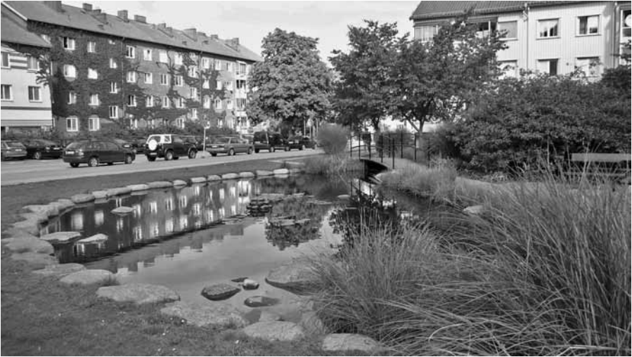
Figure 3.13 The Augustenborg neighborhood was retrofitted to manage stormwater on-site through a series of best management practices, including this attractive planted wet retention pond to store, infiltrate, and clean stormwater. Photo: Jack Ahern.
