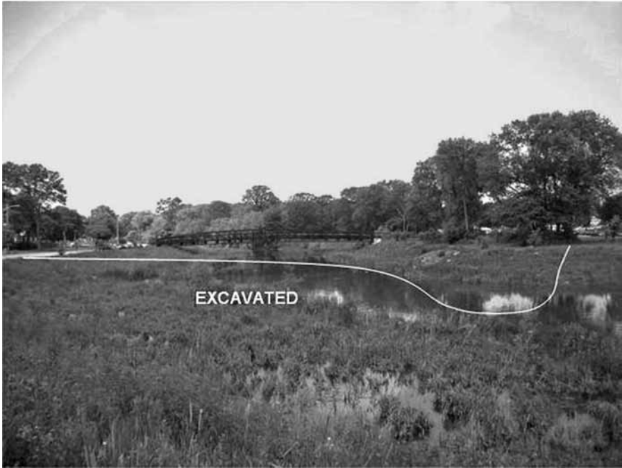
Figure 9.23 Lower portion of Lincoln Creek looking upstream. The white line shows approximately the original cross section. The right bank of the floodplain was excavated to provide flood storage with a riparian wetland. Photo V. Novotny.
