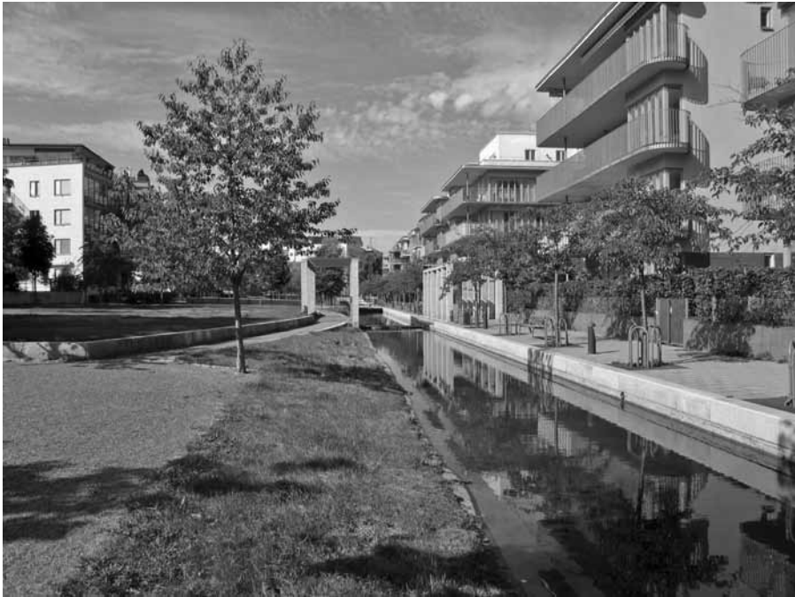
Figure 11.2 Residential area with a surface stormwater channel (Courtesy Malena Karlsson, GlashusEtt).
