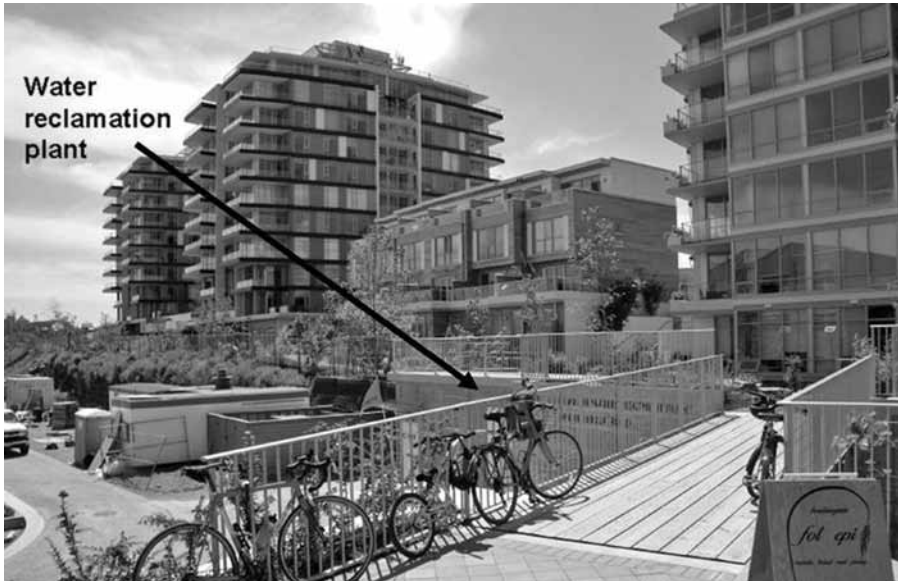
Figure 10.3 Docksde Green, Victoria, British Columbia, on-site tertiary wastewater treatment, which provides disinfected reclaimed water for use throughout the site, including toilet flushing, irrigation, and top-up water for the central waterway. (Courtesy W.P. Lucey, Aqua-Tex Scientific Consulting, Ltd.).
