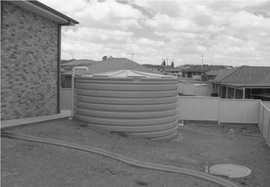
Figure 5.10 A 10,000-liter rainwater collection tank installed in Orange City, New South Wales, Australia. The city is located 270 km west of Sydney in a semi-arid area. Photo credit Orange County.
