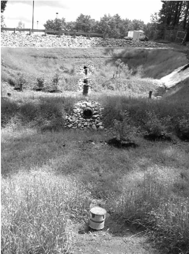
Figure 4.21 Experimental research gravel wetland treating runoff from a parking lot at the Stormwater Center on the campus of the University of New Hampshire. The compartmentalized arrangement works best for urban stormwater. Photo V. Novotny.
