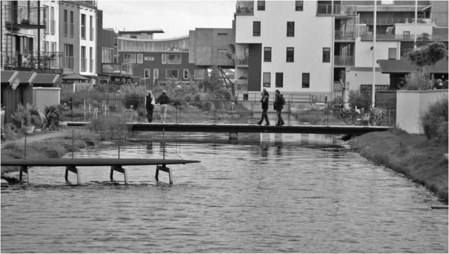
Figure 3.16 A courtyard canal in Bo01/Western Harbor, part of the surface drainage system and an important element for organizing and structuring the urban form of the project. Photo: Jack Ahern.
