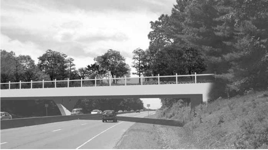
Figure 3.3 A proposal for a multifunctional wildlife and pedestrian crossing of a state highway at Walden Pond near Boston, Massachusetts. The highway overpass supports wildlife and pedestrian movement, with a major highway passing underneath—an example of “stacking functions” (Image: Jinglan Wang).
