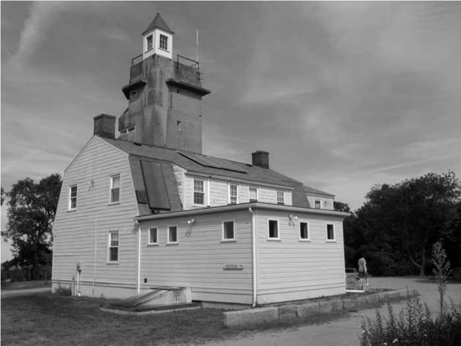
Figure 8.15 Roof solar panels (concentrated heat for hot water and photovoltaic for electricity) on the roof of a county park visitor center in Rockport, Massachusetts. Photo V. Novotny
