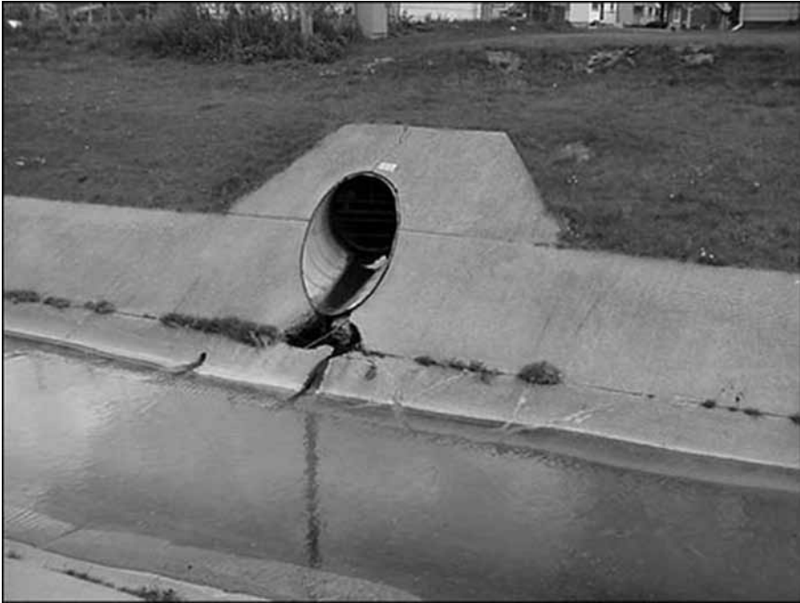
Figure 1.17 Lincoln Creek in Milwaukee, Wisconsin, was a concrete-lined channel receiving combined sewer overflows, before restoration in the 1990s. Photo V. Novotny.
