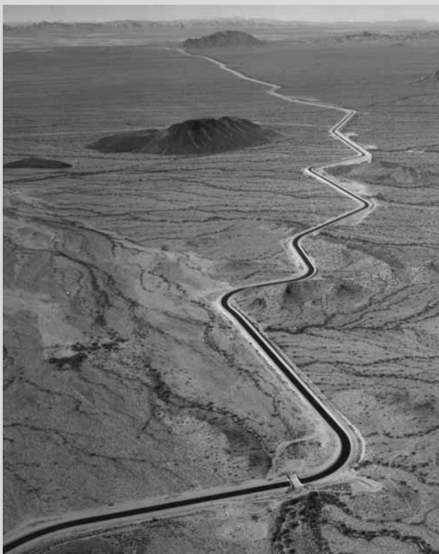
Figure 5.4 Central Arizona Project canal delivering water from the Colorado River to Arizona cities, farmers, industries, and Native American nations. The canal is 541 km long, and it is the largest water project in the U.S. (Credit U.S. Bureau of Reclamation).
