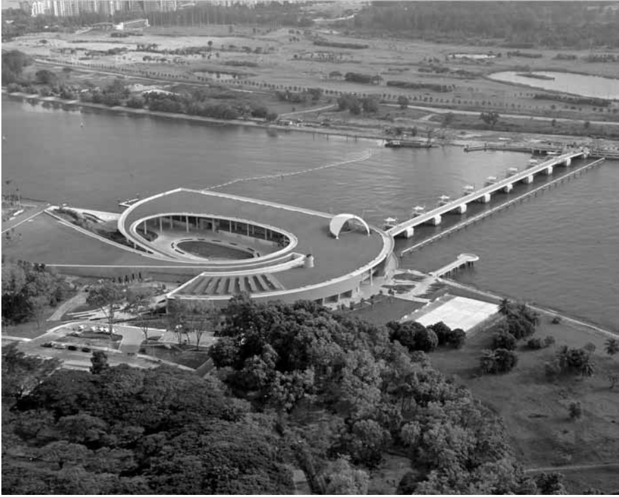
Figure 6.13 Marina Barrage and pumping station at the mouth of the Singapore River changed the tidal estuary into a freshwater body collecting treated urban runoff (to the left of the barrage). Water is pumped into upstream water supply reservoirs to augment the available fresh catchment water. The green roof of the pumping station is used as a vista and for picnicking (Photo courtesy CDM.).
