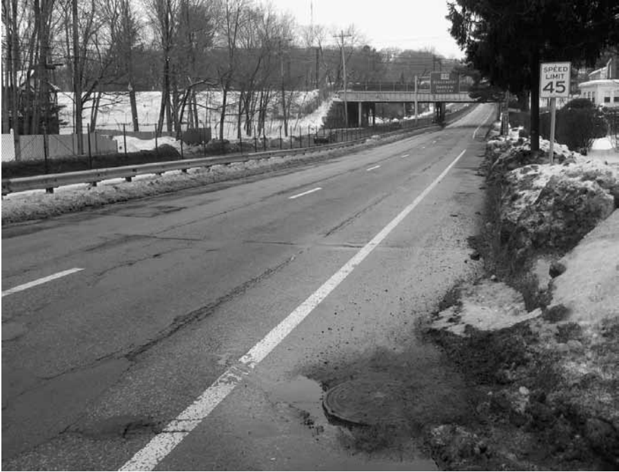
Figure 4.23 Highway 9 in Newton, Massachusetts. Heavy pollution of urban snow and snowmelt is exacerbated in storm sewered urban areas where no attenuation or removal of high concentrations of pollutants is provided (Photo V. Novotny).
