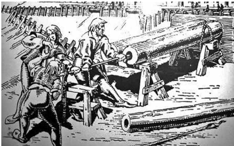
Figure 1.9 Making wood pipes for the medieval water supply systems (courtesy: Museum of Water Supply in Prague, Czech Republic).
