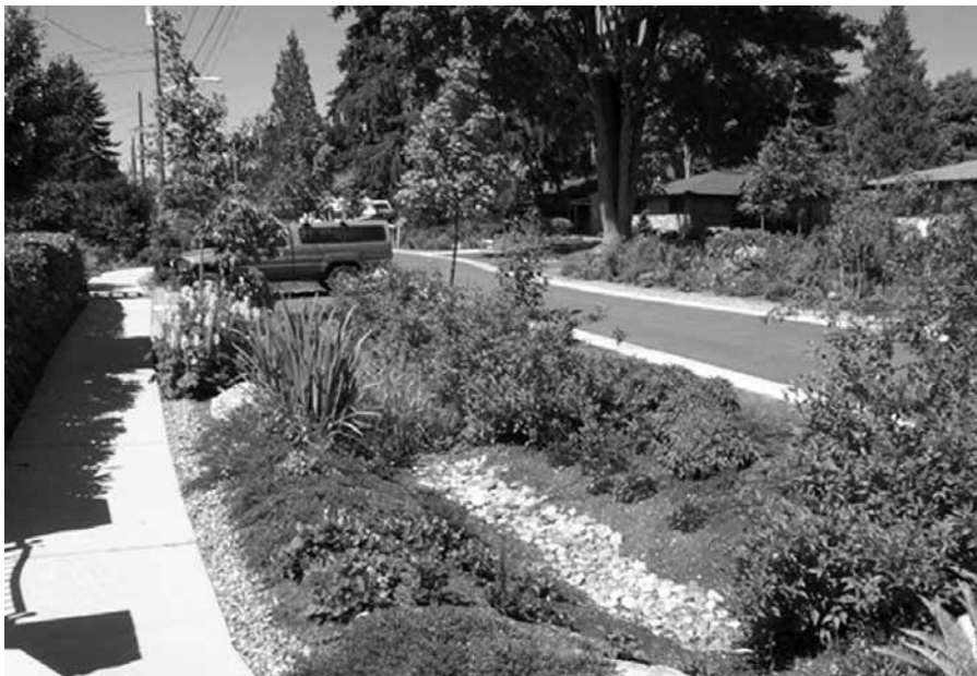
Figure 4.9 Type of swale found in a Seattle SEA neighborhood. The swale conveys, treats, and infiltrates runoff Courtesy Seattle Public Utilities.
