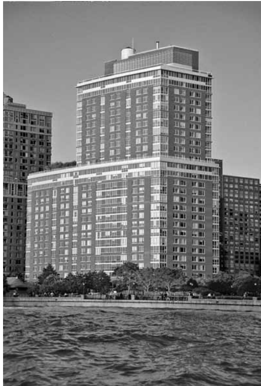
Figure 6.8 Solaire Apartments, Battery Park, in New York City. A LEED Platinum certified “green” building with nonpotable water reclamation and reuse.
