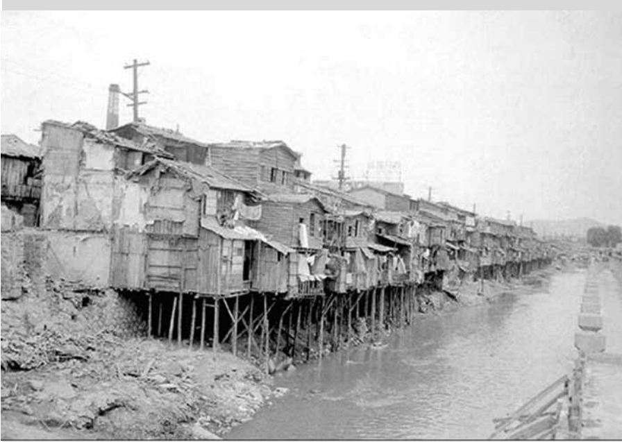
Figure 9.1 The Cheonggyecheon River in Seoul, Korea, in the 1950s. Refugees from the Korean War built squatter shanties on both sides of the river. The river did not have enough low flow to dilute raw sewage discharges. Source: Public files of the Seoul Metropolitan Government.
