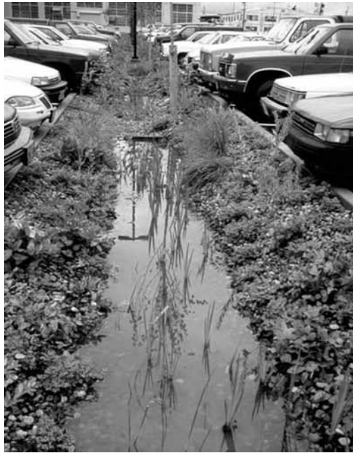
Figure 2.14 Landscaped swale providing infiltration and pollutant removal (photo from Marriott, 2007).
