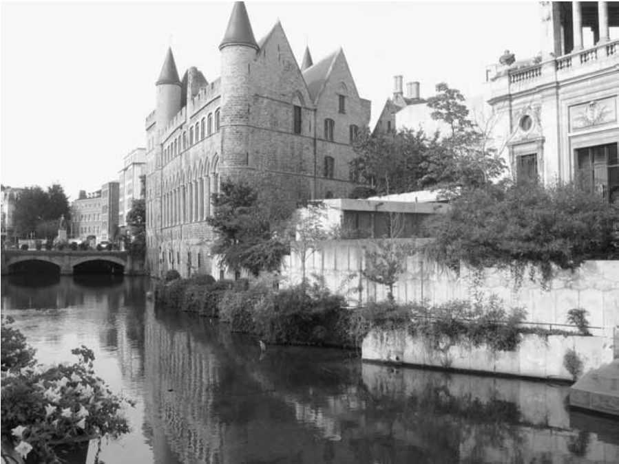
Figure 9.8 Daylighted (uncovered) portion of the canal in Ghent. The canal receives CSOs and has relatively poor habitat. Photo V. Novotny.
