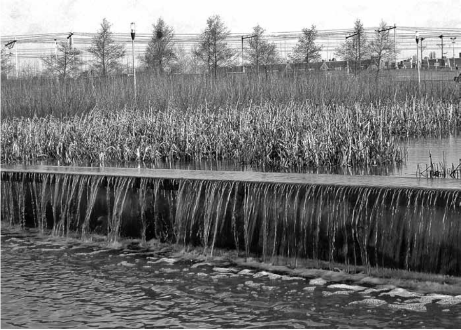
Figure 3.10 Stormwater biofilter and cascade, Westergasfabriek Park, Amsterdam. Here, green infrastructure goes beyond functionality; it creates a designed experience for park visitors that informs about sustainability, the role of plants, and the beauty of the simple process of circulating and cleaning stormwater (Koekebakker, 2003). Photo: Jack Ahern.
