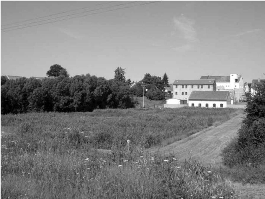
Figure 7.4 Constructed wetland with subsurface horizontal flow consisting of two parallel series, each with two compartments, built in Rakovník, Czech Republic. The load coming from a combined sewer has a population equivalent of 800, and the area of the wetland is 3080 m 2 . Courtesy Jan Vymazal.
