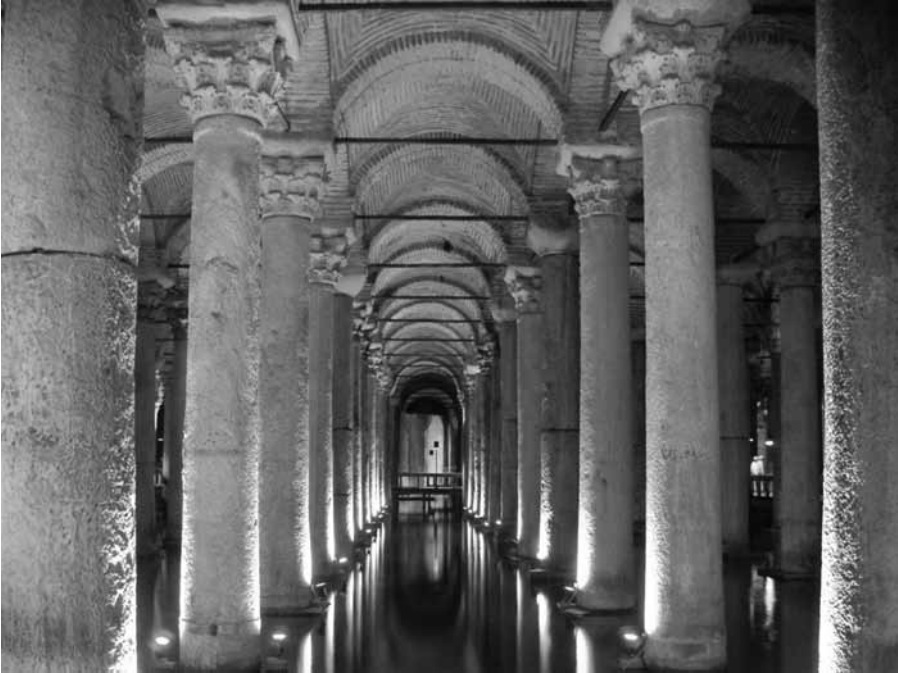
Figure 1.7 This underground Basilica cistern, capable of storing 80,000 \text{ m}^3 ( 21.1 \text{ mg} ) of water, was built at the beginning of the seventh century in Constantinople, the capital of the Byzantine Empire (present-day Istanbul in Turkey) (photo V. Novotny).
