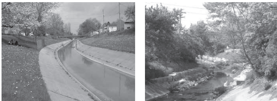
Figure 2.12 Lincoln Creek in Milwaukee, Wisconsin. Left, channelized before restoration; right, after restoration. Photos by V. Novotny.
