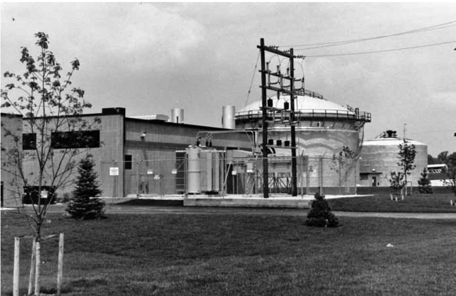
Figure 7.10 A power plant producing electricity from biogas (methane) collected from the Omega Hill landfill operated by Waste Management in Germantown (Wisconsin) in 1990s. Photo V. Novotny.
