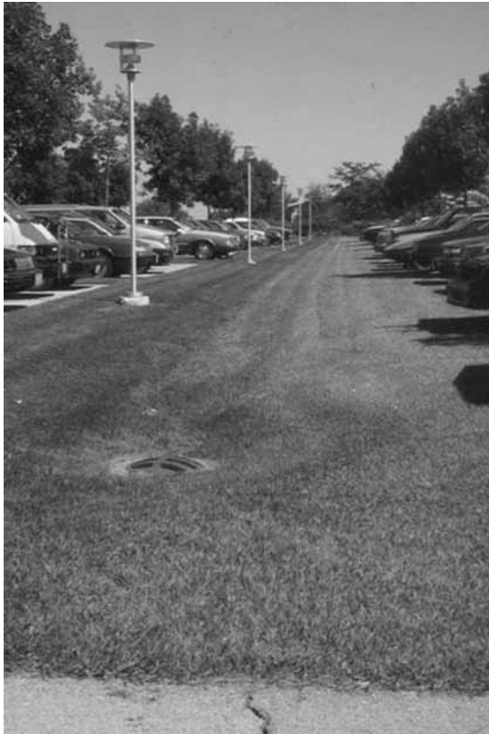
Figure 4.11 Example of a simple filter strip along a parking lot, filtering runoff before entering storm drain.
