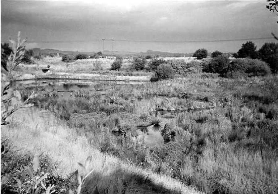
Figure 4.22 Stormwater wetland in Scotland treating runoff from an industrial site (photo V. Novotny).
