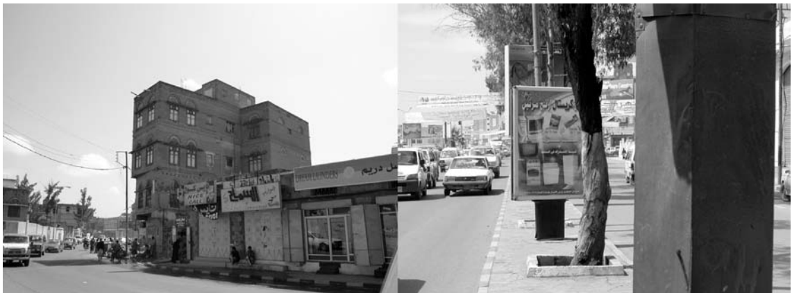
Figure 5.11. Two views of modern roads in Sana'a. Urban patterns are very varied and minimum consideration is given to human spaces.
