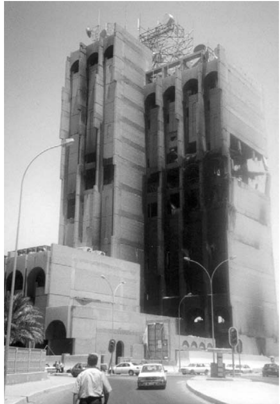
Figure 4.9. Baghdad Central Post Office in April 2003.
