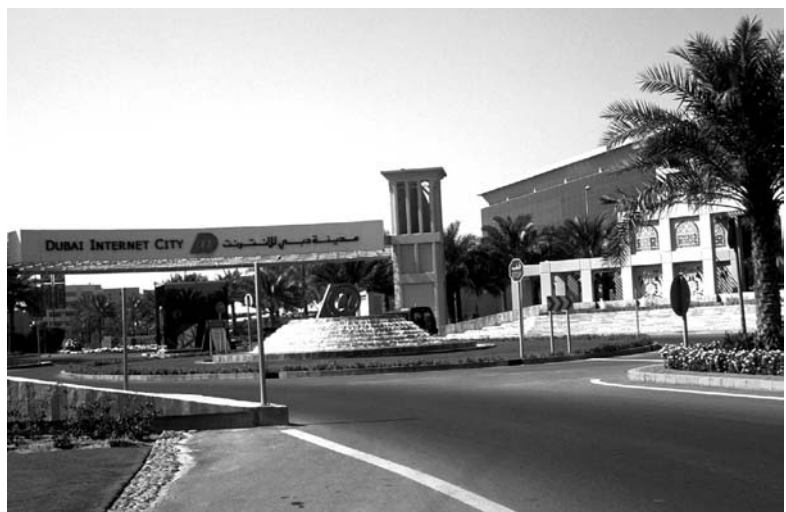
Figure 8.5. Entrance to Dubai Internet City.
