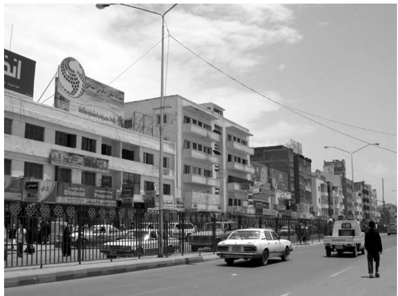
Figure 5.7. The first modern buildings to emerge in Sana'a, which were designed and constructed by Egyptian expertise in the late 1960s and early 1970s.
