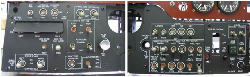
Fig. 55.2 Two control panel module of the FSTD
