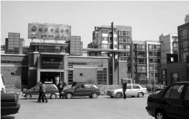
Figure 2.20. The community club of Boyaxiyuan, a middle-class residential district with 1,187 apartment units in Beijing, designed by Lu Duanmin et al. , and completed in 2004 (photo taken in 2005).
