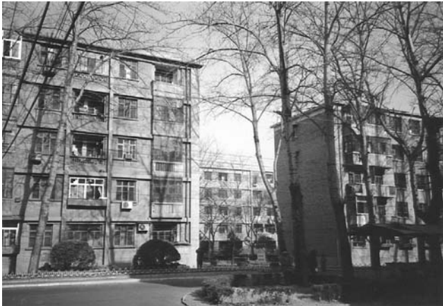
Figure 3.18. Five-storey apartment buildings in Beijing (photo taken in 1999)
