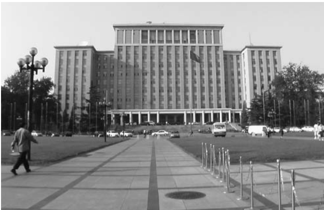
Figure 3.12. Main Building, Tsinghua University, Beijing, competed in 1968 (photo taken in 2005). The design of the building was influenced by the main building of the Moscow State University. Due to limited construction funds, the central Soviet-style tiered tower in earlier plans was replaced with a plain terraced roof.
