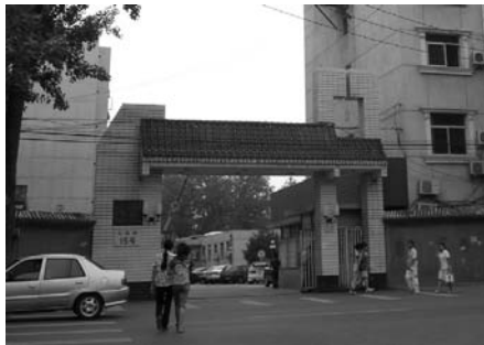
Figure 3.1. Gate with the janitor's room on one side, Beijing (photo taken in 2005).
