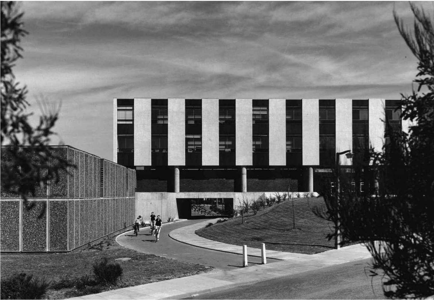
Wine makers Gilbeys expanded into gin and whiskey production, with new offices and distillery in Harlow, shown here in 1964. Copyright: Museum of Harlow.
