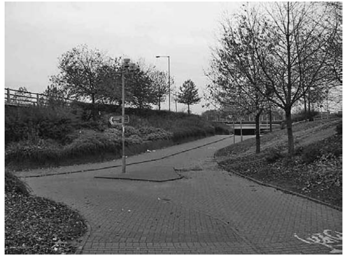
Segregated and grade-separated pedestrian and cycle routes were intended to be safer, but lack 'natural surveillance' and have proved expensive to maintain.
