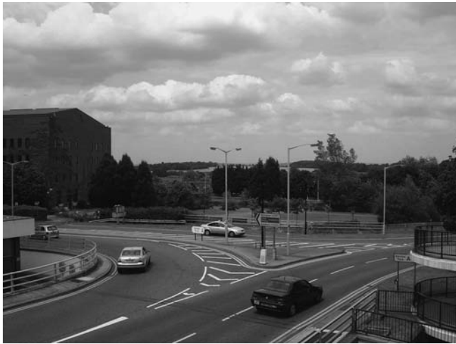
Highway-scale roads next to Bracknell town centre create severance.
