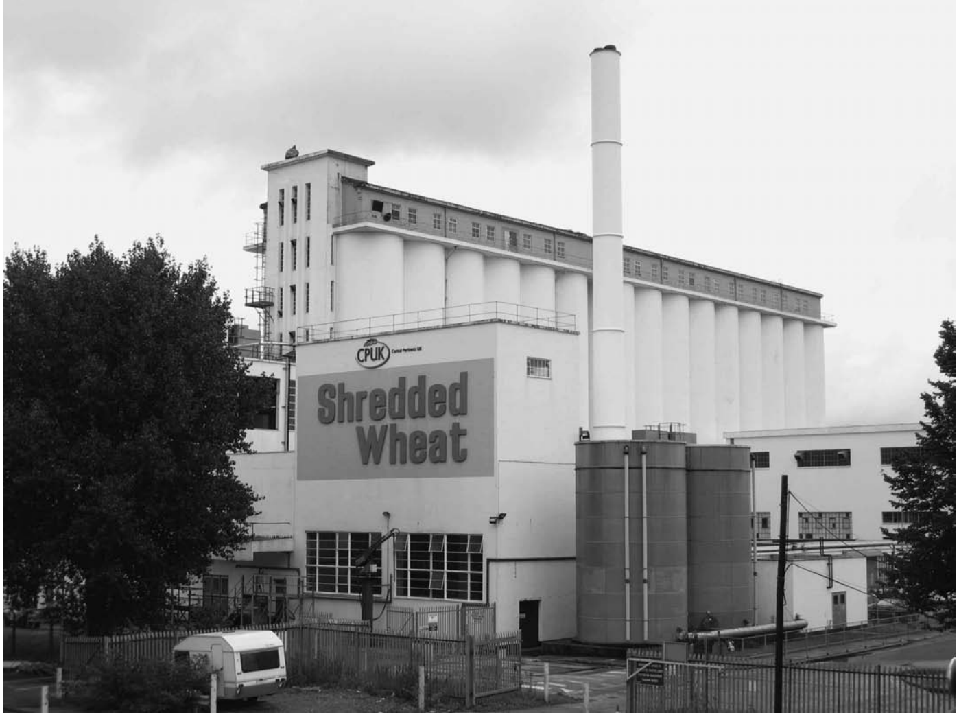
Welwyn's industrial facilities included Nabisco's Shredded Wheat Factory.
