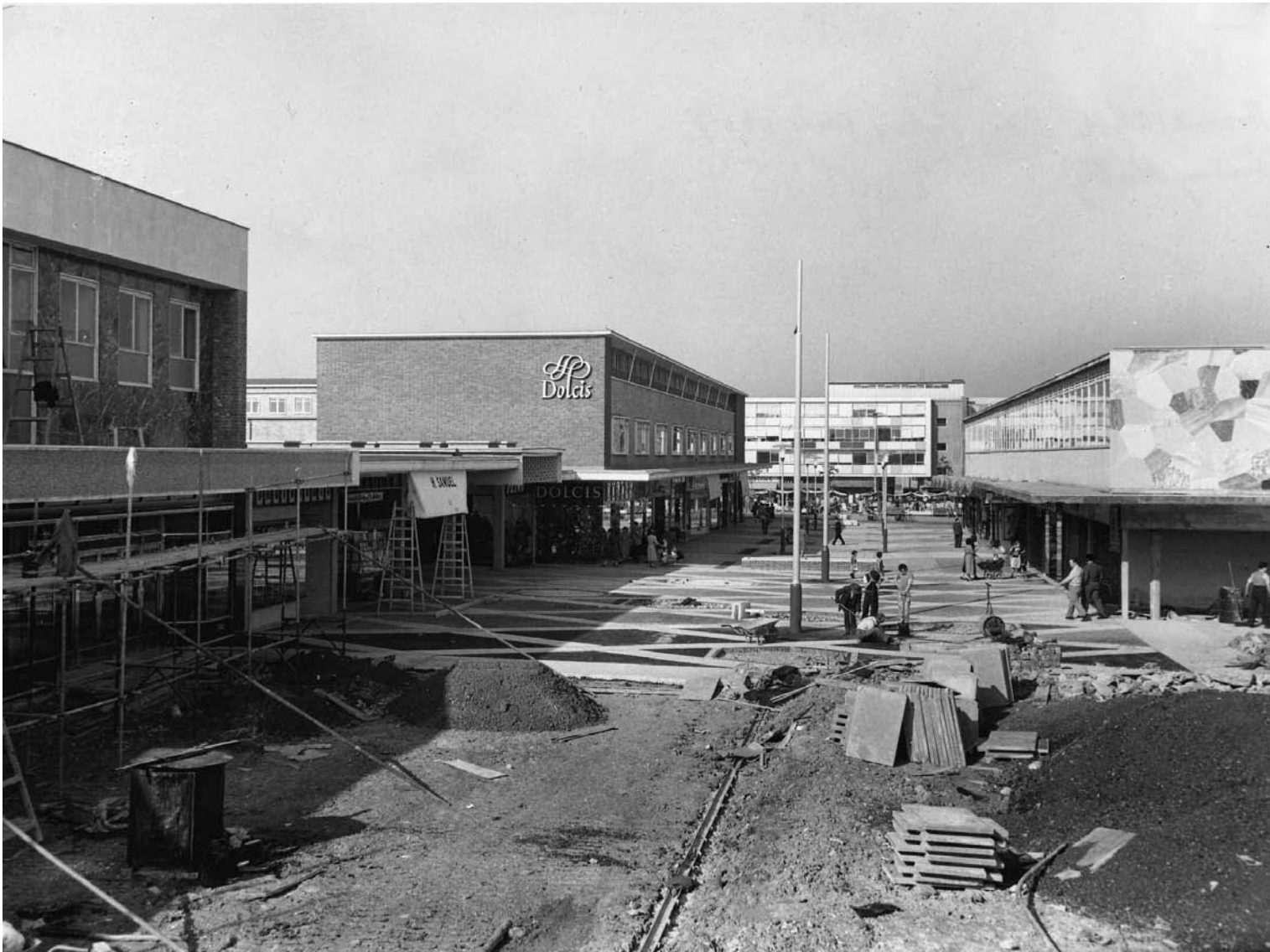
Broad Walk, The High, Harlow town centre, under construction in 1956. Source: Museum of Harlow.
