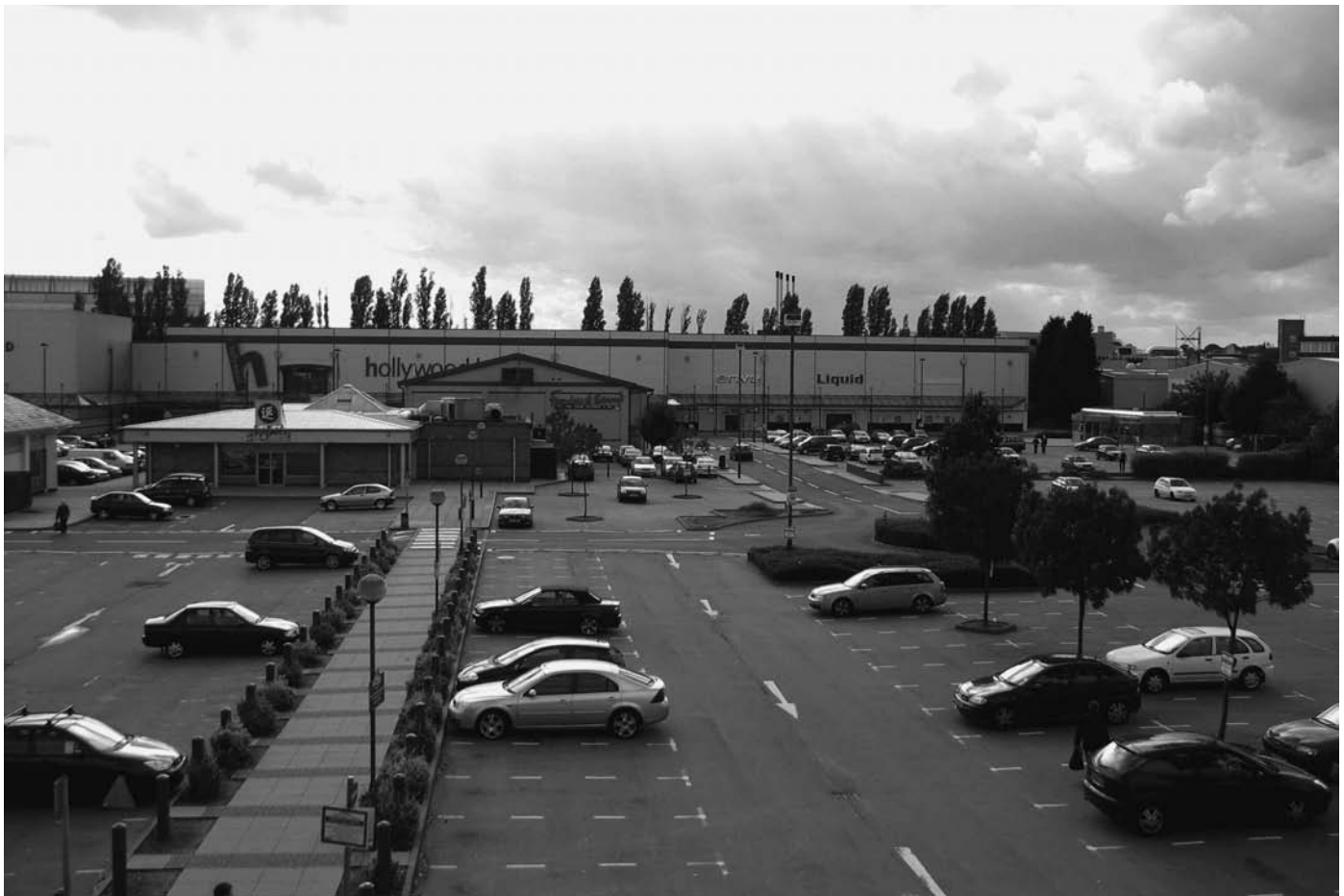
The Stevenage Leisure Centre on part of the former industrial estate immediately to the west of the train station and the town centre, represents a major new centre of activity for the town. As with Crawley (described on page 86) this new development represents growth but also draws economic life away from the former places of activity in the town.
