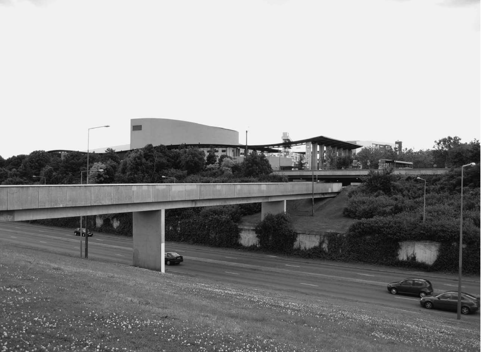
Central Milton Keynes and its high capacity road network
