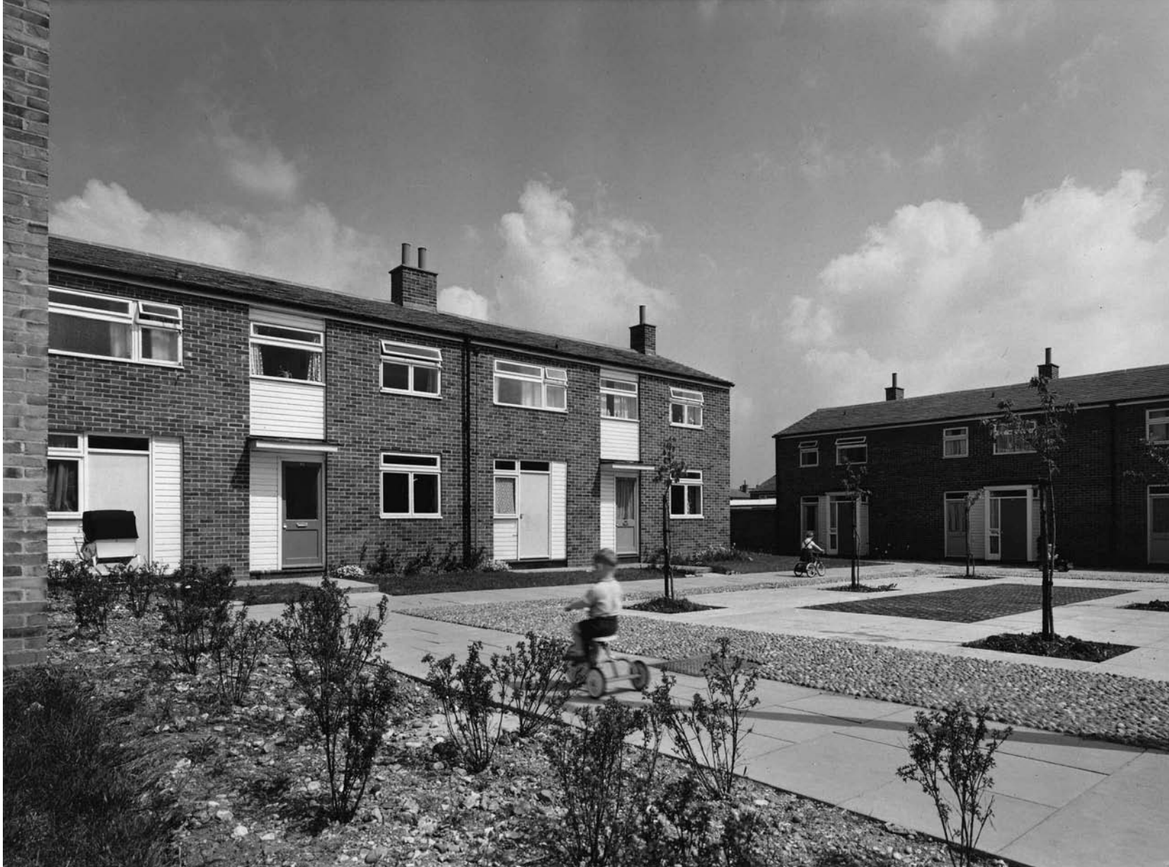
The Altham Grove estate in Harlow, built to the Radburn principles of the front of the house facing a car-free area, and cars parked at the rear of the house.
