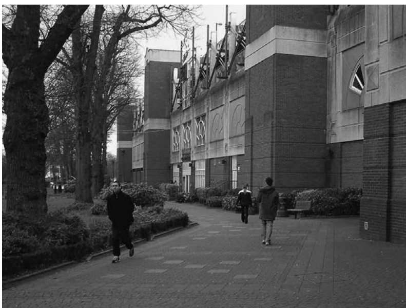
Opening in 1992, The County Mall is a large indoor shopping centre with multi-storey car park, located a short distance to the south of Crawley New Town centre, and easily accessed by car.
