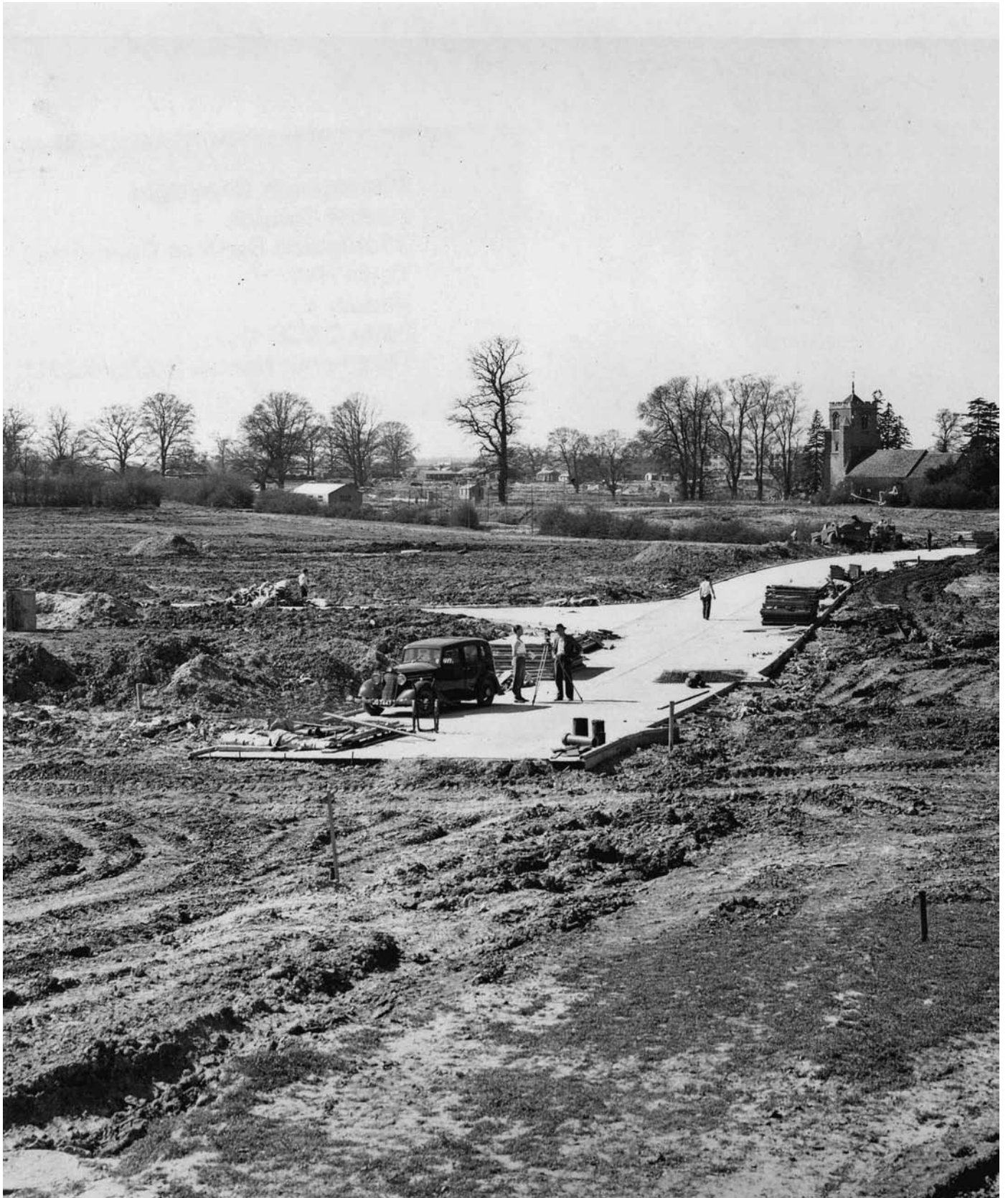
Construction begins in Mark Hall North, Harlow, 1951.
