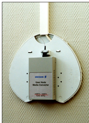
Fig. 11-37–11-39 The wall-outlet with opto-electric switch
