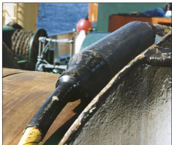
Fig. 11-30 The submarine joint closure SJC 240 ready to go down.
