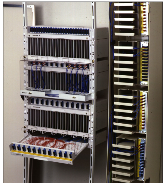
Fig. 11-49 Pre-terminated ODF.
