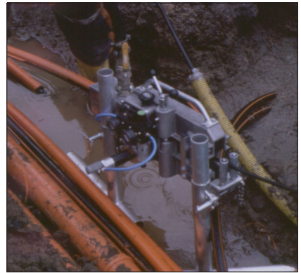
Fig 11-17 Floating with water, equipment set-up.
