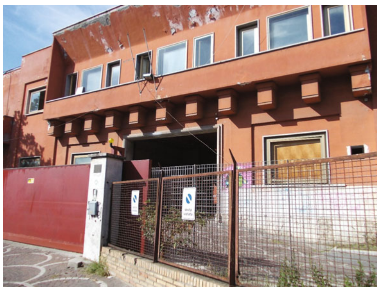
Fig. 13.7 Main entrance Cartiera (Figure by Gaja Maestri)
