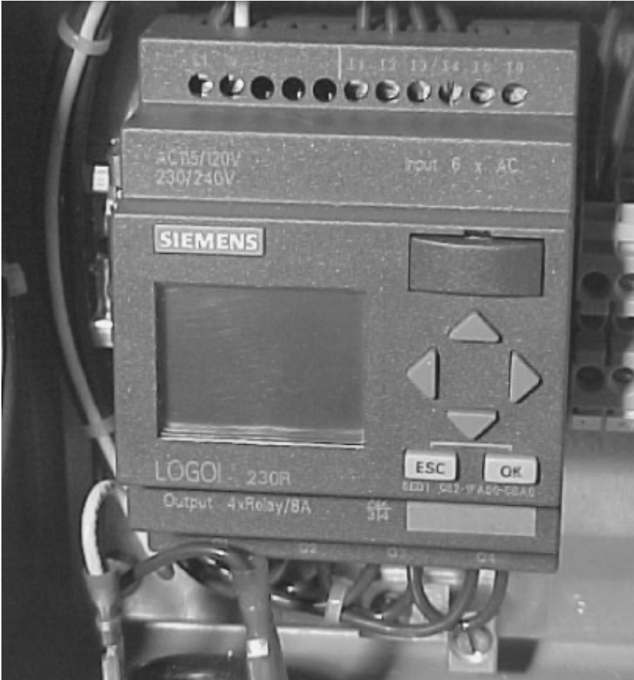
Photo 3.2 Programmable logic controller
