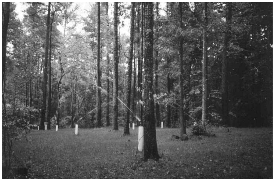
Photo 5.6b Spray irrigation system installed in wooded area, back yard of a house, used for dispersal of effluent from an advanced onsite wastewater treatment technology that serves a single family home.
