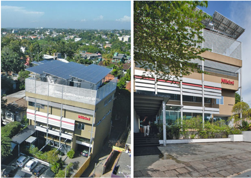
Fig. 4.3 Left: The aerial view of Nikini building with the roof PV panels and shading devices. Right: Front elevation of Nikini building (Source: The Authors)
