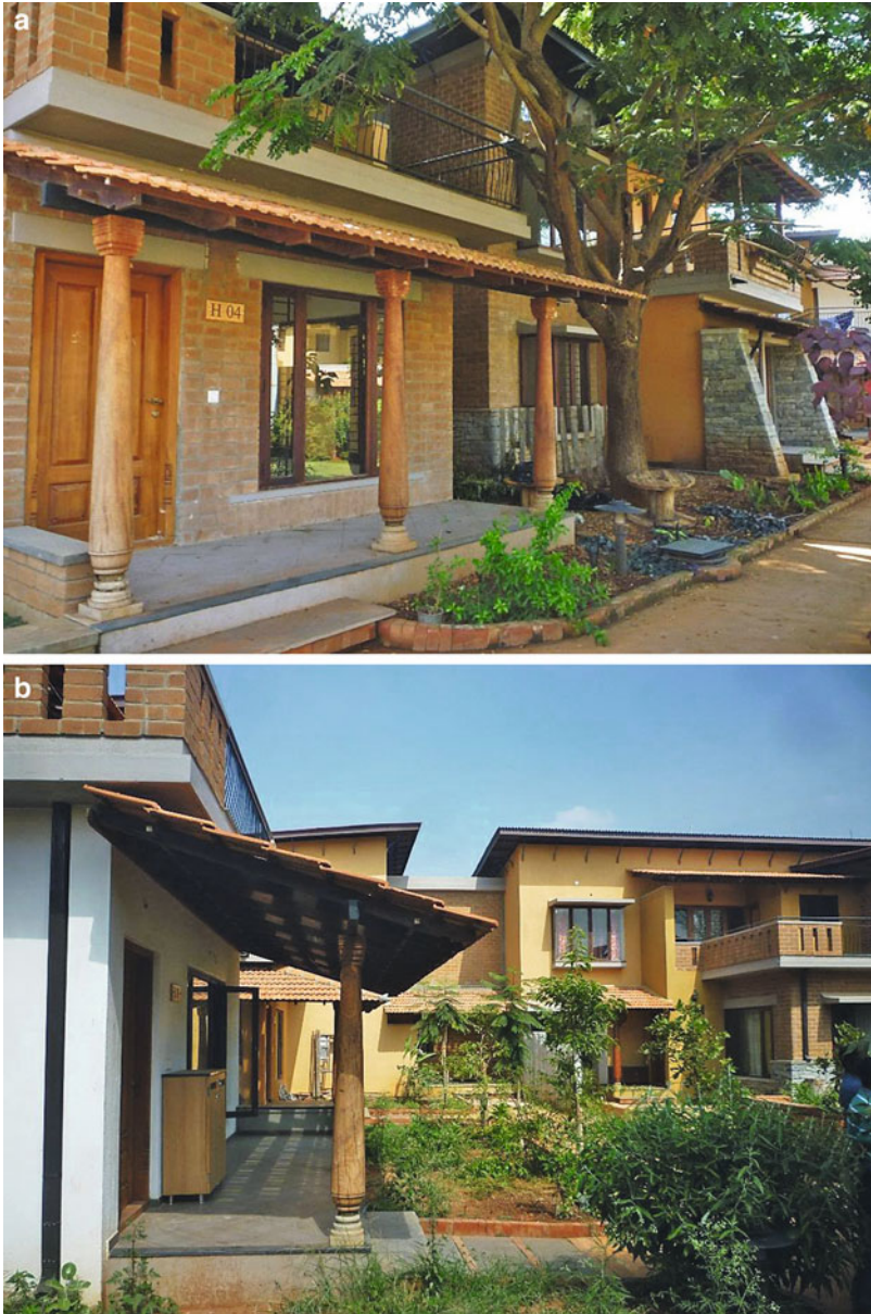
Fig. 7.4 The front view ( top ) and side view ( bottom ) of clustered houses with mud blocks and shading from verandas and fast-growing trees (Source: The Authors)
