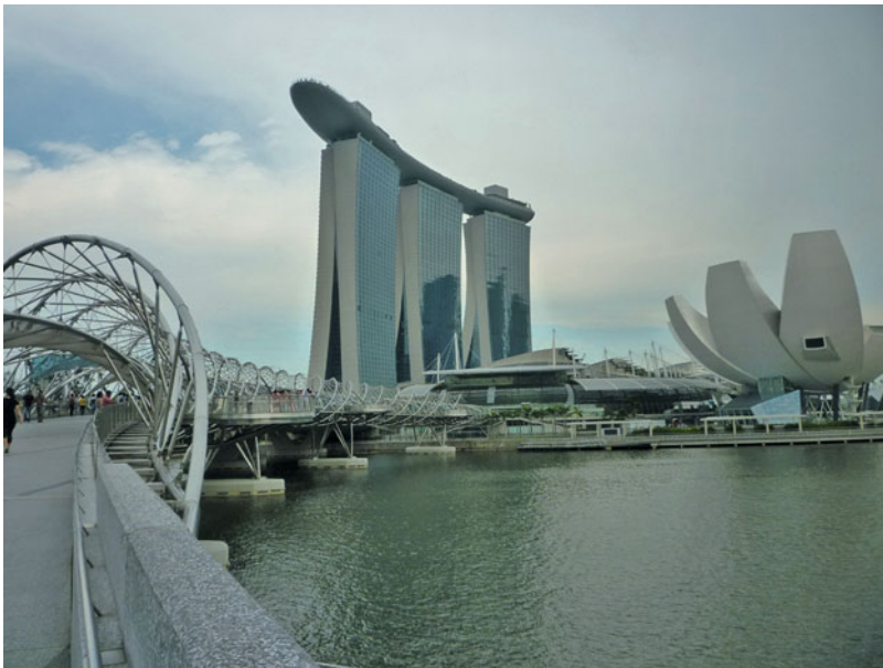
Fig. 12.5 The Marina Bay project in Singapore is one of the largest district cooling projects in the world. It illustrates integration of sustainable urban energy systems into large urban design and architectural projects. Marina Sands Bay, Singapore (Source: Ali Cheshmehzangi).
