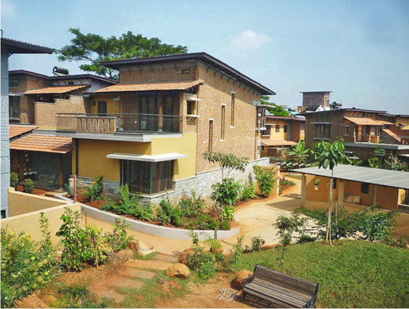
Fig. 7.2 The clustered layout of housing communities of Malhar eco-village (Source: The Authors)
