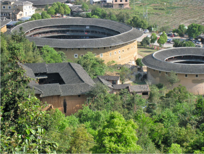
Fig. 12.2 China's remarkable Tulou houses represent some of the best examples of vernacular architecture. These structures represent several dimensions of sustainability: social (by creating strong local communities), environmental (by using local materials and enhancing passive cooling), and economic (by durable construction methods with low costs and maintenance). Fujian Province, China (Source: Chris Butters).
