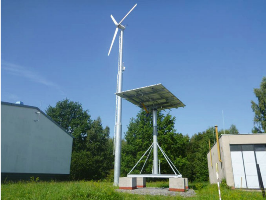
Fig. 4.19 A photo of the WPP together with an adjustable swivel unit of the PPP
