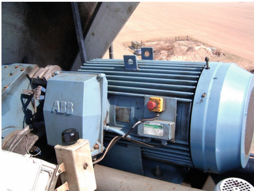
Fig. 2.17 A generator placed in the nacelle of the wind motor
