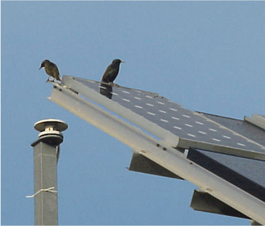
Fig. 3.23 Pollution of the surface of photovoltaic panels [15]
