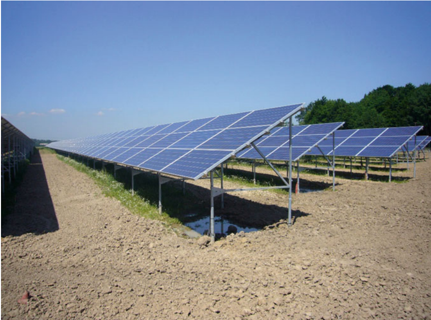
Fig. 3.24 Properly designed spacing between individual rows of panels
