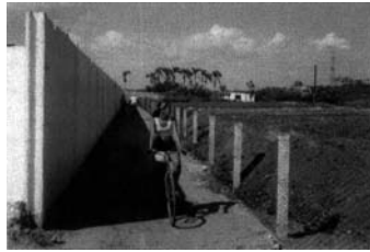
A cycle path shaded by a wall runs alongside the Cuatro Caminos organoponico in Cienfuegos.
