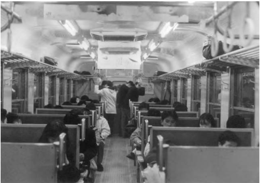
Figure 9.2a A more comfortable carriage built by JNR for a local commuter train
