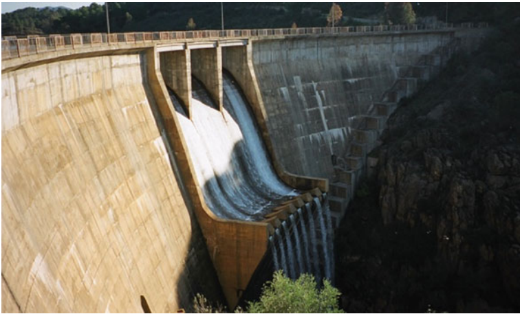
Fig. 6.35 Industrial water supply reservoir at Almagrera, Spain
