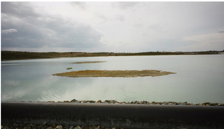
Fig. 6.19 Exposed tailings surface during sub-aqueous disposal
