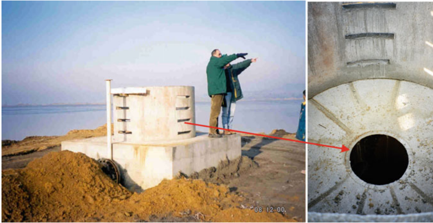
Fig. 6.51 Central decant tower at Baia Mare, Romania
