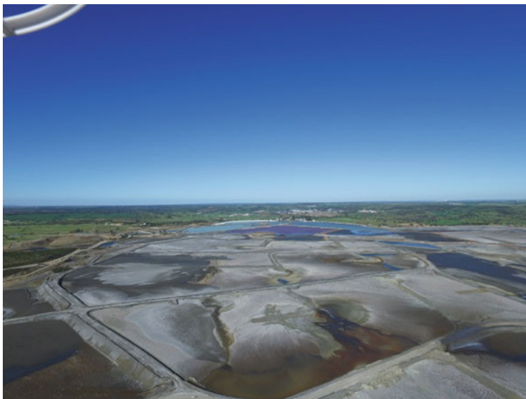
Fig. 6.40 Paddock system for tailings disposal on IRCL, Portugal
