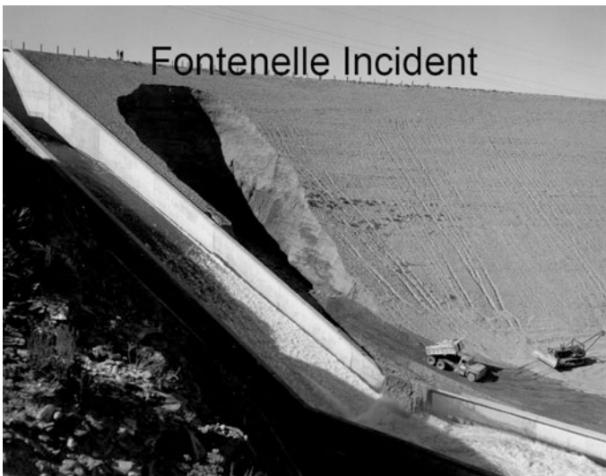
Fig. 5.11 Piping in dam face (Snorteland 2013)
