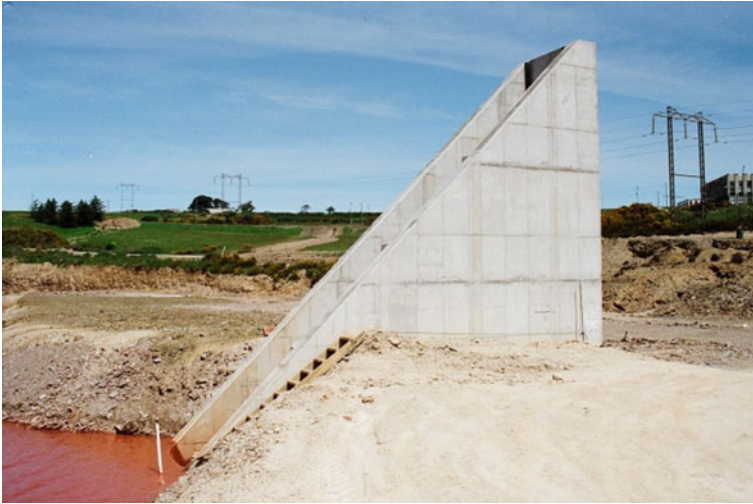
Fig. 6.49 Emergency spillway at CVTD, UK
