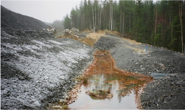
Fig. 7.12 Toe inundation preventing detailed inspection
