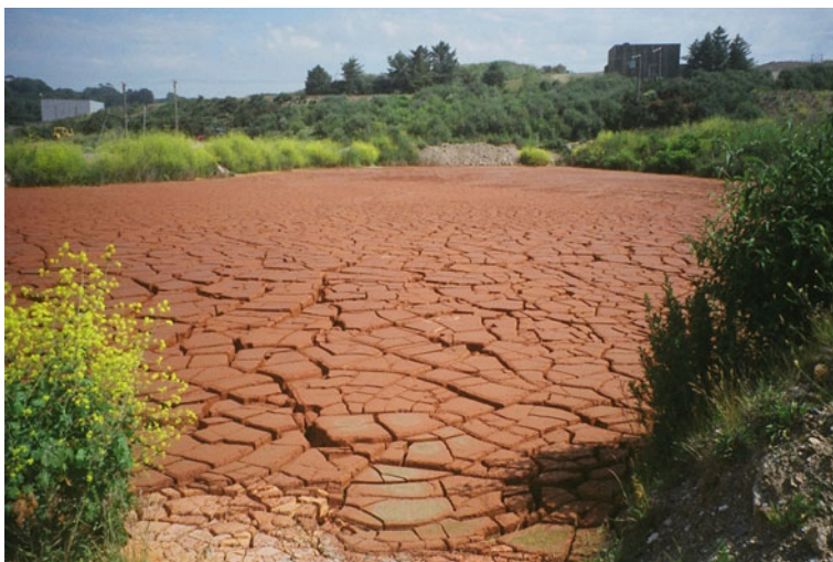
Fig. 6.39 Desiccating paddock minewater sludge on CVTD, UK
