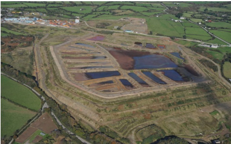
Fig. 6.37 Paddock system for storage of minewater treatment residues at CVTD, UK (Photograph courtesy of Wheal Jane Ltd)
