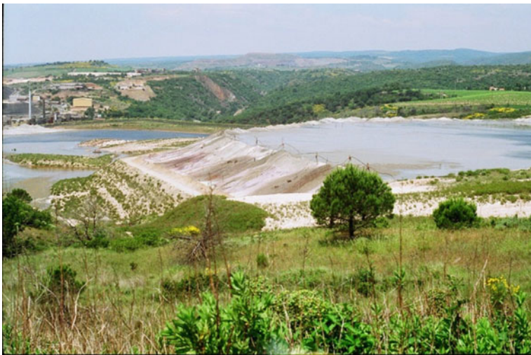
Fig. 6.28 Upstream construction using hydrocyclones, France
