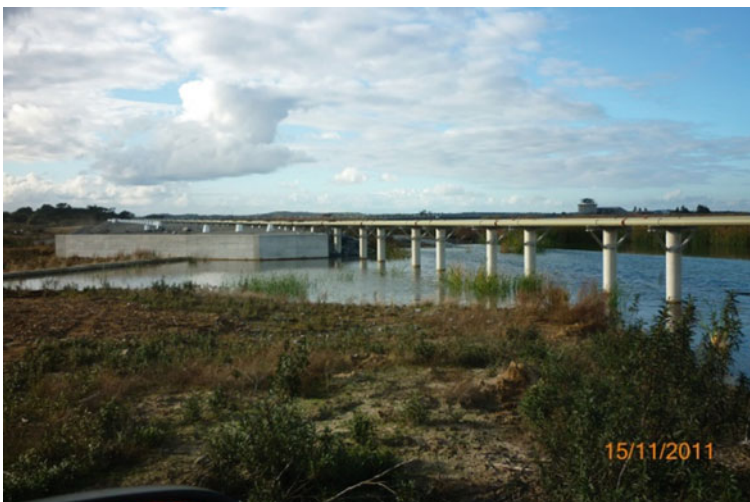
Fig. 6.48 Emergency spillway at IRCL, Portugal
