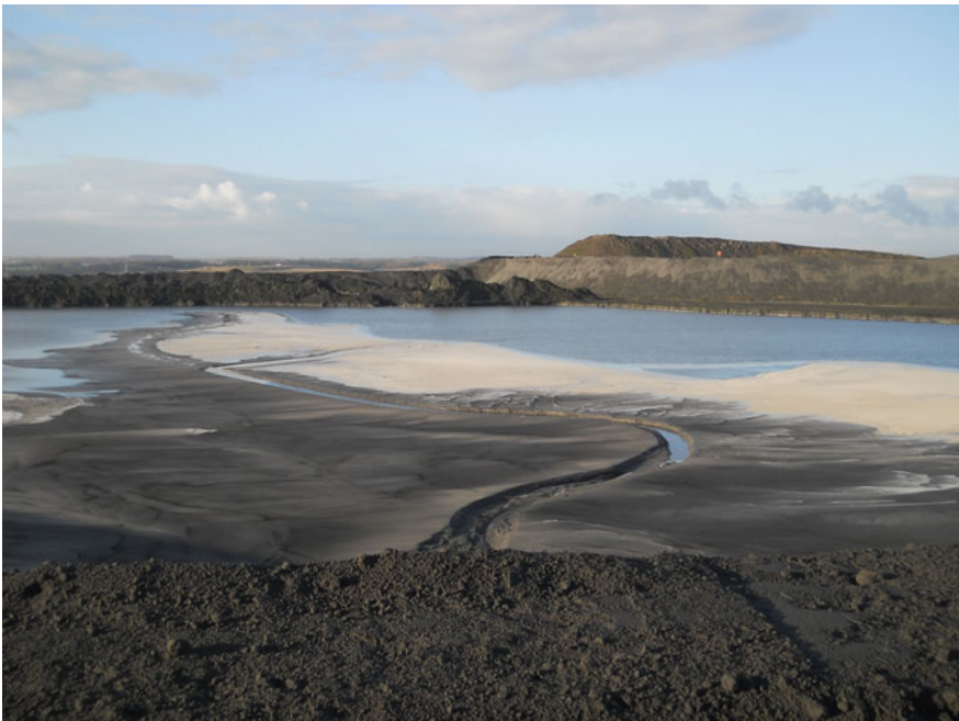
Fig. 8.2 Beach development in a fly-ash depository
