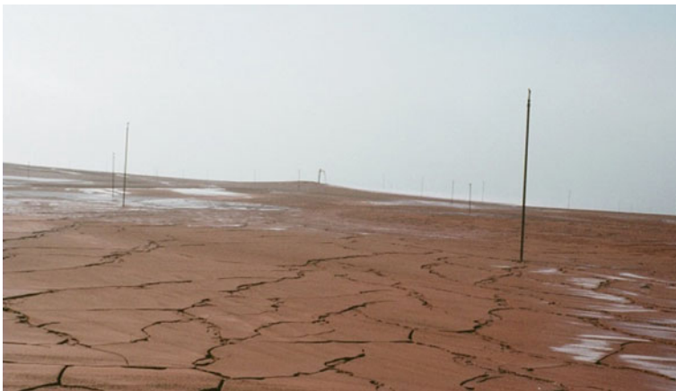
Fig. 6.32 Thickened deposition, Aughinish MWF, Ireland
