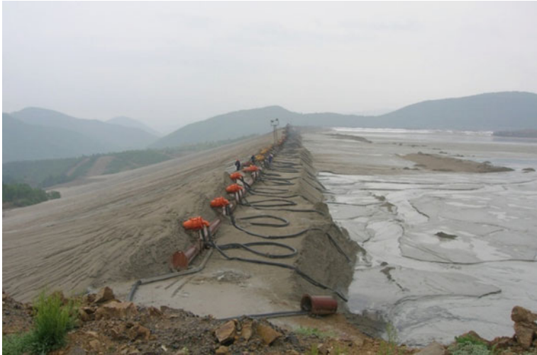
Fig. 6.27 Downstream construction using hydrocyclones, Bulgaria
