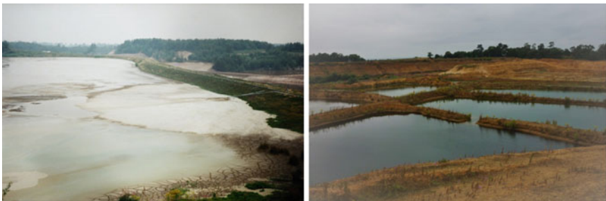
Fig. 6.4 Examples of in-pit hydraulic fill confining embankments
