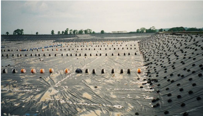
Fig. 6.6 Pre-deposition lining system at Galmoy MWF, Ireland
