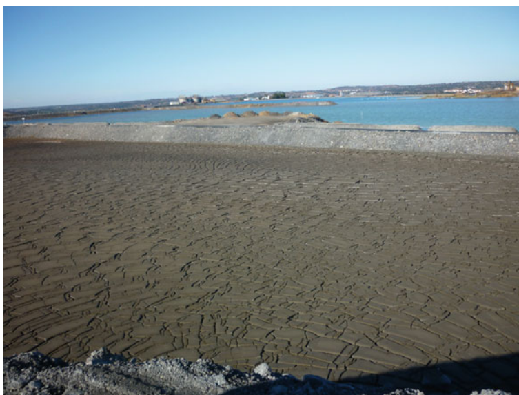
Fig. 6.41 Tailings disposal into paddock on IRCL, Portugal
