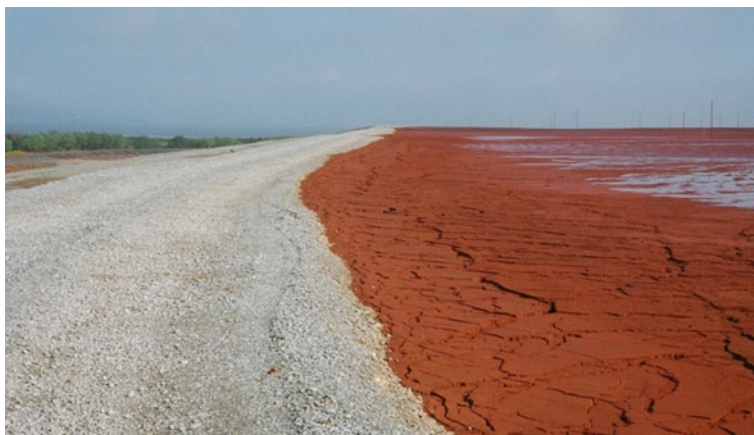
Fig. 6.33 Deposition against rockfill toe, Aughinish MWF, Ireland
