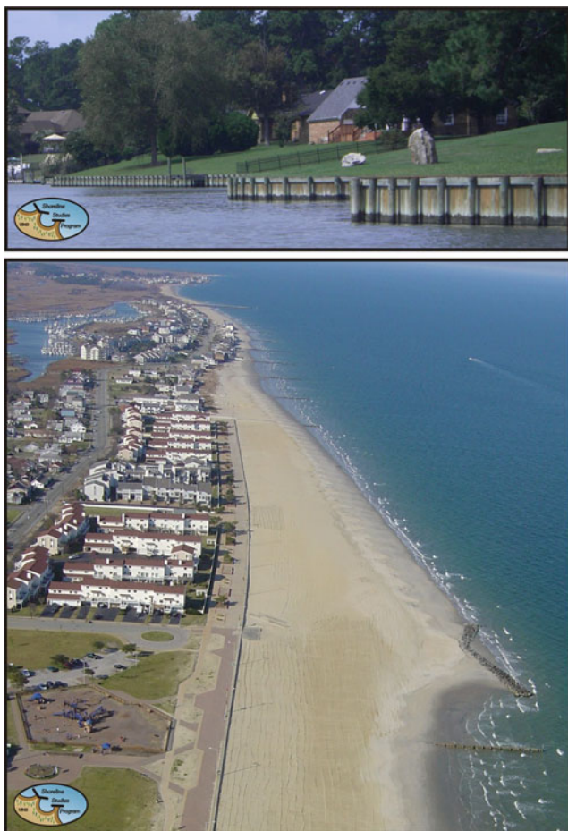
Estuarine Beaches, Figure 3 Top: Bulkheads in low-energy estuaries occupy the intertidal zone instead of beach or marsh habitat. Often, no buffer exists. Bottom: breakwater and beach fill create a wide, protective recreational beach.
