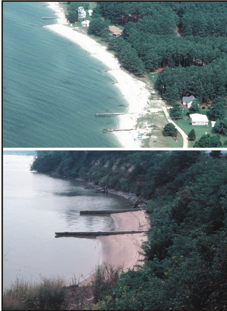
Shore Protection, Figure 4 Examples of groin fields in Chesapeake Bay, USA, that have top : a sufficient sand supply to create a protective beach and backshore and bottom : an insufficient supply of sand such that the groins act as littoral barriers and prevents sand from reaching the downdrift shoreline (From Hardaway and Byrne, 1999).
