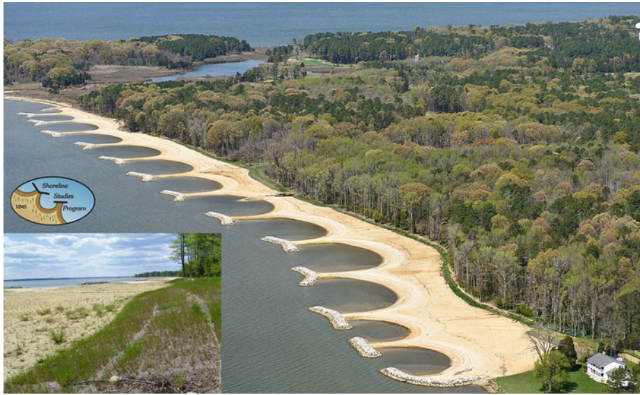
Headland Breakwaters, Figure 1 An aerial photo showing a headland breakwater project on the Potomac River within the Chesapeake Bay estuarine system soon after installation. Inset: A ground photo showing the extensive vegetation planting along the backshore.
