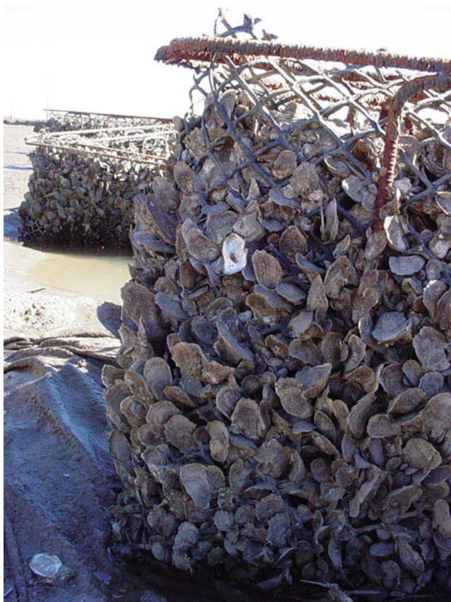
Bivalve Molluscs, Figure 10 Development of ReefBLK living shoreline reefs constructed of rebar and filled with shell in Texas, USA. Natural recruitment and growth after roughly one year (Source: Jeff DeQuattro, TNC, Mobile, AL, USA). See http://www.reefblk.com/ for more information.
