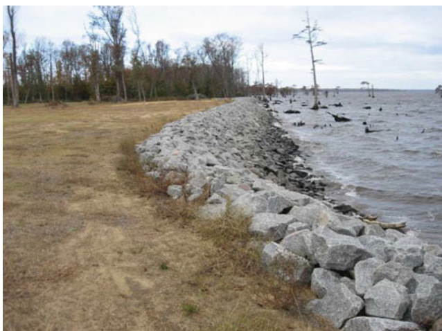
Coastal Erosion Control, Figure 11 Rip-rap revetments (Trowell, 2012).
