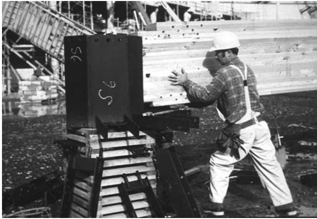
FIGURE 10.3 Large composite beam made from laminated lumber.
