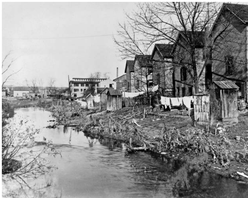
Figure 2.163: Bronx River Parkway, The Bronx, New York, and Westchester County, New York. Gilmore Clarke, Landscape Architect and Civil Engineer; Arthur Hayden, Designing Engineer; and Hermann Merkel, Forester; 1907–1925. A 1912 photograph documenting the conditions along the Bronx River before construction of the parkway. This “before” view from White Plains, New York, shows privies draining into the river. The “after” view in 1915 is shown in Figure 2.164. Library of Congress, Prints & Photographs Division, Historic American Buildings Survey/Historic American Engineering Record/Historic American Landscapes Survey Collection, HAER NY-327-80
