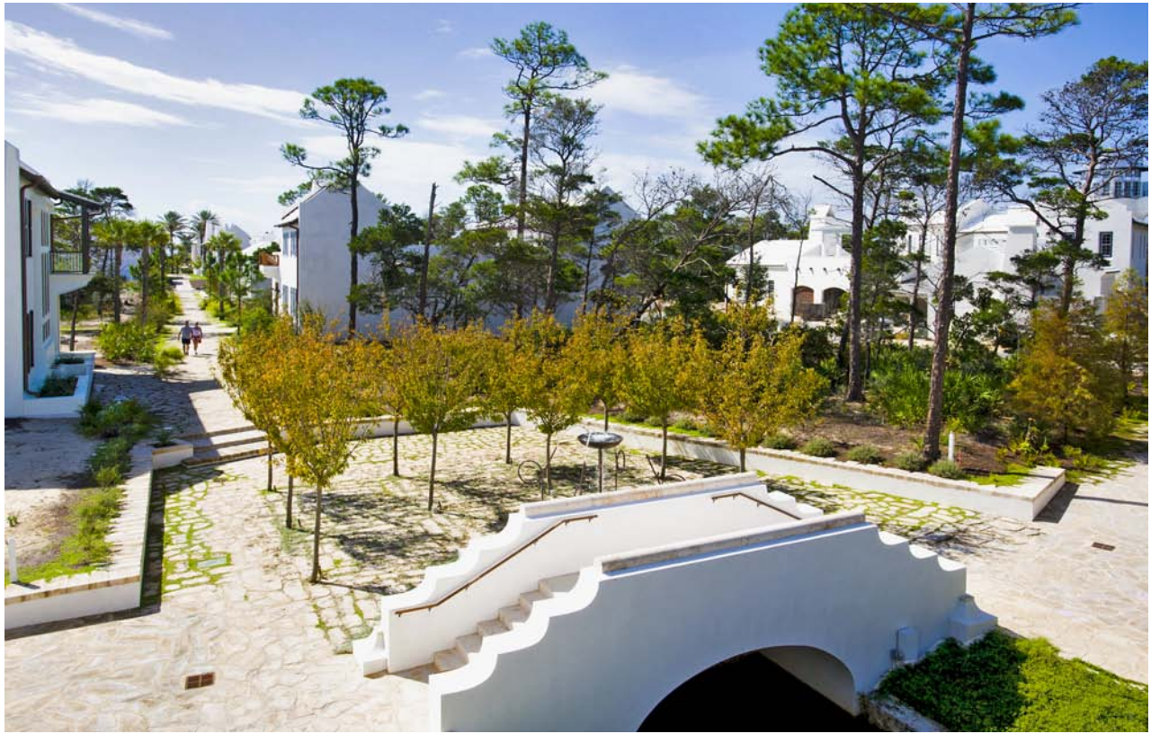
Figure 5.81: Sea Garden Walk, Alys Beach, Florida. Duany Plater-Zyberk & Company, 2003. At its northern end, the Walk opens up into less tightly wound space. (Construction photo.) Image courtesy of Kurt Lischka
