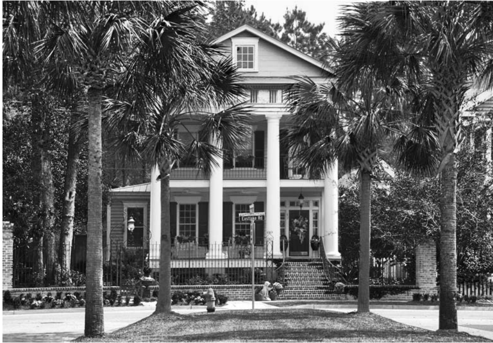
Figure 5.65: Boathouse Close, l’On, Mount Pleasant, South Carolina. Duany Plater-Zyberk & Company and Dover, Kohl & Partners, 1995. A Neoclassical house (B. J. Barnes, 2001) on Eastlake Road concludes the space.
