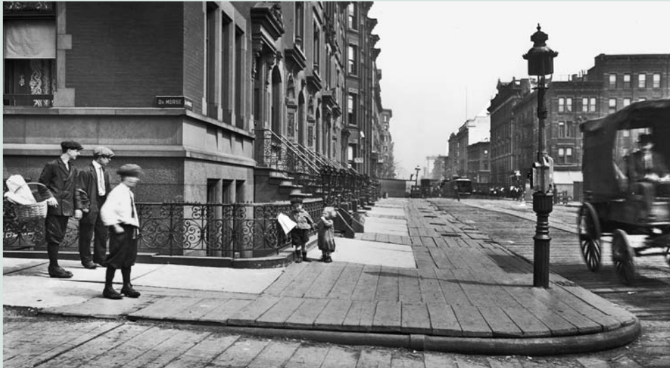
Figure 6.3: Lexington Avenue, New York, New York. Before: The northwest corner of Lexington Avenue and 89th Street in 1913. Photographed during the construction of the East Side IRT subway line, which explains why parts of the sidewalk have wooden planks rather than concrete. Image courtesy of the New York Transit Museum
