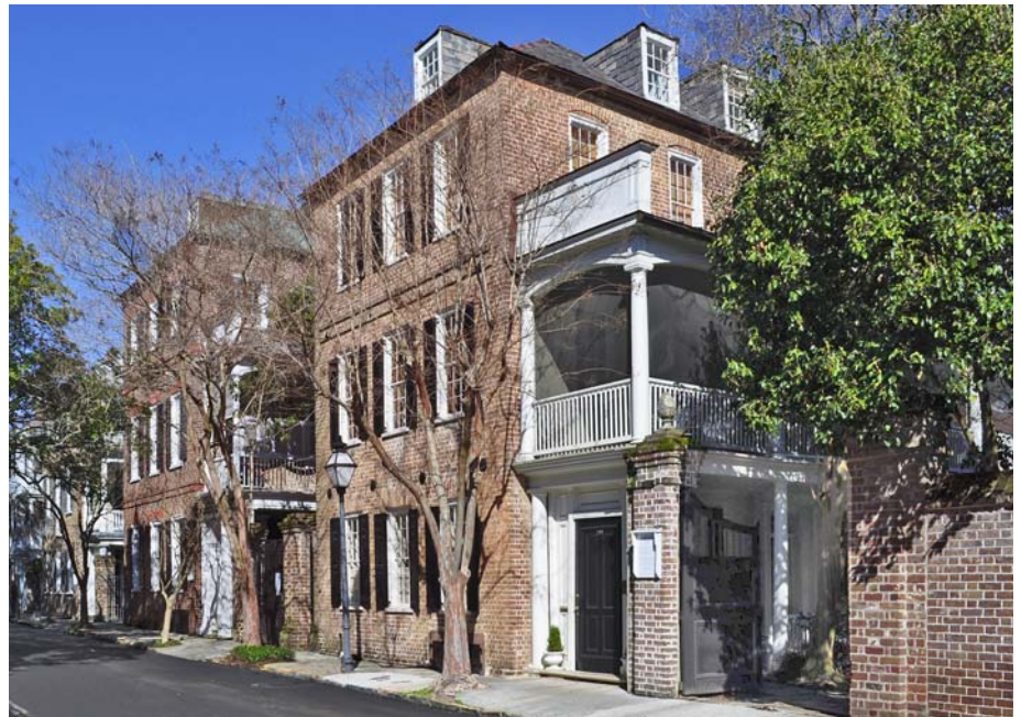
Figure 3.4: 90-94 Church Street, Charleston, South Carolina. Two Single Houses from the 1760s flanking an 1830s replacement show the continuity over time in Charleston’s homegrown building type. © 2013 Max L. Hill, III
