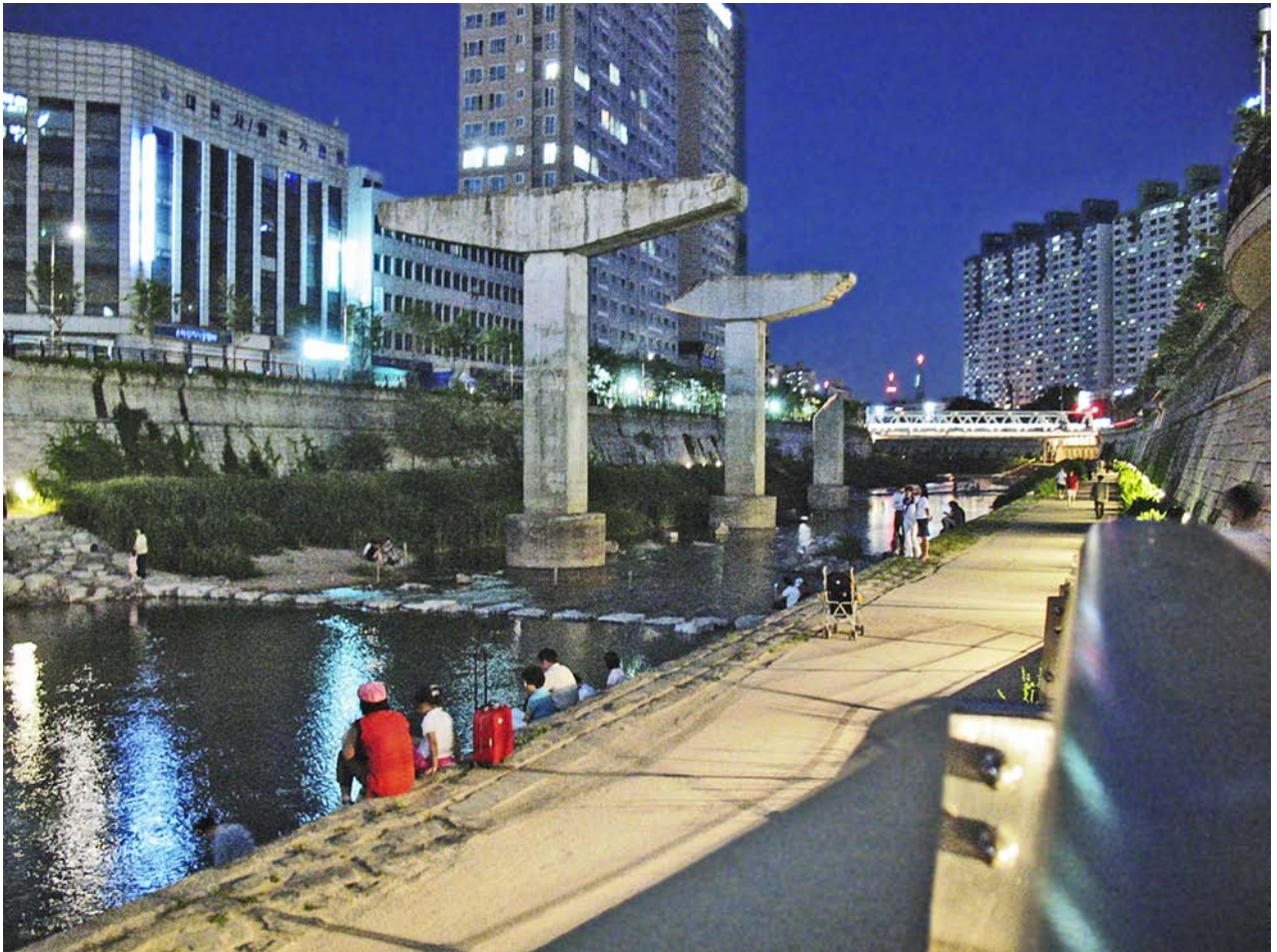
Figure 3.58: Cheonggyecheon, Seoul, South Korea. Remnants of the highway after its demolition. © 2007 Kyle Nishioka / Creative Commons Attribution 2.0 Generic license.
