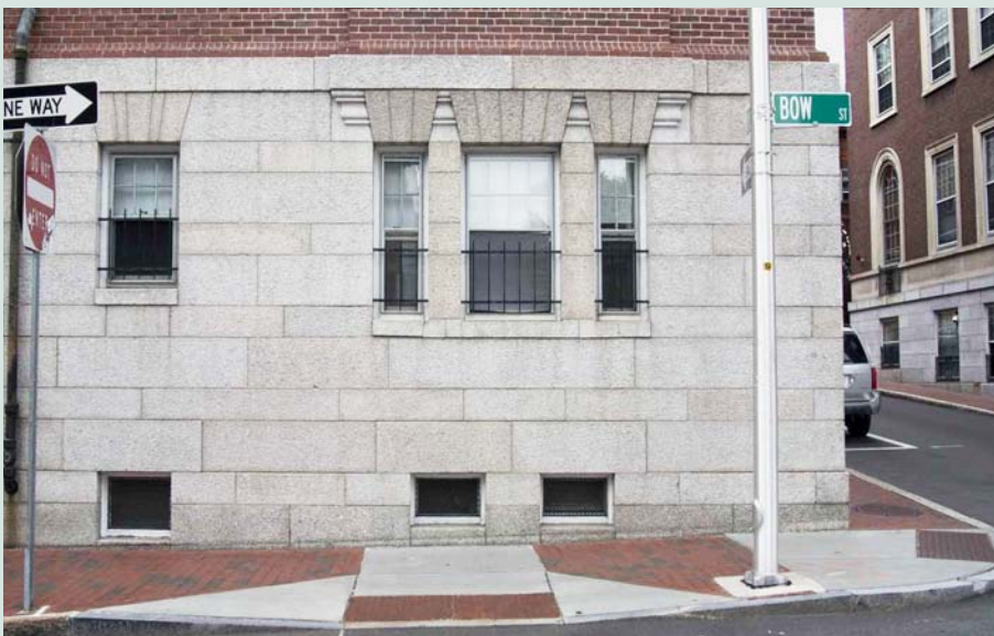
Figure 4.36: Bow Street, Cambridge, Massachusetts. Sidewalk detail. Looking north towards Adams House (Harvard College) at Plympton Street. The Bow Street sidewalk formerly had a ramp detail identical to the one in Figure 4.35, which is one block away. The ugly and unnecessary new detail seen here was put in at considerable expense. Its odd geometry combines with similar details on the other corners and a pedestrian island between Bow Street and Mt. Auburn Street to call attention to the ramps in a jarring way that detracts from the streetscape. A holistic view of the street, rather than a specialist's narrowly focused view, would say the previous detail was both cheaper and better.
