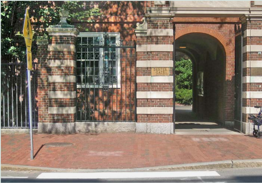
Figure 4.35: Massachusetts Avenue, Cambridge, Massachusetts. Sidewalk detail. Looking north towards Wigglesworth Hall and an entrance to Harvard Yard. The access ramp is simply made by sloping the bricks and tapering the granite curb.
