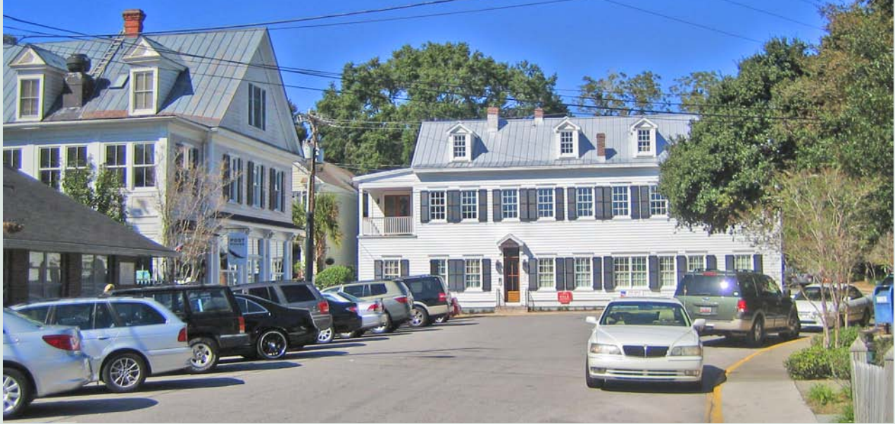
Figure 2.106: Pitt Street, Mt. Pleasant, South Carolina. “That’s not a real town,” goes an old Southern saying, “that’s just a wide spot in the road.” Pitt Street plays slightly to form an extraordinary funnel-shaped space in the Old Village in Mount Pleasant, faced by housing, lodging, the old post office (now a restaurant) and the Pitt Street Pharmacy, arguably the social center of the town. Image courtesy of James Dougherty
