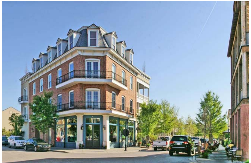
Figure 5.44: Crystal Lake Drive, Hammonds Ferry, North Augusta, South Carolina. Dover, Kohl & Partners, 2005. Mixing businesses, houses, and apartments feels natural at Hammonds Ferry, but it is rare today in newly developed neighborhoods. Image courtesy of Joseph Kohl
