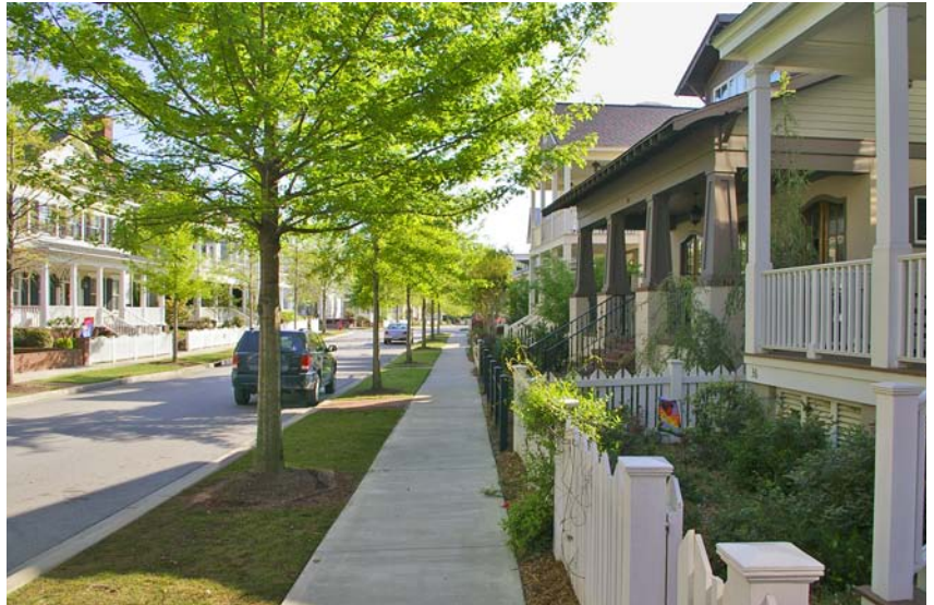
Figure 5.43: Crystal Lake Drive, Hammonds Ferry, North Augusta, South Carolina. Dover, Kohl & Partners, 2005. Front porches, not garage doors, face the street space. Image courtesy of Joseph Kohl
