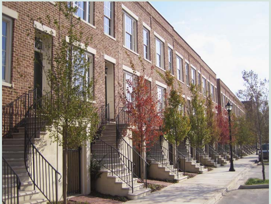
Figure 5.66: Glenwood Park, Atlanta, Georgia. Dover, Kohl & Partners and Tunnell-Spangler-Walsh, 2001. Rowhouses designed by Historical Concepts in 2006 face the public space with their fronts. Image courtesy of James Dougherty
