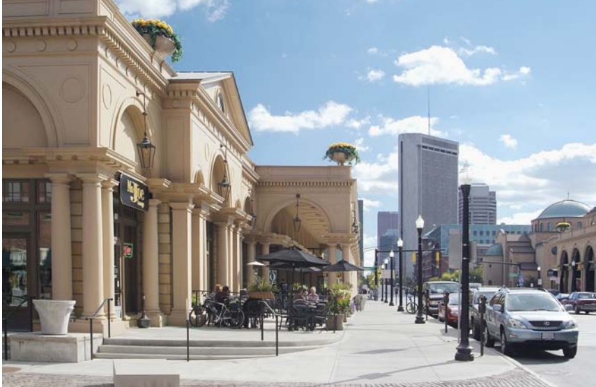
Figure 3.53: The Cap at Union Station, N High Street over I-670, Columbus, Ohio. View looking south on N High Street, showing The Cap crossing I-670. Image courtesy of David Meleca
