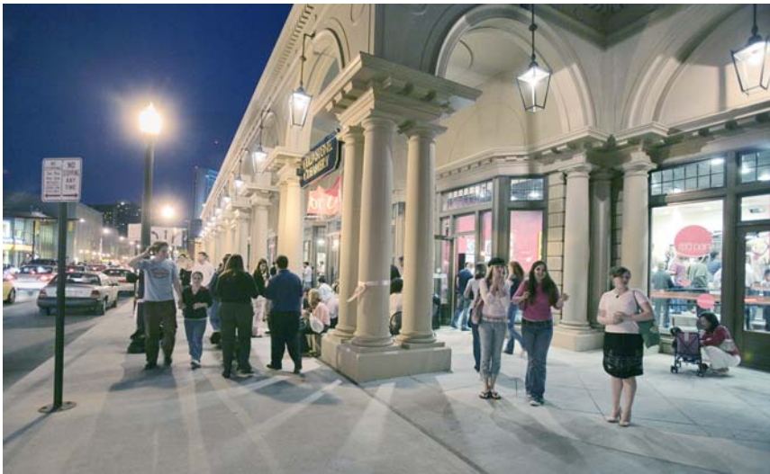
Figure 3.54: The Cap at Union Station, N High Street over I-670, Columbus, Ohio. View showing an arcade at The Cap. Image courtesy of David Meleca
