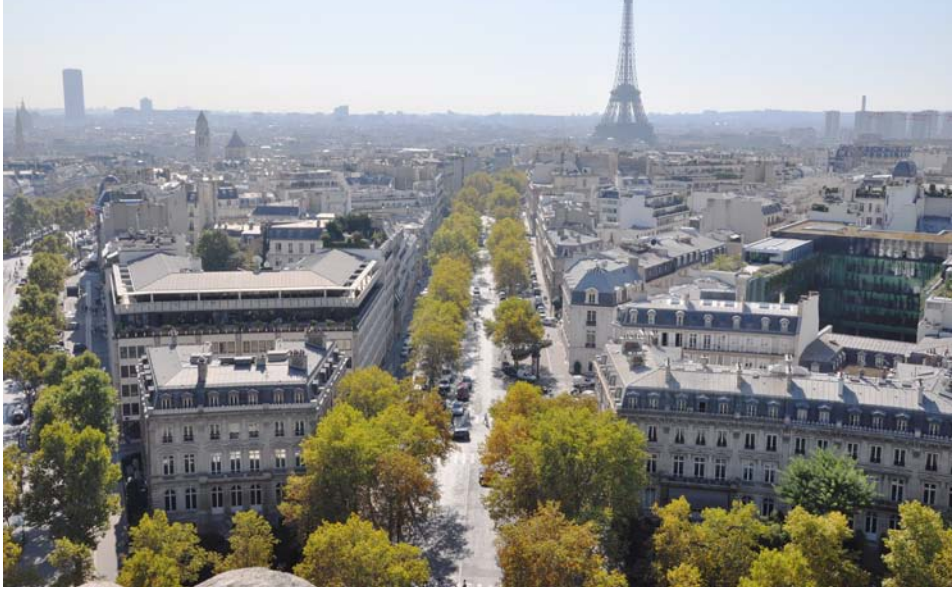
Figure 2.15: Avenue d'Iena, Paris, France. Bureau de la Voirie Parisienne, 1858. Looking south from the top of the Arc de Triomphe. The most beautiful parking lot in the world.
