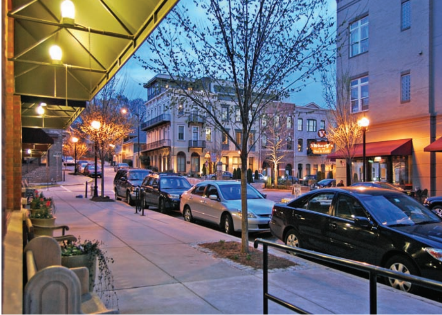
Color Plate 34: Garrett Street, Glenwood Park, Atlanta, Georgia. Dover, Kohl & Partners and Tunnell-Spangler-Walsh & Associates, 2001. View looking east toward Brasfield Square. The development was directed via detailed regulating plans and a form-based code. Approval of the narrow street cross-sections required extensive arm-twisting with reluctant public officials. Image courtesy of Christopher Podstawski
