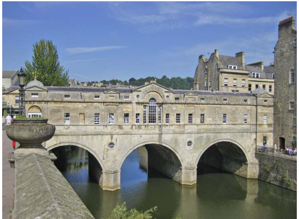
Figure 3.57: Pulteney Bridge, Bath, England. Robert Adam, 1774, later expanded and altered. Spanning the River Avon, the Pulteney Bridge is promoted in Bath as one of four bridges in the world crossing a river that has shops on both sides. The Cap at Union Station shows that the type has tremendous promise for neighborhoods torn apart by half-buried highways.
