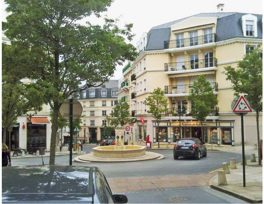
Figure 6.1: Place François Spoerry, Le Plessis-Robinson, France. François Spoerry, 1993. When Philippe Pemezec was elected Mayor of le Plessis-Robinson in 1989, three-quarters of the city's residential stock was dilapidated, twentieth-century public housing. With designs by Spoerry, Xavier Bohl and Breitman Architectes, Pemezec reintroduced traditional streets and buildings to le Plessis-Robinson. The slow speeds in these narrow streets allow the introduction of traditional civic elements like fountains without the need for bold striping and reflective warning signs. Image courtesy of Gabriele Tagliaventi
