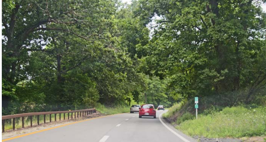
Figure 2.168: Taconic Parkway, Hudson River Valley, New York. Gilmore Clarke, 1925–1949. Looking north on the Taconic Parkway in Dutchess County, New York. The roadways are narrow enough that the trees can make canopies over the parkway.
