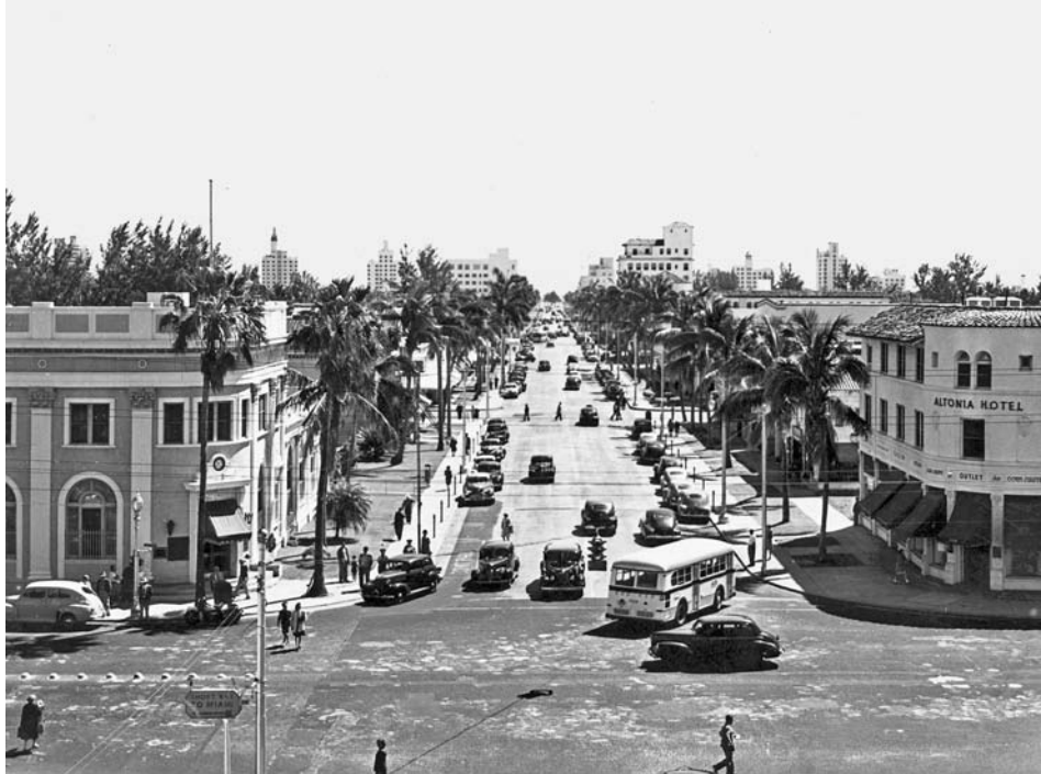
Figure 4.88: Lincoln Road, Miami Beach, Florida. View looking east, circa 1936. The street was open to traffic and lined with tall palms. The asymmetrical Mediterranean Revival silhouette of the Van Dyke Building (1924) is visible in the background, at center right. Image courtesy of HistoryMiami, Archives and Research Center
