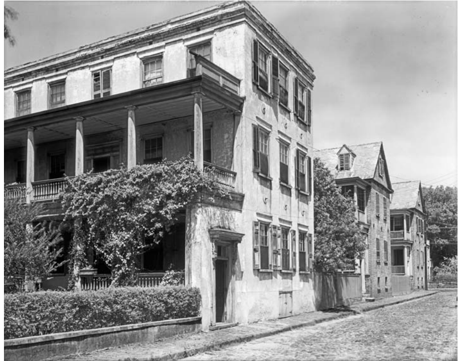
Figure 3.3: Maiden Lane, Charleston, South Carolina. This 1937 photograph of Single Houses on Maiden Lane shows the characteristic house type and streetscape of Charleston. “Single” refers to the one-room width of the houses: they also have a porch facing a side yard, perpendicular to the street. The regular pattern of yard-porch-house along the street establishes a spatial rhythm in Charleston streets. Modern development replaced these particular Single Houses with larger new buildings. Library of Congress, Prints & Photographs Division, Carnegie Survey of the Architecture of the South, LC-J7-SC-1187
