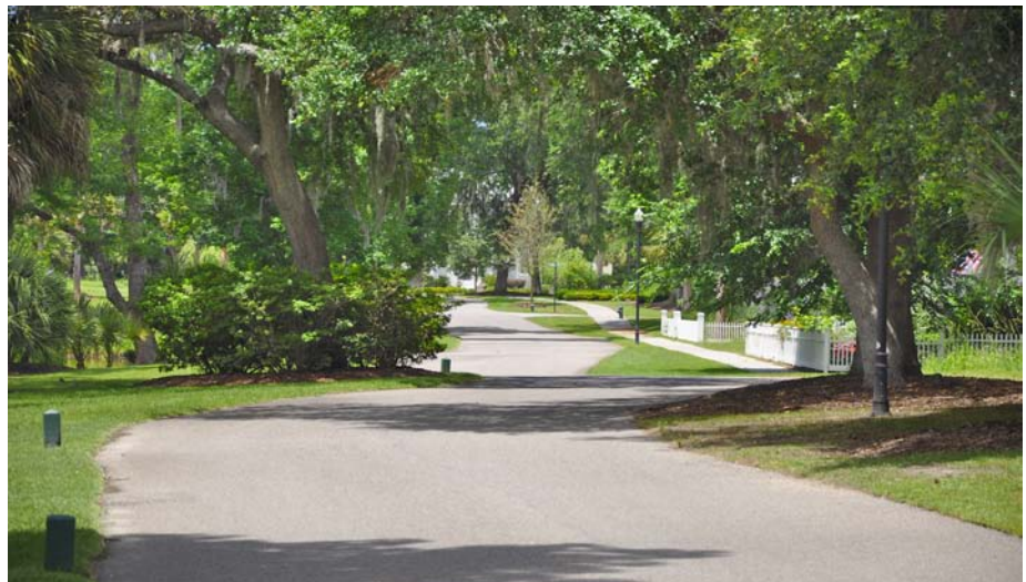
Figure 5.38: South Park Way, Habersham, Beaufort, South Carolina. Duany Plater-Zyberk & Company, 1997. At the neighborhood edge, the Light Imprint street is curbsless and winding, saving mature trees.
