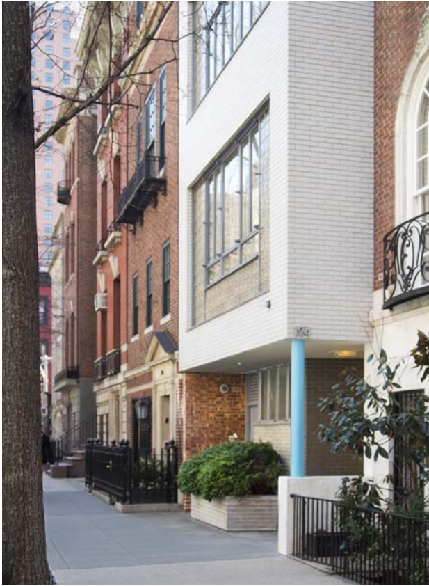
Figure 1.21: Edward A. Norman House, 124 East 70th Street, New York, New York. William Lescaze, 1941. The thin column, the wide, horizontal openings, and the shallow brick veneer of the Lescaze house all emphasize that the facade is a curtain wall rather than a structural, load-bearing wall. That is one of the reasons why the house has a different effect on the streetscape than the neighboring houses.
