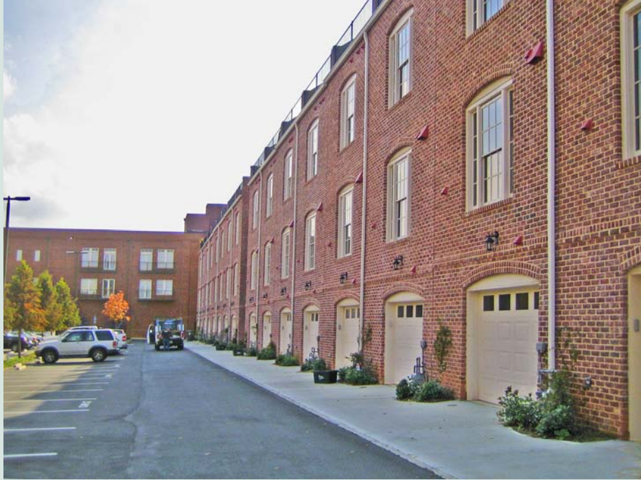
Figure 5.67: Glenwood Park, Atlanta, Georgia. Dover, Kohl & Partners and Tunnell-Spangler-Walsh, 2001. The garage doors and midblock parking areas for the row-houses designed by Historical Concepts are on the alley side. Image courtesy of James Dougherty
