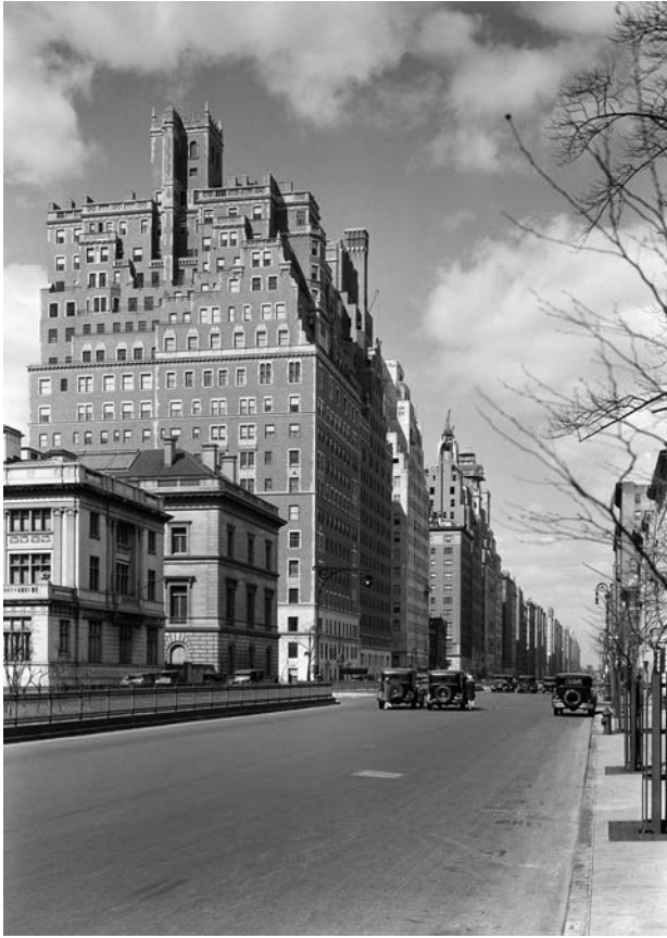
Figure 2.35: Park Avenue, New York, New York. Looking north from 68th Street in 1930. The large apartment house on the west side of Park Avenue at 70th Street is 720 Park Avenue, designed by famous New York apartment architect Rosario Candela in 1929. Older buildings on Park Avenue were limited to a 150-foot height by fire regulations. The City's 1929 Multiple Dwelling Act allowed taller buildings, if they set back above 150 feet. Several wonderful examples of what could be done were quickly built on Park Avenue around 70th Street (some still under construction in this photo). Compare this to Figure 2.33, which shows a slightly less wealthy section of Park Avenue, where development took longer to recover. Image courtesy of the Museum of the City of New York
