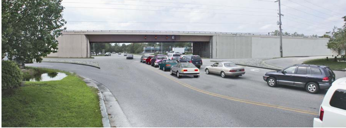
Figure 1.38: Johnnie Dodds Boulevard, Mount Pleasant, South Carolina. A simulation of the Highway Overpass scenario, 2005. © 2005 Dover, Kohl & Partners / UrbanAdvantage
