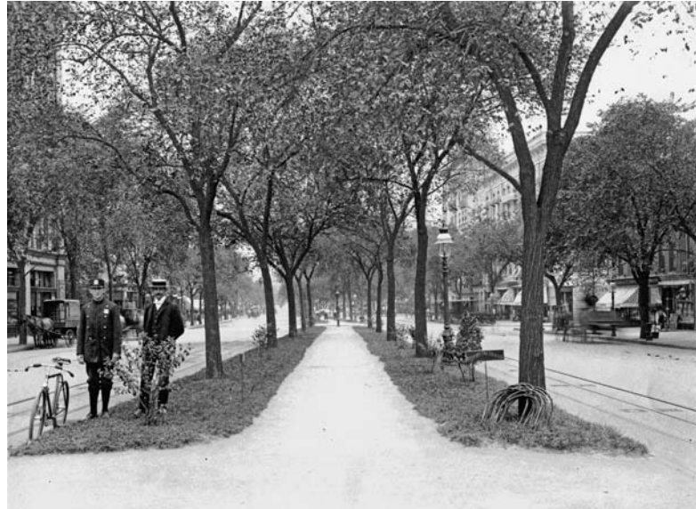
Figure 2.36: Broadway at 85th Street, New York, New York. A view looking north in 1900, showing an informal promenade down the center of the boulevard that preceded the “cut and cover” construction of the West Side IRT subway in 1904, when the median was frequently used for venting the subway platforms. Image courtesy of New York Transit Museum
