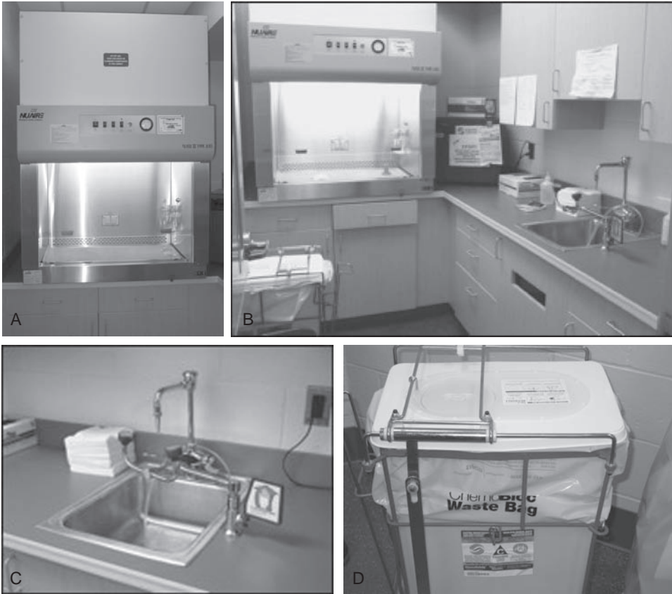
Figure 5.24. Laminar flow hood for chemotherapy drug preparation (A). Typical well-ordered room for chemotherapy preparation (B), containing a sink specifically designated for chemotherapy (C) and specialist waste disposal (D).
