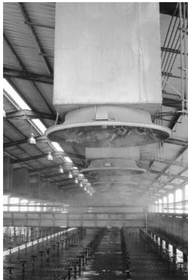
Fig. 71.2 Coolers over a collecting yard. Note the udder washers on the floor.
