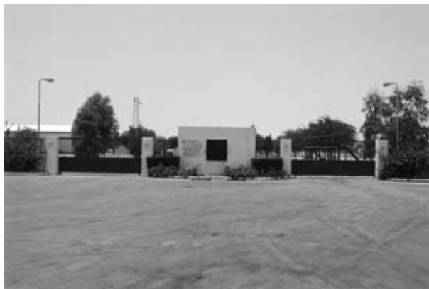
Fig. 71.3 A farm gatehouse, which is controlled to reduce the risk of foot-and-mouth entering the farm.
