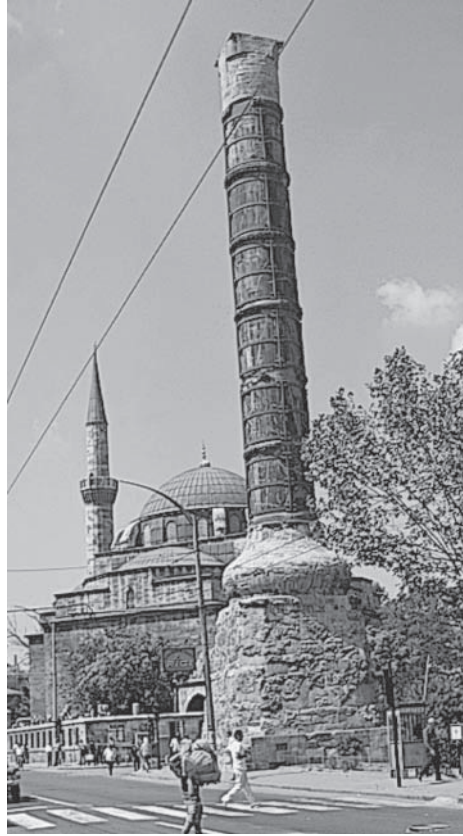
Figure 3.2 Column of Constantine, Constantinople. Roman emperors had commonly erected monumental columns to honor themselves and their military victories; several of these survive in Rome, including the column of the Byzantine emperor Phokas (610–17). Constantine erected this column in Constantinople and it became, in many ways, the center of the city. The column was surrounded by a round colonnade, creating thus the Forum of Constantine, and the main street of Constantinople (the Mese, or “Middle Street”) passed through the monumental complex. Later emperors, when successful in war, passed from the Golden Gate, through the Forum of Constantine, to the palace complex. The column was surmounted by a statue of Constantine, which had been made by re-carving a statue of the god Apollo in order to give it the features of the emperor. According to one tradition, Constantine had the nails from the Crucifixion and the Palladium built into the column – the latter was the sacred cloak of Athena, which had been brought to Italy from Troy after the sack of the city and became the special protection of Rome. According to another tradition, Constantinople would never fall to any of its enemies as long as the sculpture remained in place. Photo: Timothy E. Gregory
