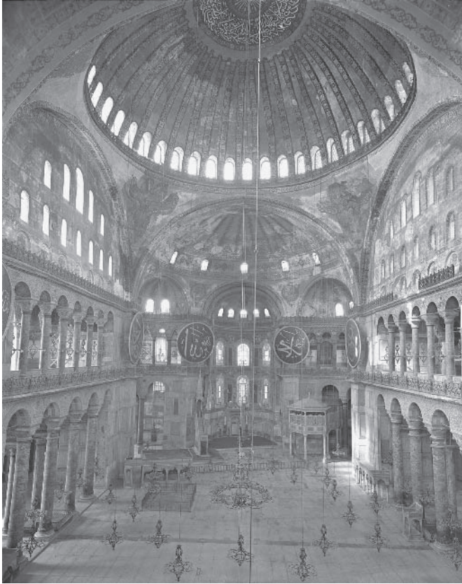
Figure 6.3 Hagia Sophia, interior. This view of the interior of Hagia Sophia, looking east toward the apse where the altar was, captures something of the immense inner space of the building. The original dome collapsed in 558 and was rebuilt and dedicated in 562. Earthquakes and the wear of time caused other problems but these were all repaired with the resources available at the time, but the result is that the building today is considerably different from what it was when first built; one aspect of this is that the original windows were much larger, letting in even more light and “opening up” the interior even more than they do now. The Arabic inscriptions and the furniture were added after the building was converted to a mosque in 1453. It is now a museum. Photo: Dumbarton Oaks
