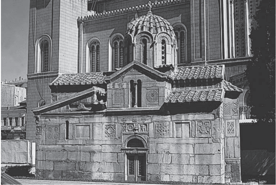
Figure 12.4 “Little Metropolitan,” Athens, ca. 1200. This small cross-in-square church in Athens is unusual in that it was built completely of marble blocks, reused from earlier structures. These blocks include a representation of the ancient goddess Athena, allusions to the cult of Eleusis, and the only surviving depiction of the Panathenaic procession. Many ancient funeral reliefs were also employed, frequently modified to include crosses. Photo: Timothy E. Gregory
