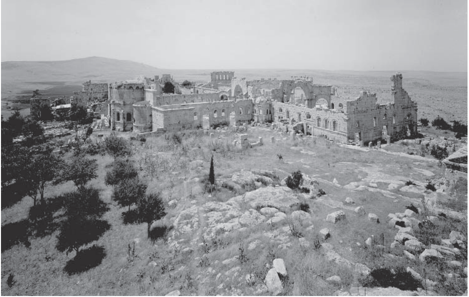
Figure 5.5 Qal'at Sem'an. This pilgrimage complex in northern Syria was built around the column of Symeon Stylites the Elder ca. 476–90. Symeon had already died by this time but his fame was such that an unknown donor (possibly the emperor) had a large octagon constructed around the column along with four basilicas radiating out from it. A monastery was constructed in the vicinity and, after the Arab invasions, it was refounded in the tenth century. Photo: Dumbarton Oaks / Richard Anderson
