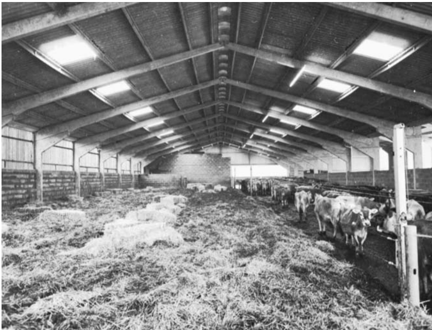
A dairy unit, with lying area, parlour and dairy under one roof. Note the Yorkshire boarding to the left of the picture – a means of ensuring good ventilation and an absence of condensation.
