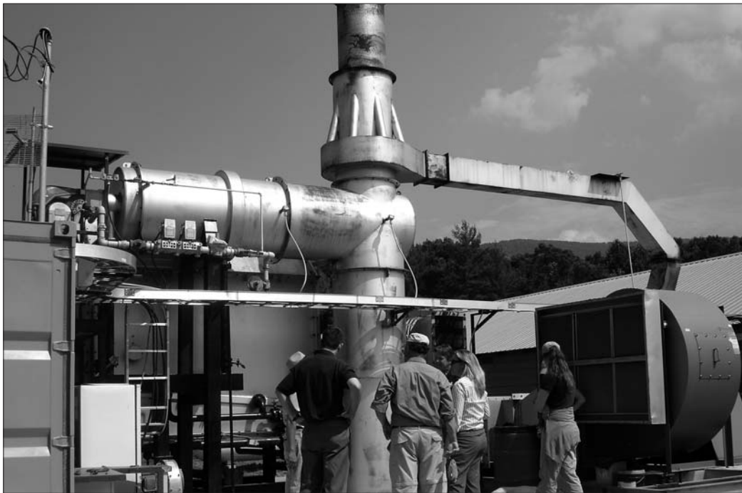
Figure 9.3 Pyrolysis unit and adjacent poultry house, Wardensville, West Virginia: biomass feedstock and energy demand are co-located with matching energy and manure disposal needs
