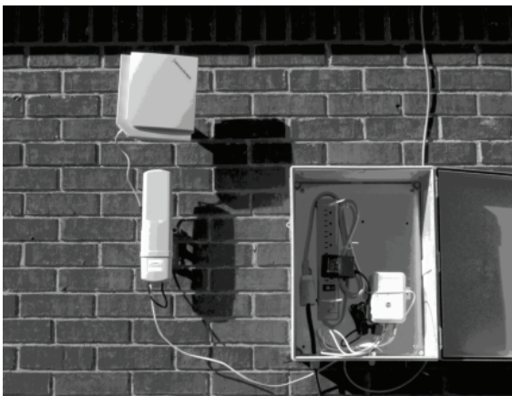
Figure 5. Outdoor antenna mounted at end user site 9 km east of the base station. Antenna and radio are shown on the left with the antenna on top with the radio mounted below. The NEMA 4 box contains the surge protected power strip mounted on the left side interior of the box along with the power converter which supplies 24 VDC power over Ethernet (POE) to the radio, and antenna lightning protector shown mounted on the lower right
