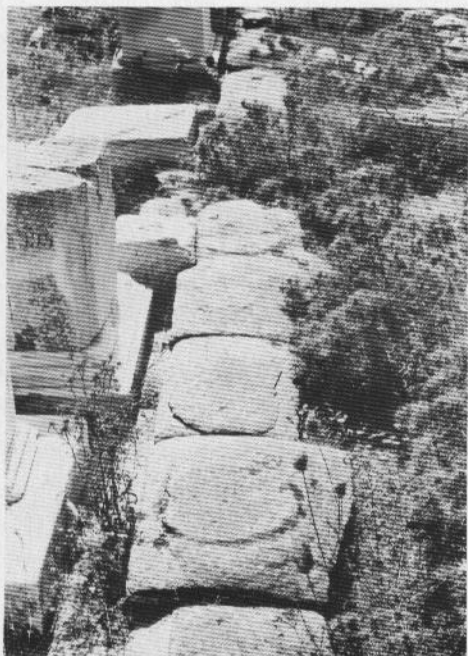
Plate 2 a. Delos: Stylobate of southern façade with de- dicatory bases on steps, from east.
