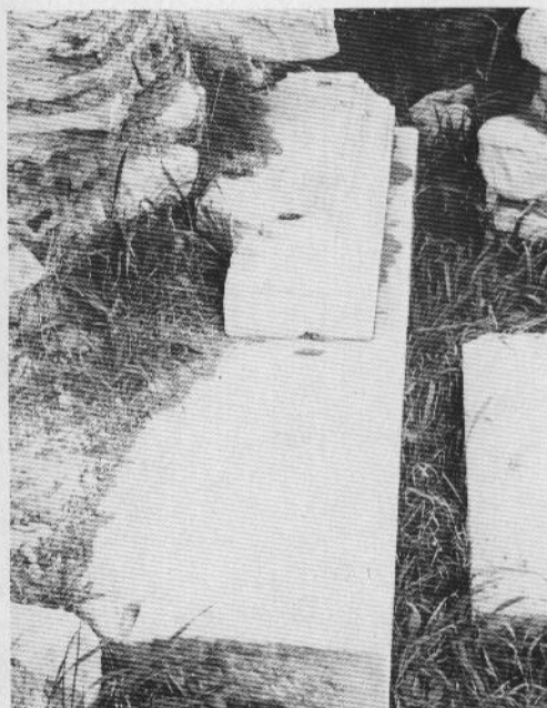
c. Ephesos: Northeast corner of altar in east court with first step and western re- turn of base moulding, from south.
