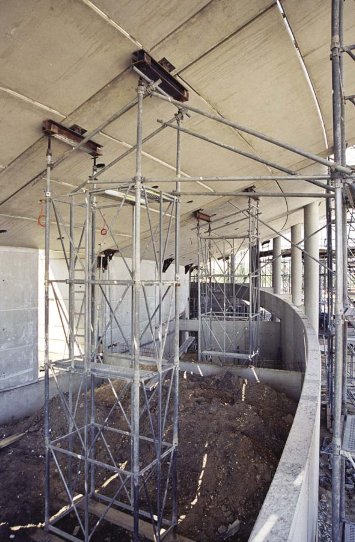
Precast concrete work
