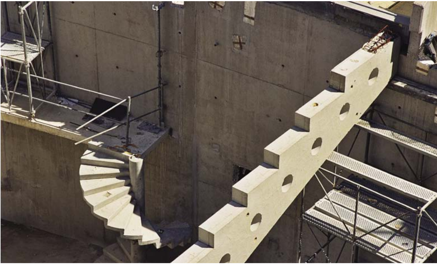
Precast concrete seating construction
