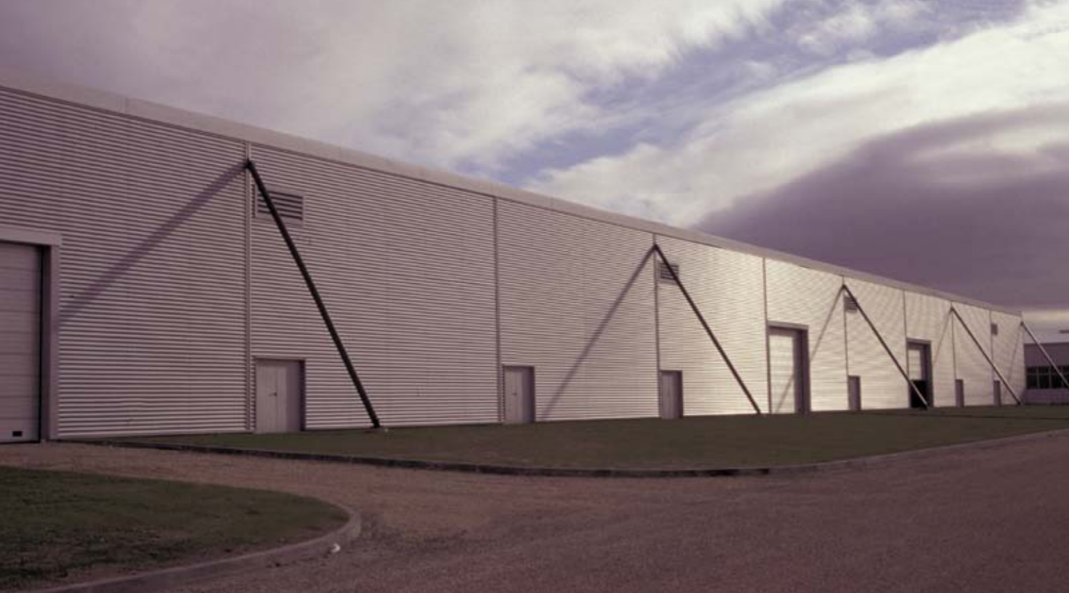
West facade of Hall 7 with exterior lateral bracing
