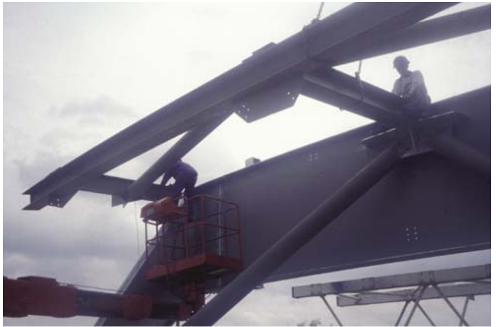
Views of transition structure assembly
