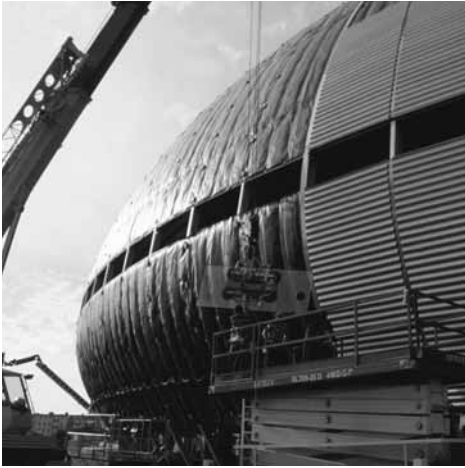
Cladding installation
