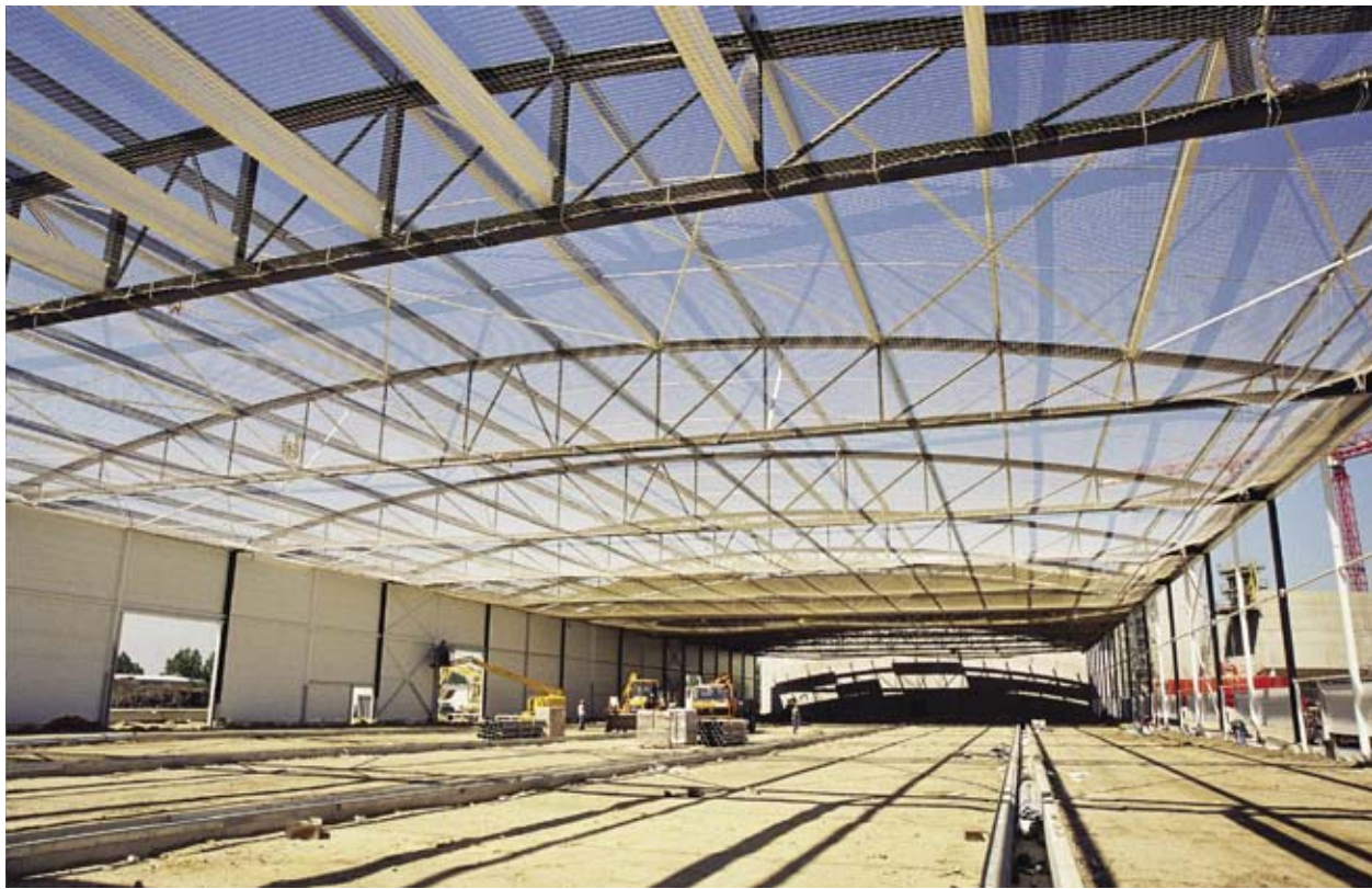
top and left: Hall 7 during construction
