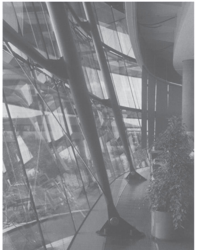
8.4 First floor interior looking along the façade. Note the air supply grille on the floor, the roller blinds and the open space to the second floor above.
