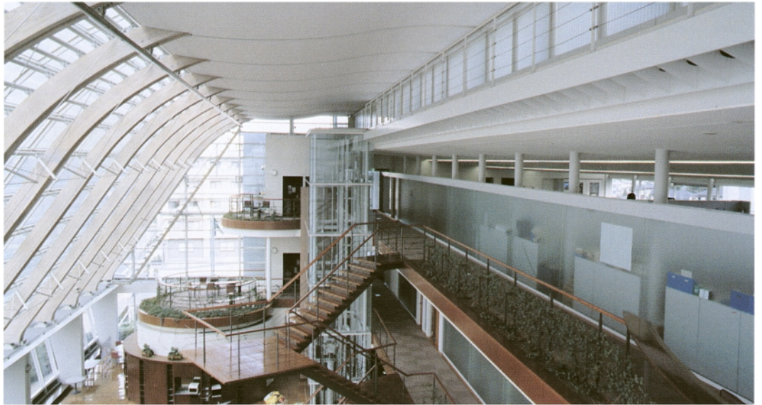
Plate 23 The Eastgate Centre, Harare—upper section of the atrium showing the large gap for airflow between roof and canopy.
