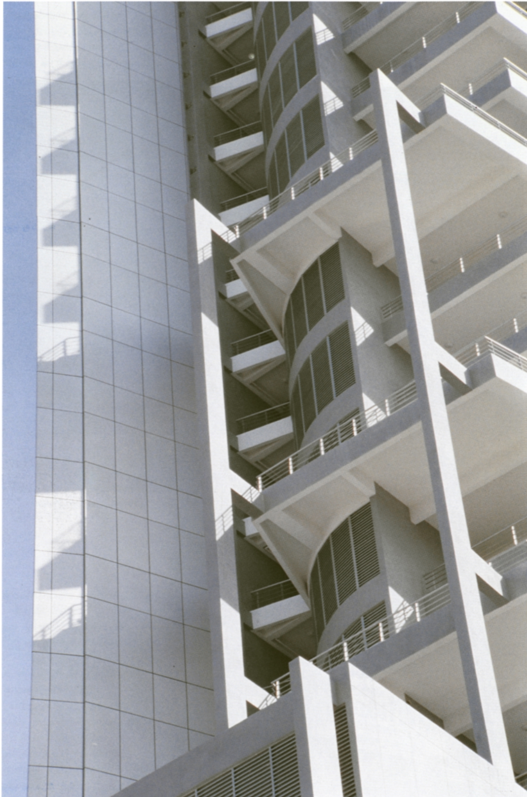
Plate 33 Menara UMNO, Penang—north-east-facing wing wall.
