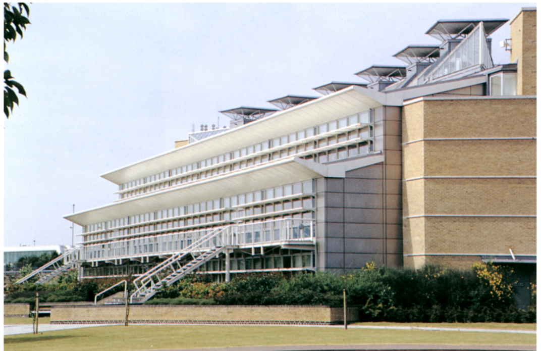
Plate 2 Ionica Headquarters, Cambridge —south façade solar shading. Note also the six ventilation towers above the roofline.
