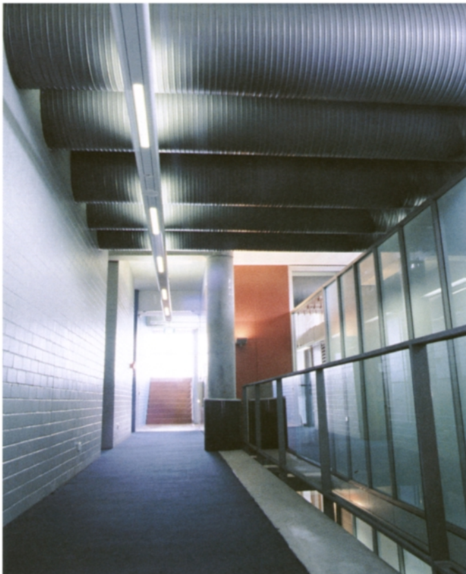
Plate 25 UNSW Red Centre, Sydney—'airshaft' between Levels 3 and 4, and horizontal sections of some of the ventilation chimneys.
