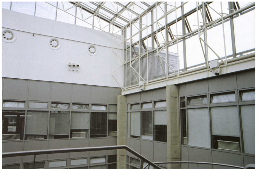
Plate 15 The Scottish Office, Edinburgh —upper level inside one of the atria. Note the mechanical ventilation extract grilles and the motorised window openings as well as the venetian blinds and hopper windows of the adjacent third floor office.
