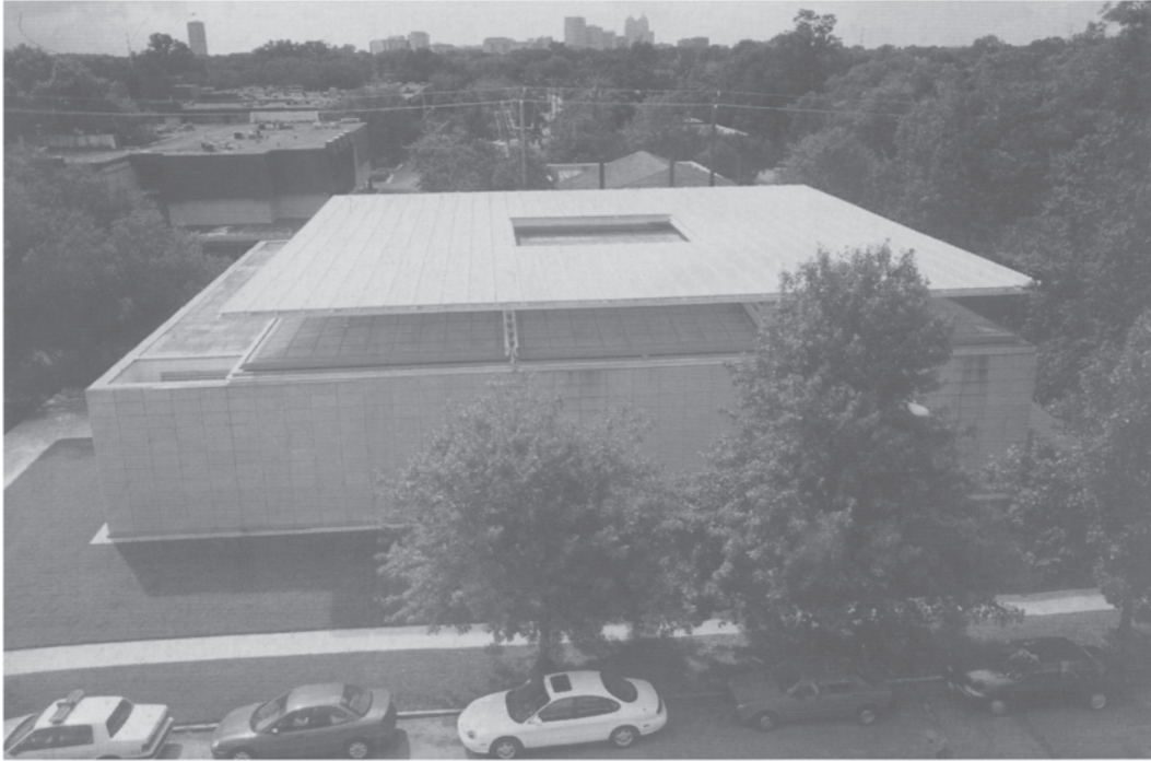
3.13 Cy Twombly Gallery—view from the roof of the Menil Museum. The topmost layer of fixed louvres shields the glazing below from high-altitude angle direct solar radiation.
