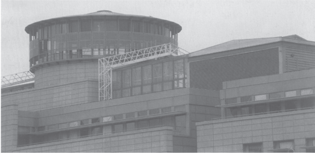
9.11 Close up of the top of the rotunda (note the solar shading) with the top of the adjacent atrium and a flanking plant room on the right.
