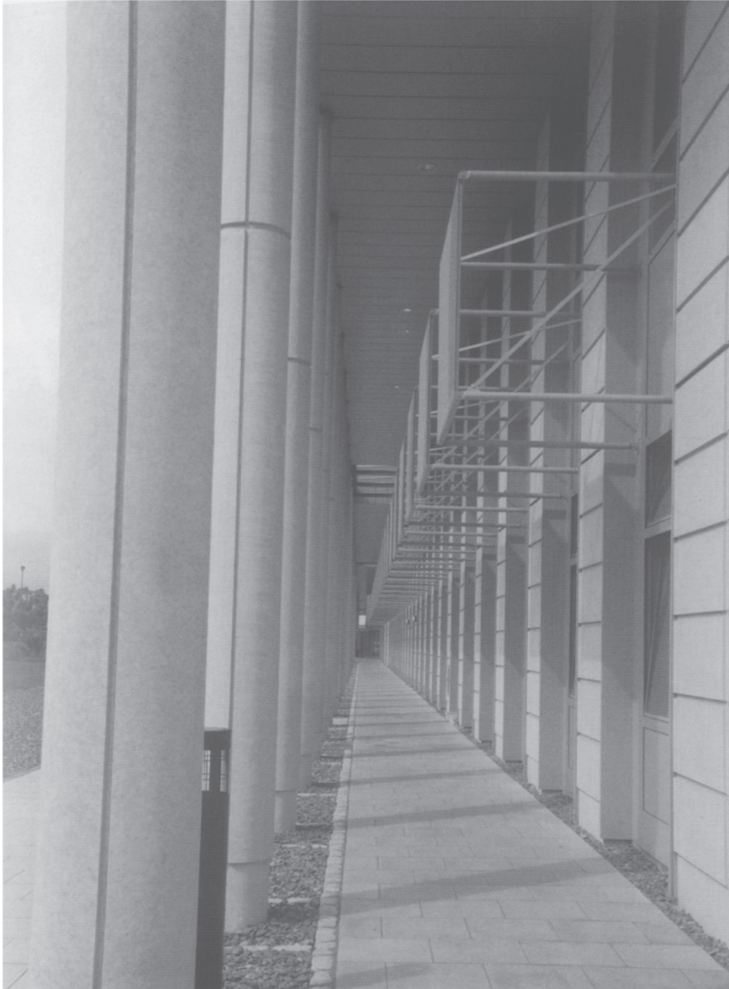
9.10 View along the colonnade.
