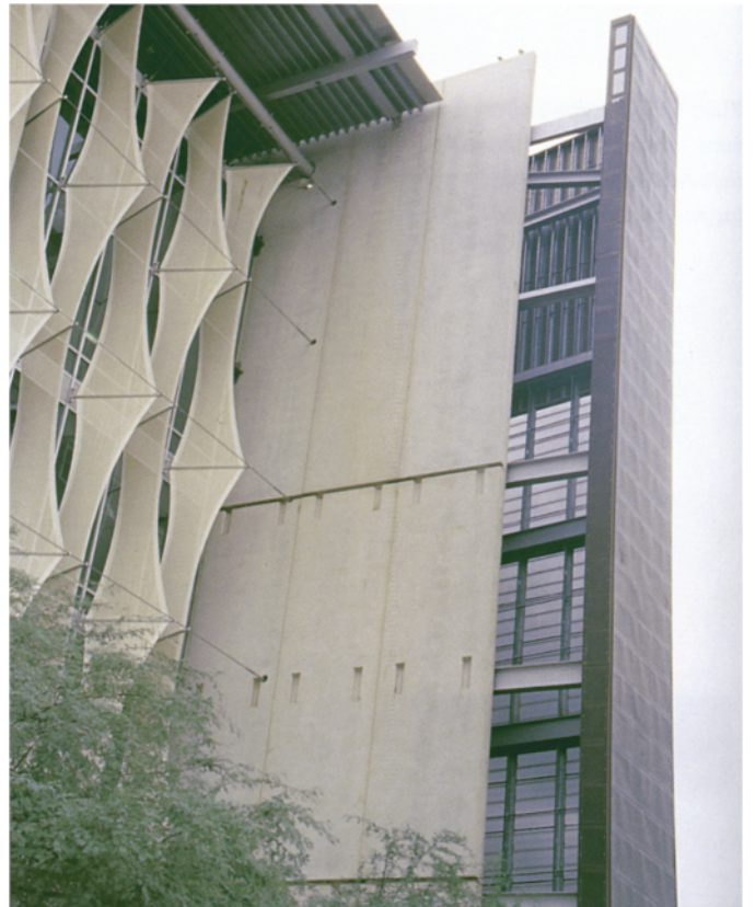
Plate 11 Central Library, Phoenix—north façade showing the fixed vertical shades and the open end of the saddlebag at the north-west corner.
