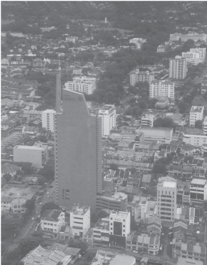
18.1 Looking north-west towards the building from the KOMTAR.
