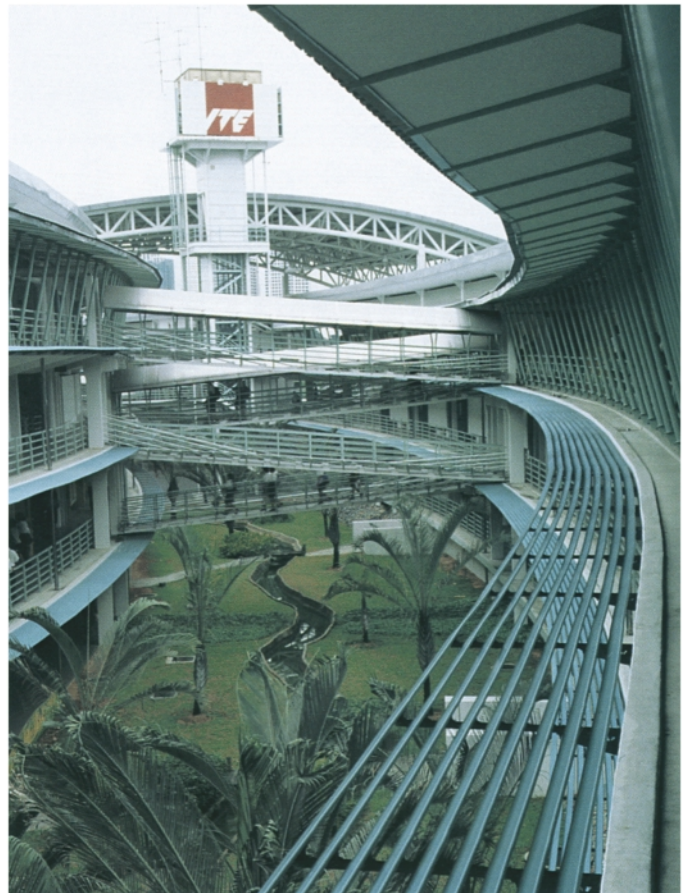
Plate 4 ITE Bishan—looking southwards along the landscaped internal street. Note the louvred extensions from the walkways and (upper background) the open roof over the amphitheatre.
