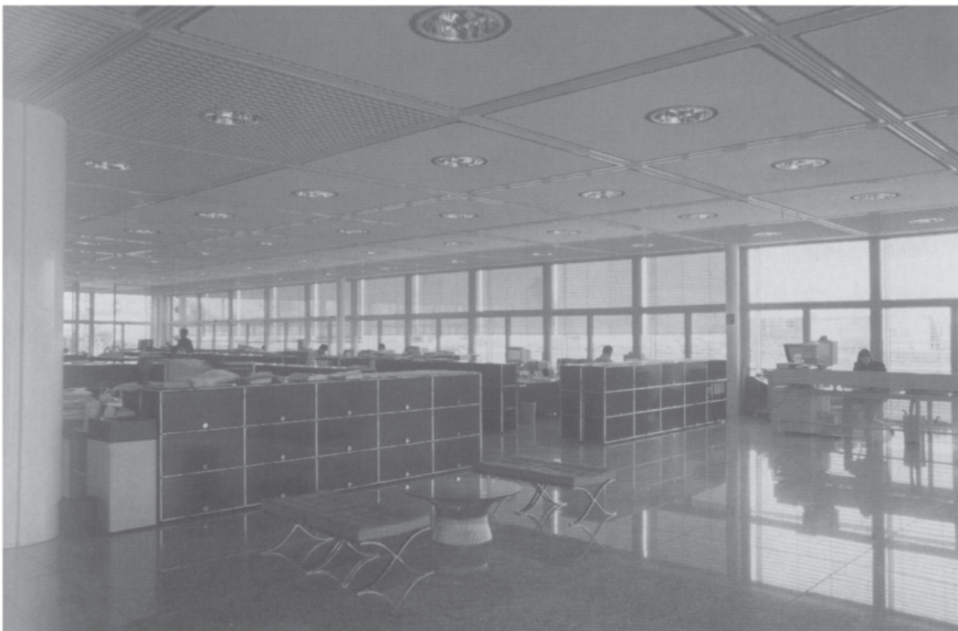
6.9 General view of part of the ground floor office space. Note the granite floor in which heating/cooling coils are embedded, and the slots in the false ceiling that enable air circulation to the slab above. The egg-crate arrangement seen in some parts of the ceiling incorporates cooling coils.
