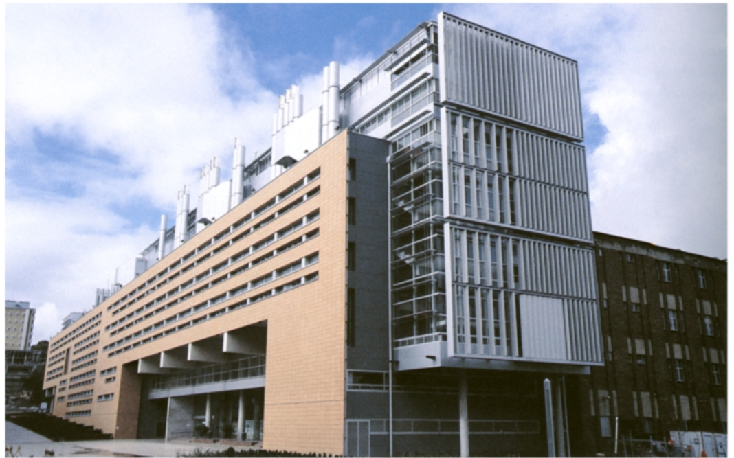
Plate 25 UNSW Red Centre, Sydney—'airshaft' between Levels 3 and 4, and horizontal sections of some of the ventilation chimneys.
