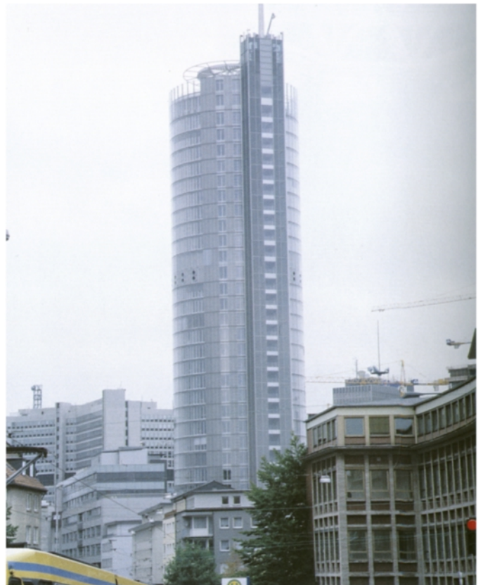
Plate 26 RWE Headquarters, Essen—view of the building from Gutenbergstrasse. Note the lift tower to the south-east.
