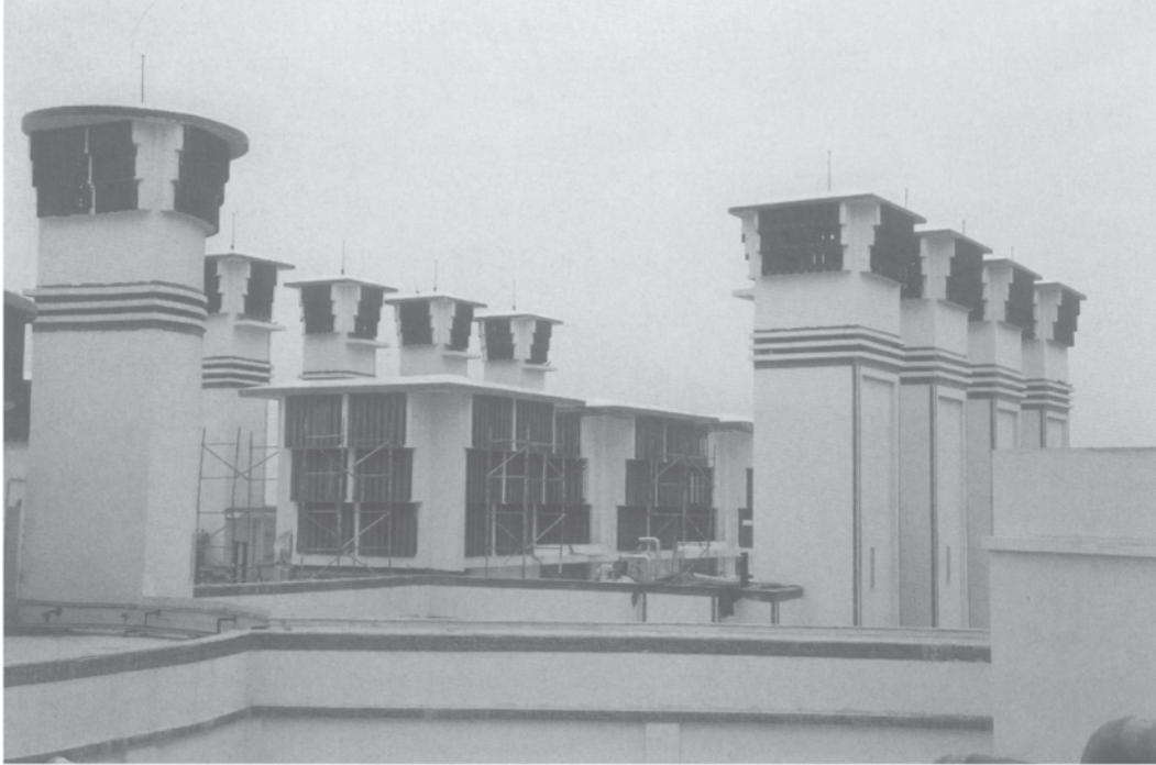
17.5 View across the roof of a Laboratory Building from the roof of the Core Building (No. 7) showing the tops of the air inlet and exhaust towers (the one on the extreme left foreground is an exhaust air tower from the Core Building).
