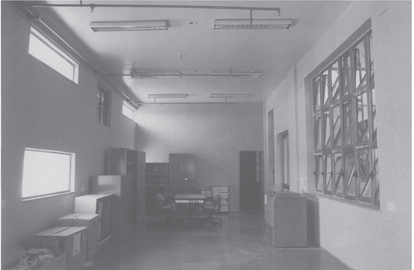
17.15 Typical office space showing the fixed windows and exhaust openings on the left (external) wall and the hopper windows on the right adjacent to the corridor.
