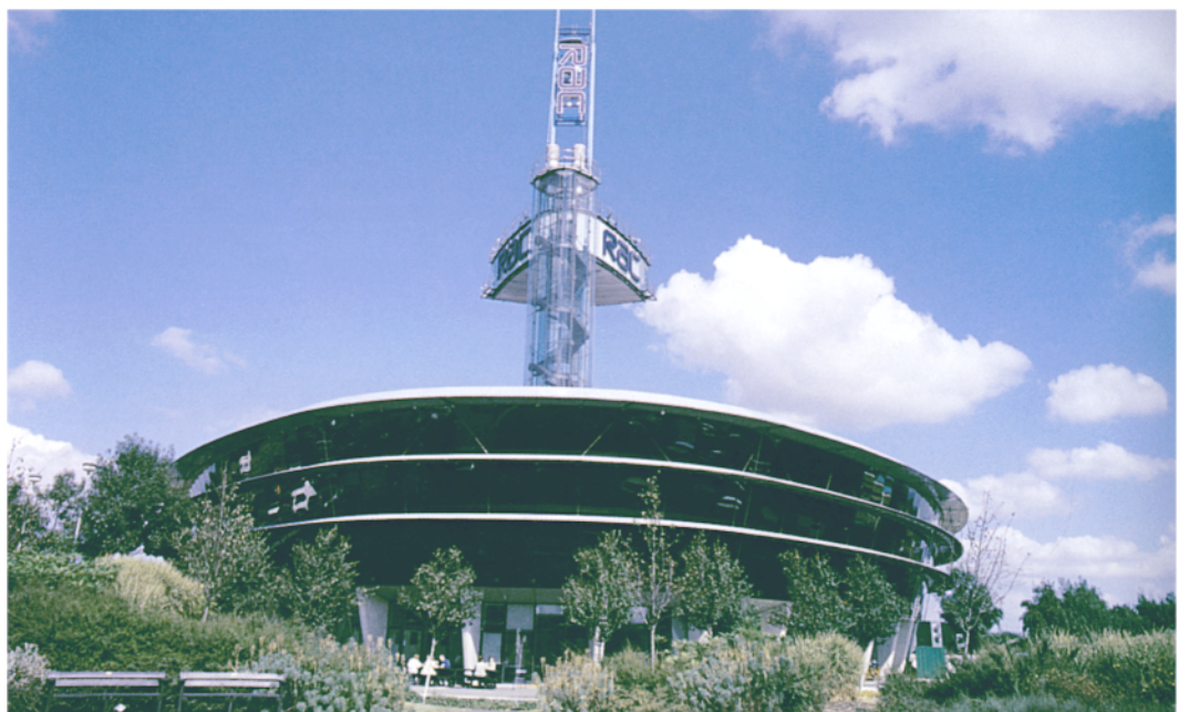
Plate 12 RAC Regional Centre, Bristol—general view of the building from the landscaped area to the south.
