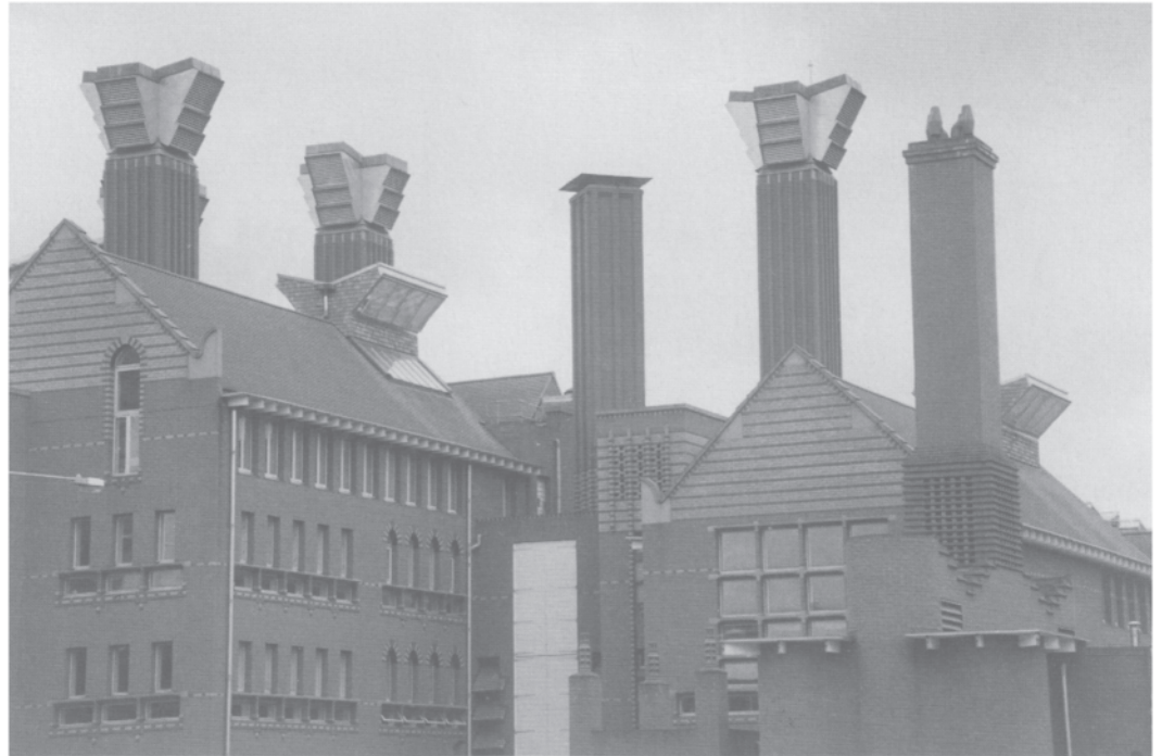
3.32 Queens Building, De Montfort University—portion of the roofscape with a range of ventilation stacks.
