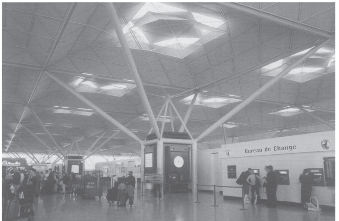
3.9 Stansted Airport—departures side of the concourse. Note the skylighting modules and the structural trees with services pods within their 'trunks'.
