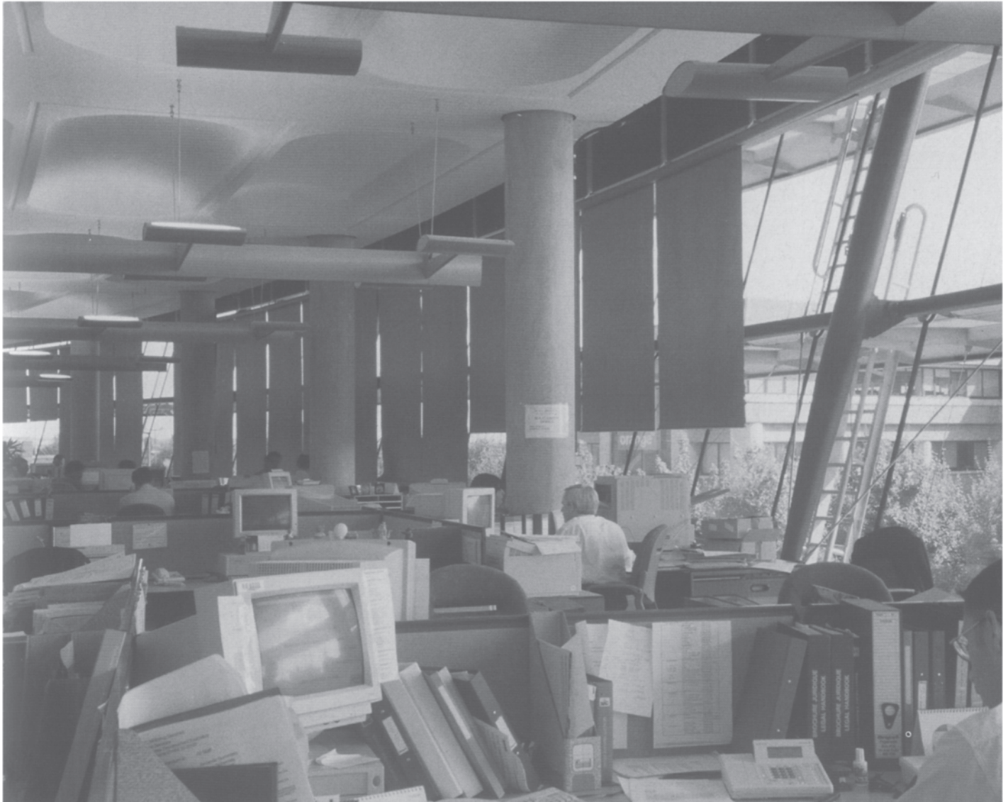
8.11 General view into a first floor office space. Note the roller blinds, the uplighting system and the coffered ceiling.
