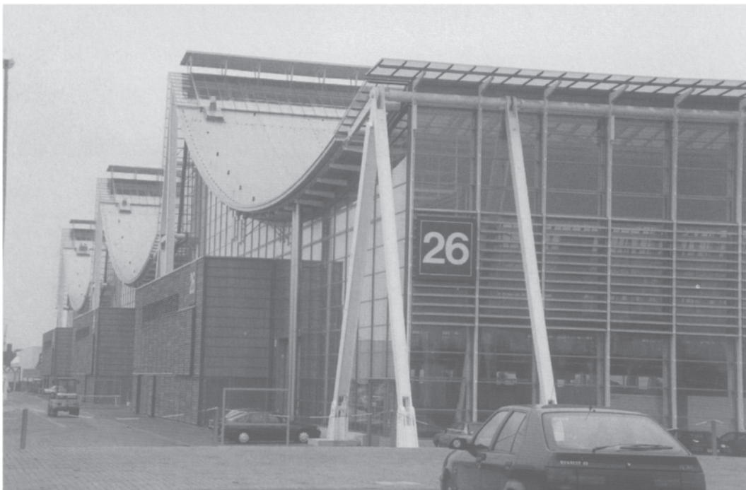
11.7 Exterior view showing the service pods on the west façade and the solar shades on the south.
