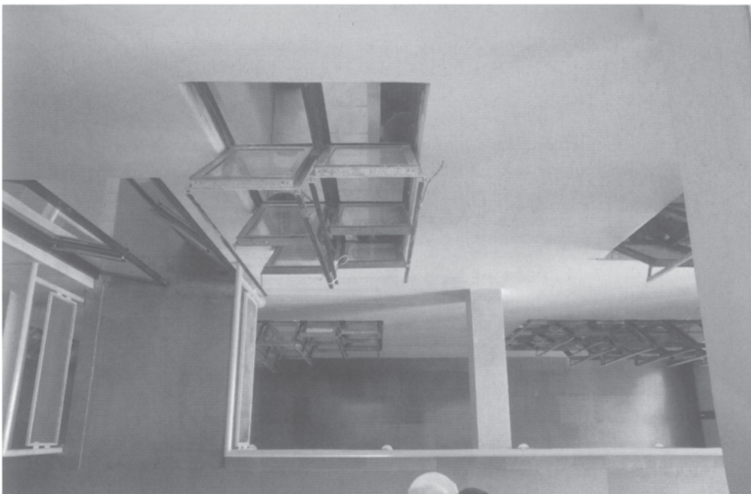
17.13 Looking down from the corridor of the second floor. what the air 'sees' as it descends via the openings in the floors and is diverted by the hopper windows into the adjacent spaces.
