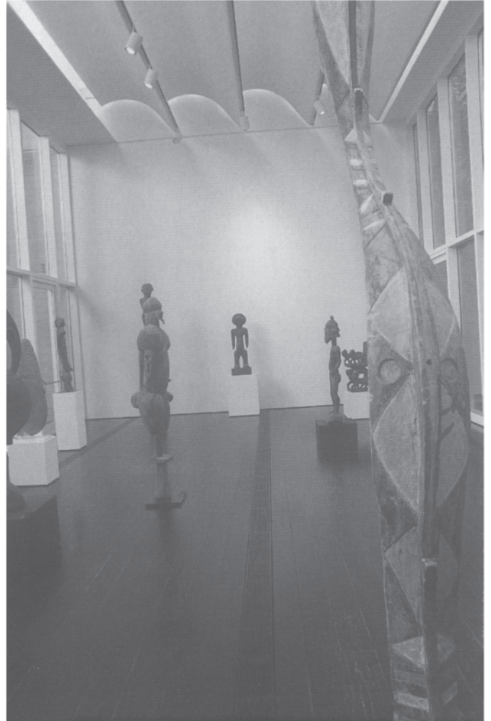
3.11 Menil Museum—typical display space. Note the curved ceiling louvres for direct sun exclusion and the linear floor grille for air supply.
