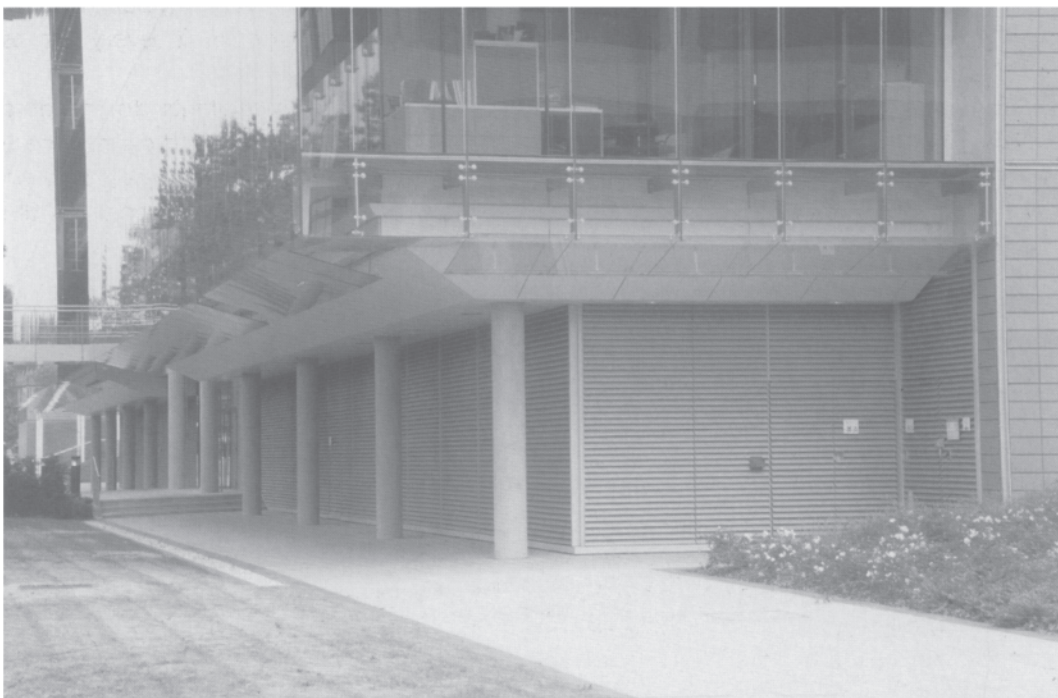
16.12 Lower ground floor at the south-west corner of the building. The main plant rooms are housed behind the louvred façade, both here and at the north-west corner.
