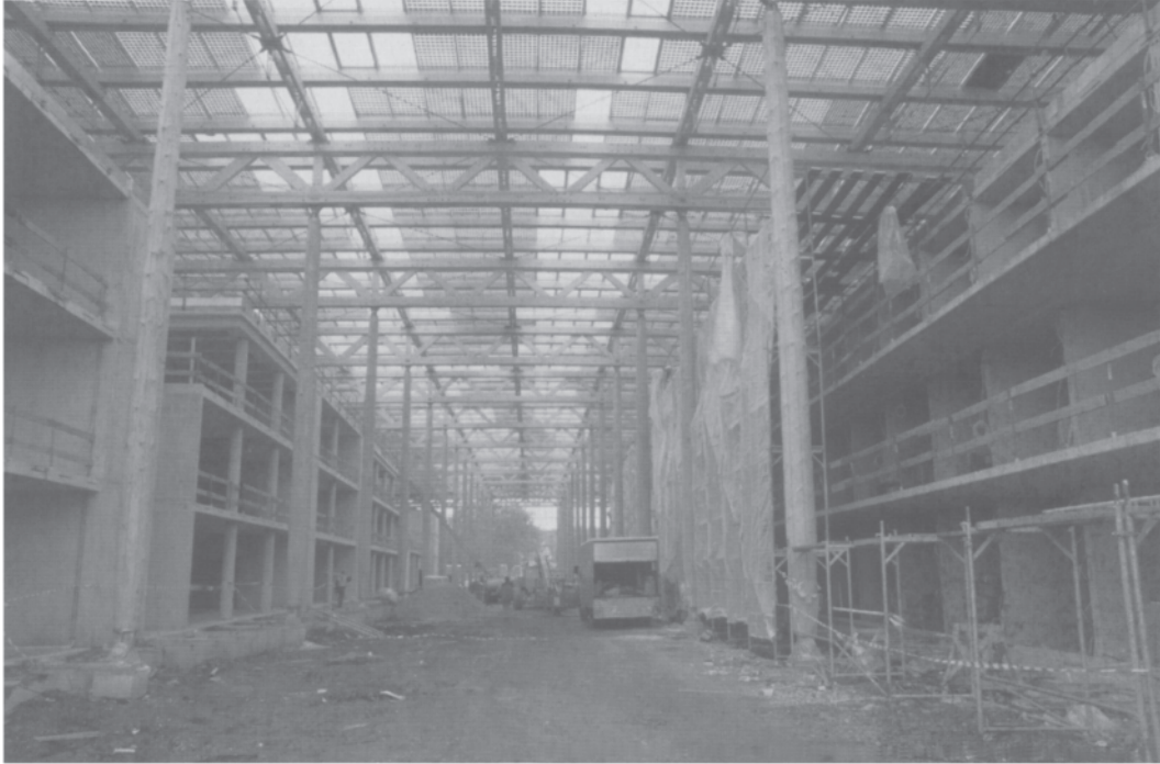
19.7 Government Training Centre, Herne-Sodingen—interior view when under construction in October 1998.
