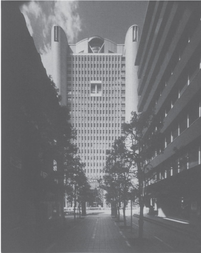
19.5 Liberty Tower, Meiji University, Tokyo—note the ventilation opening in the centre of the ‘Wind Floor’ (Level 18). These are designed into each façade (photo: Kawasumi Architectural Photograph Office).
