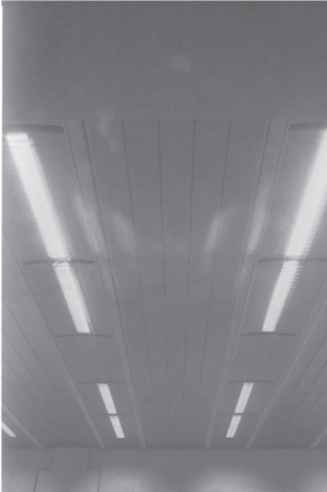
7.8 Perforated ceiling air supply
