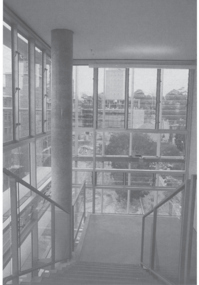
14.14 Stairwell at the east end of the building showing horizontal ventilation louvres and exterior vertical solar louvres: the actuator for the latter is in the centre.
