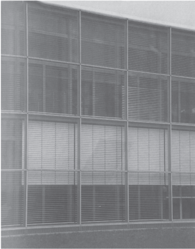
6.8 Section of the façade. Note the louvre configuration on the ground floor level—the upper part reflective, the lower part absorbent
