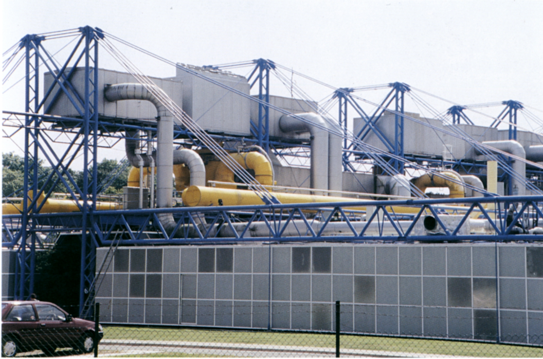
Plate 2 Ionica Headquarters, Cambridge —south façade solar shading. Note also the six ventilation towers above the roofline.
