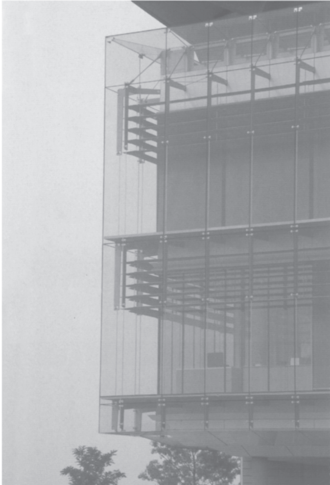
16.10 Southern end of the east façade. The roller blinds on the second floor are fully extended; those on the first floor are fully open.
