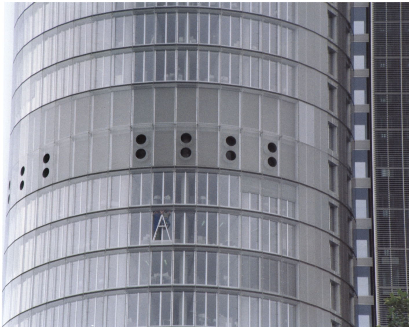
Plate 27 RWE Headquarters, Essen—floors accommodating the central plant (air-handling units and cooling towers mainly) on Levels 17 and 18. Note the placement of the circular air inlets and outlets, and the separate lift tower.
