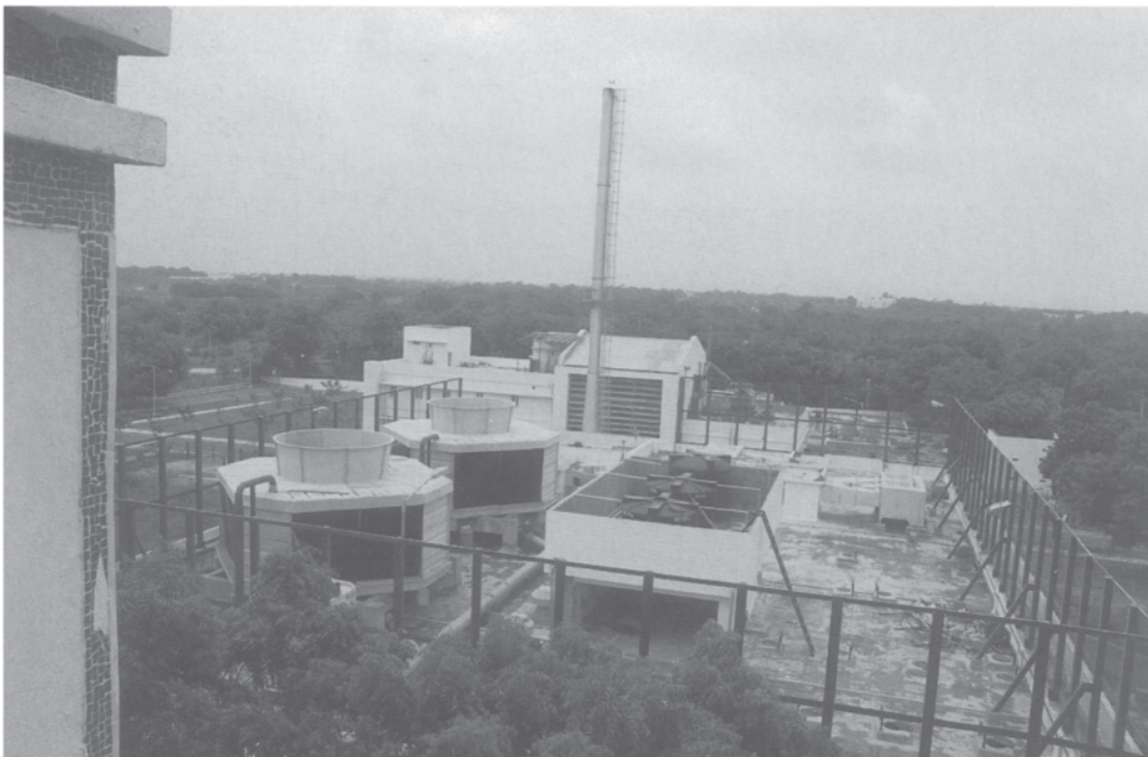
17.6 View from the roof of Building No. 4 across the top of the Utilities Building; cooling towers and boiler chimney are very much in evidence.
