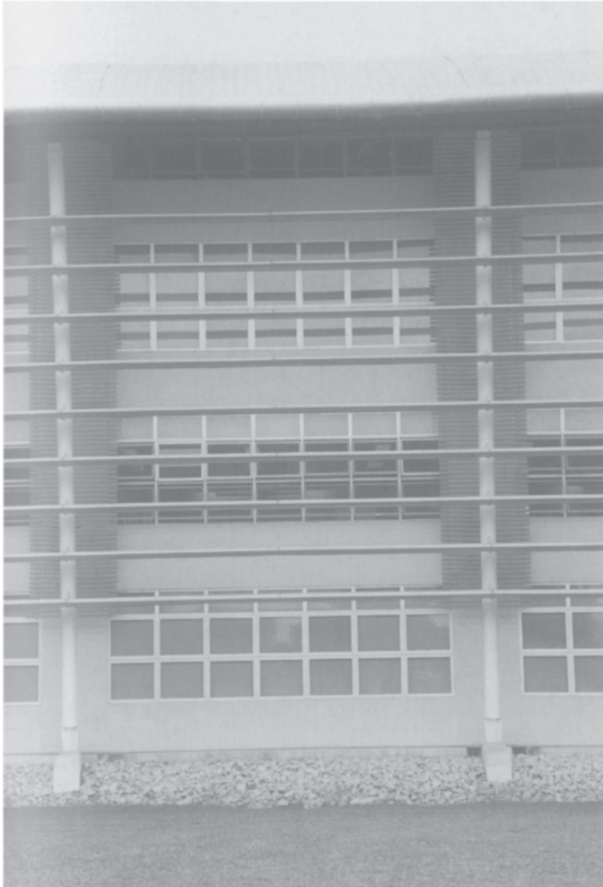
4.11 View of one of the west façade modules. Note the main horizontal solar louvres, the windows and the louvred screens for the condenser units.
