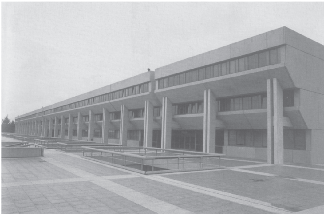
3.30 City University of Udine—south-west façade shape designed to provide shading to the lower floors and at ground level (the north-east façade is similar).
