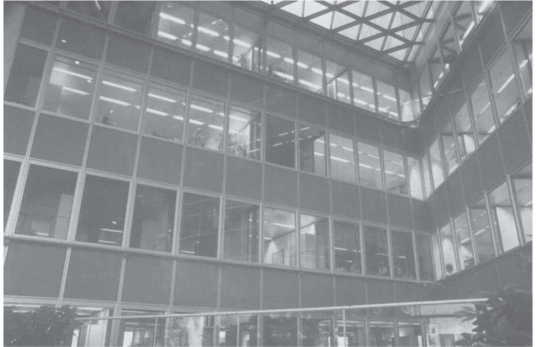
3.47 Commerzbank Headquarters, Frankfurt—looking towards the adjacent office spaces from one of the garden areas. The windows are openable for natural ventilation.
