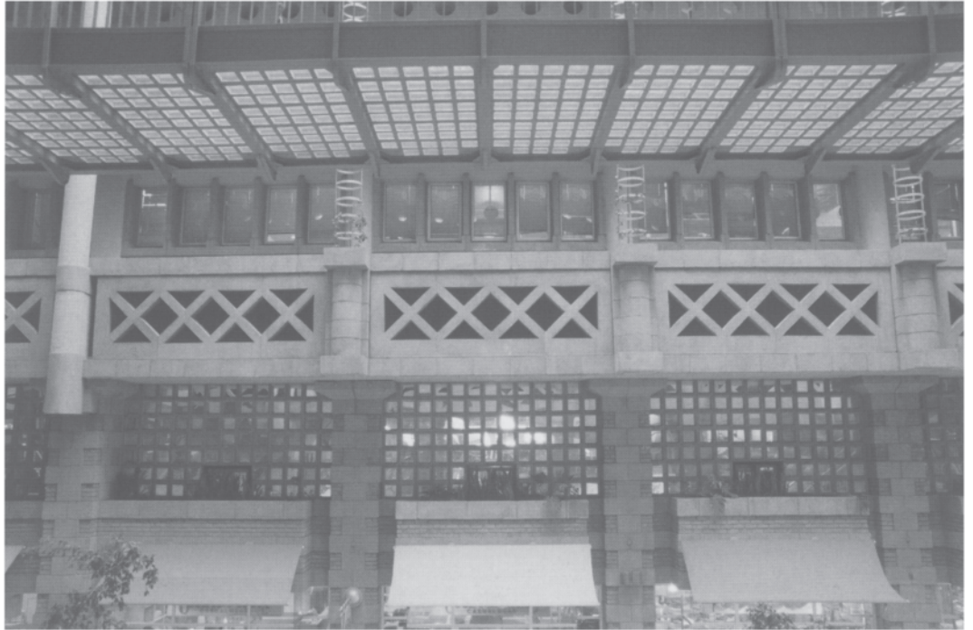
13.15 Fresh air intakes via the cross-chevron screens with a parking area below and the skywalk above.
