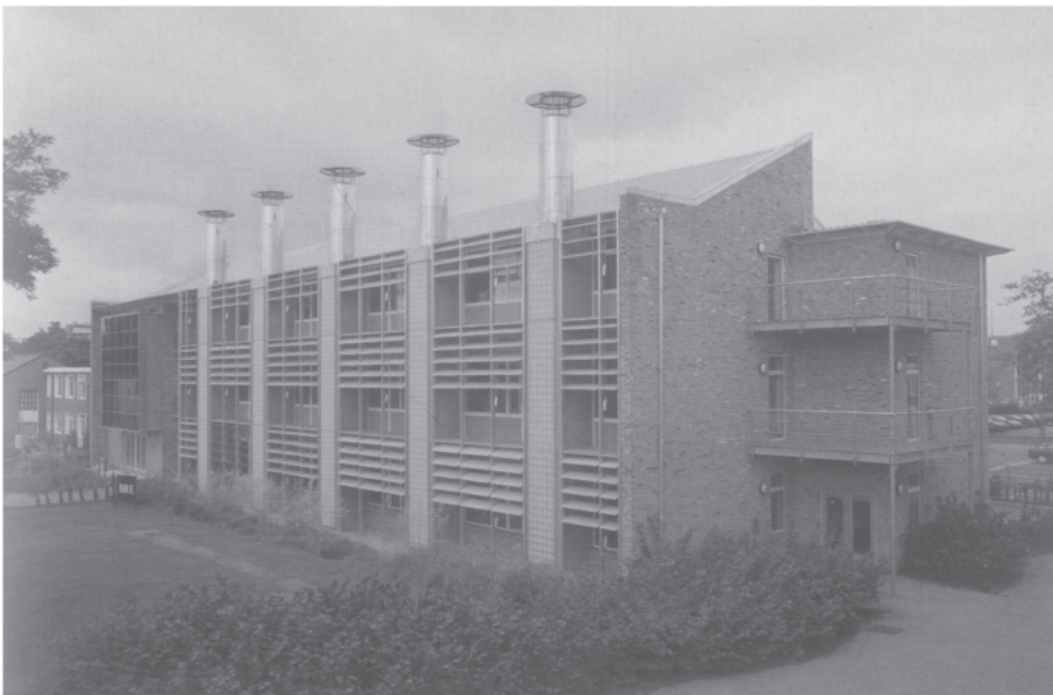
3.42 The BRE Environmental Building, Watford—south façade with its five glass block-clad ventilation stacks.
