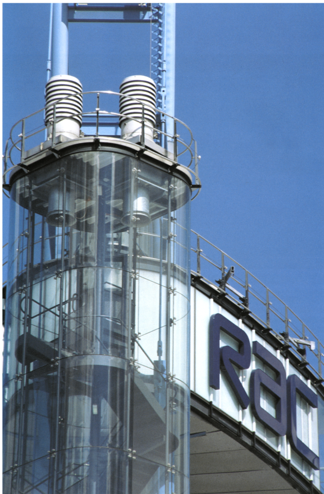
Plate 13 RAC Regional Centre, Bristol—customer visitor room and the top of the tower with its twin exhausts designed to provide smoke extraction.
