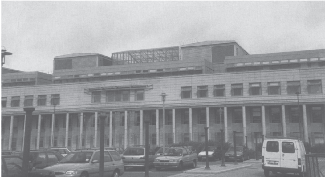
9.4 Eastward end of the south elevation. Note the colonnade, the glazing and shading of the upper floors, and the top of one of the atria flanked by two of the plant rooms.
