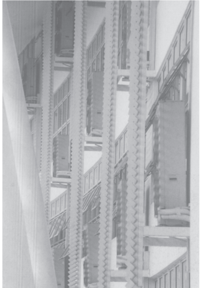
4.12 Banks of condenser units stacked behind their louvred screens.
