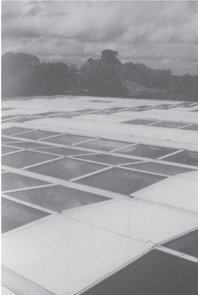
3.12 Menil Museum—roofscape. Note the white detachable external panels used to obtain additional light control.
