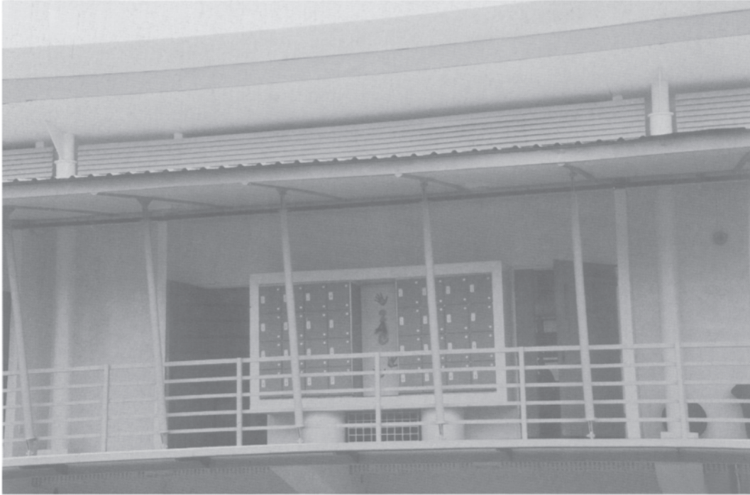
4.6 View towards the inner façade of a classroom. Note the louvred ventilation opening at high level and the grilled one below the lockers.
