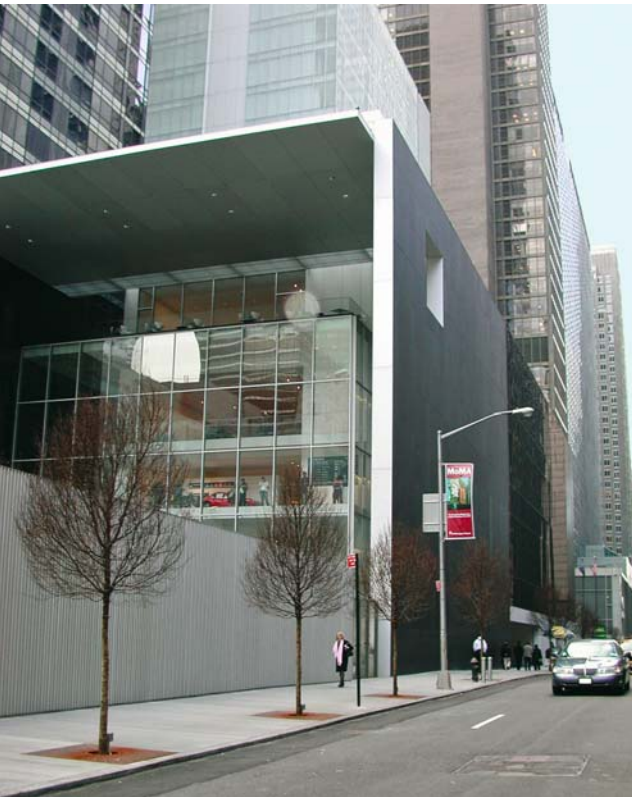
The MOMA expansion in New York City brought large concentrated loads on the garden pavers. The result was broken paving blocks.
