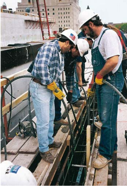
Extensive vibration is required during pours to remove air pockets that can lead to surface defects. Pulitzer Foundation, St. Louis.
