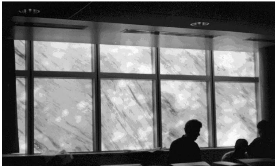
right Translucent stone façade allows light into the building. E.N.S.A.D., Paris, 1997
