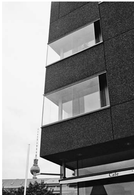
above and right Exposed aggregate in precast concrete panels, Headquarters of Sozialverband Deutschland, Léon Wohlhage Wernik Architekten, Berlin, 2003.
