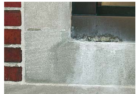
above Aluminum will corrode if in contact with wet concrete.
