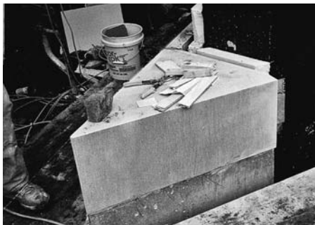
Because the corner is exposed to the gorillas and keepers at grade level, the durable corner was fabricated as a solid unit and beveled to resist chipping. Regenstein Center for African Apes, 2004, Chicago.
