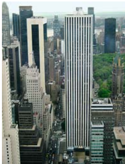
General Motors Building, New York City, 1968. Clad with white marble, with no signs of thermal hysteresis.
