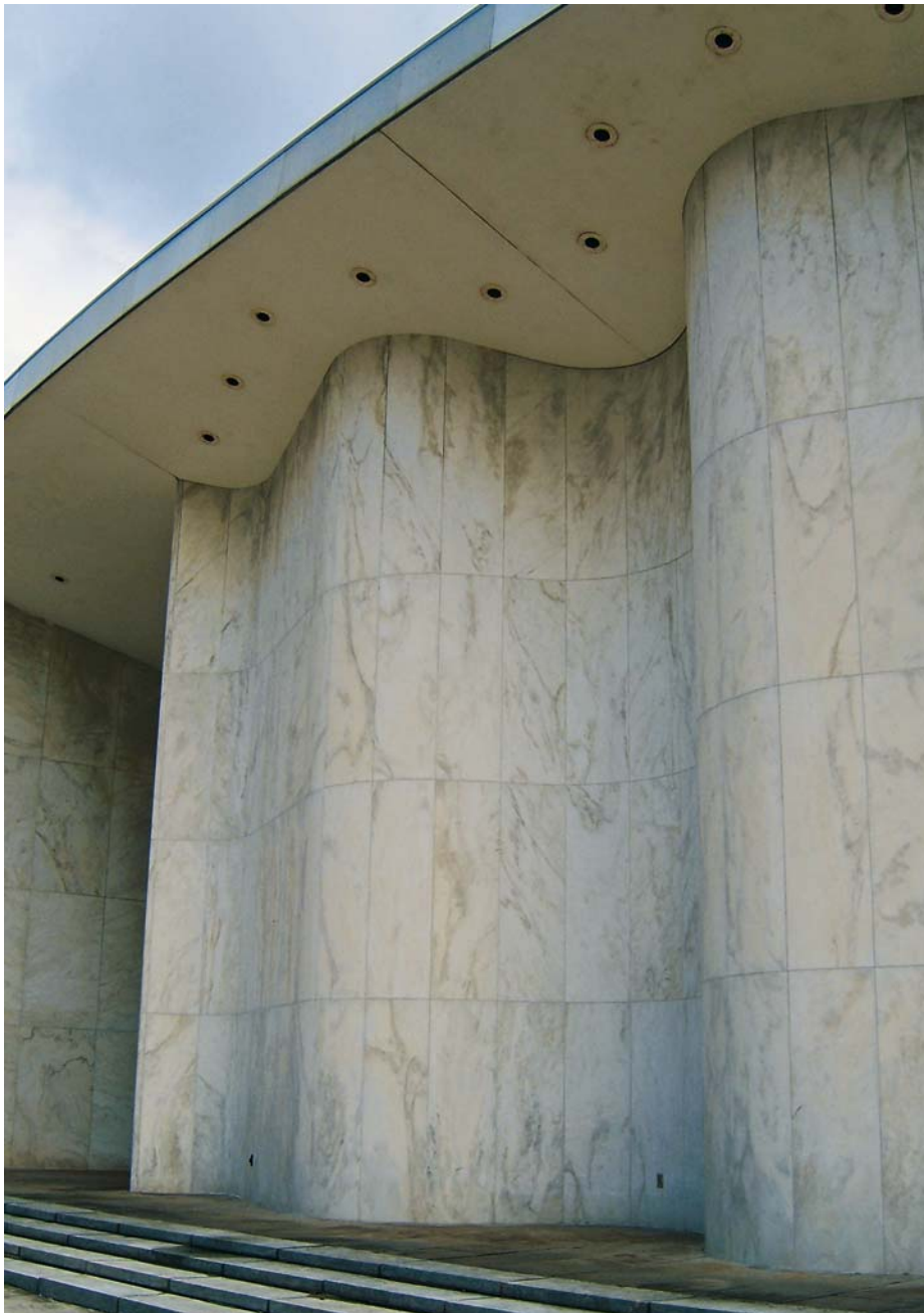
The top portion of the undulating stone façade has marks from a soffit that does not drip water away from the façade. Hall Auditorium at Oberlin College.
