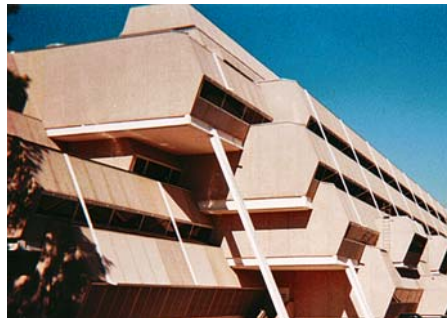
Burroughs Wellcome Headquarters, Research Triangle Park, North Carolina, 1972. Exterior wall and original test mock-up.
