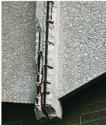
above Aluminum will corrode if in contact with wet concrete.
