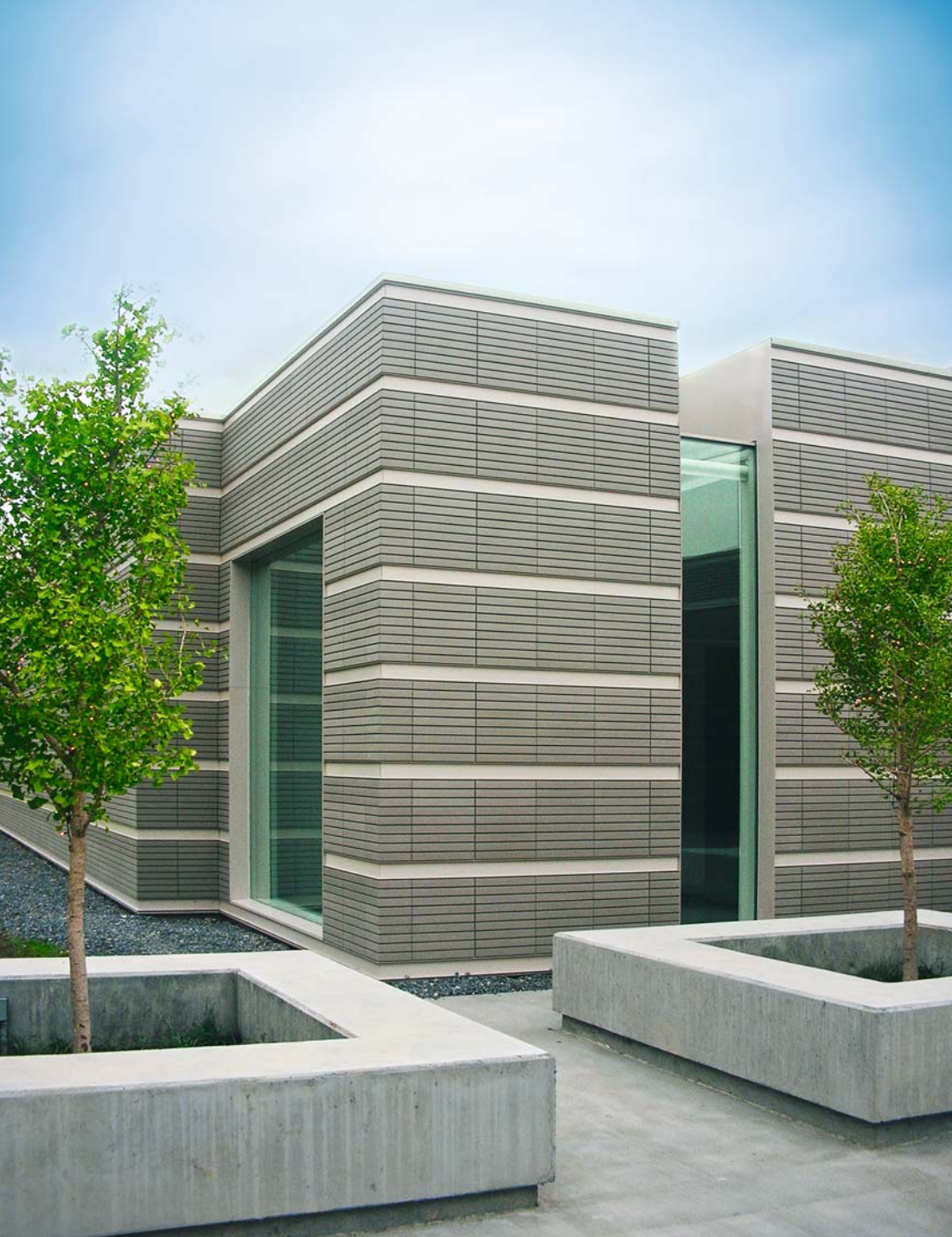
Terra-cotta panel façade, designed by Goettsch Partners, Hessel Museum, CCS Bard College, New York, 2006.
