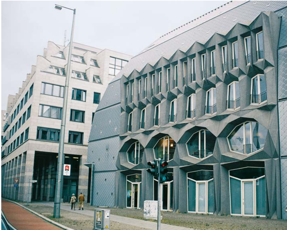
The headquarters of the Berlin Water Works, House III, 2003.
