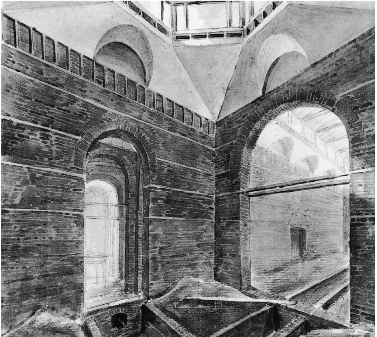
1.7 Dulwich Picture Gallery, view under construction showing the heating duct
