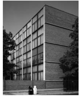
4.3 Glazed and brick façades viewed from the west
