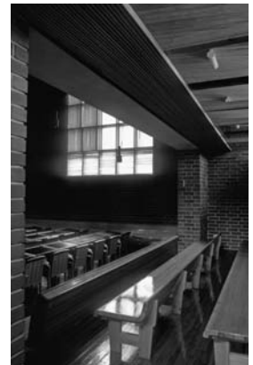
3.34 Detail of the Council Chamber seating. The relationship of seat and radiator is shown in the cross-section.
