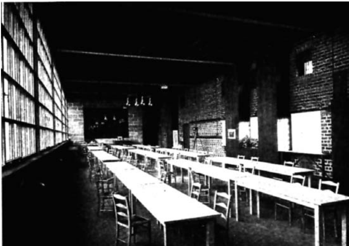
1.21 Glasgow School of Art. Second Floor Studio showing electric lighting, cast iron radiators beneath the windows and the timber cased air ducts on the inner wall.
