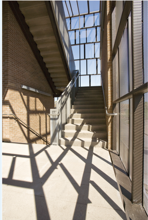
Figure 11-9 New egress stair Photo by Bill Timmerman
