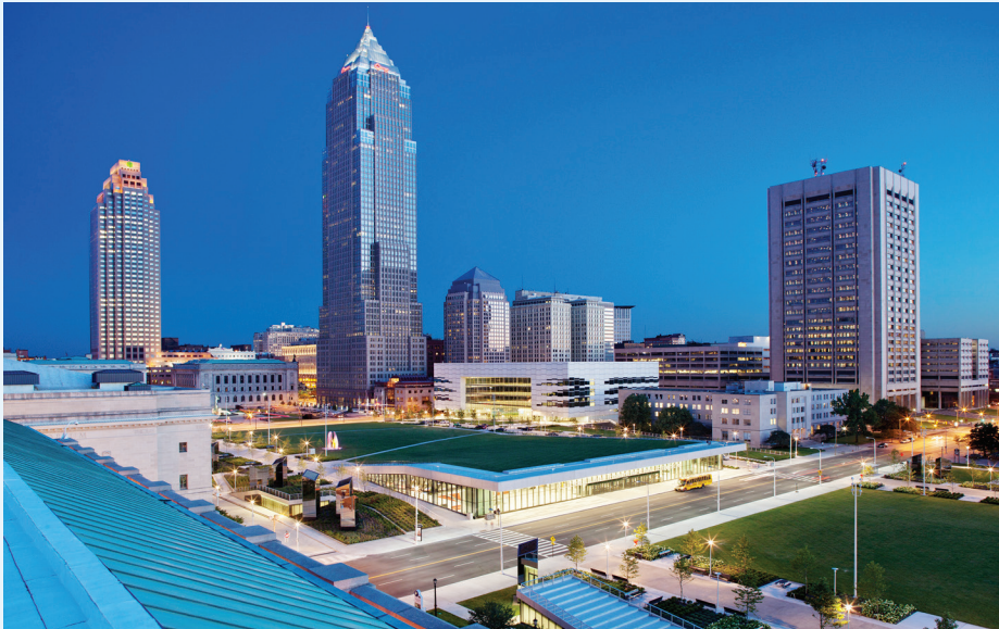
Figure 6-5 View from Lakeside and East Mall Allee, showing convention center entry and Burnham Mall in foreground © LaCasse Photography
