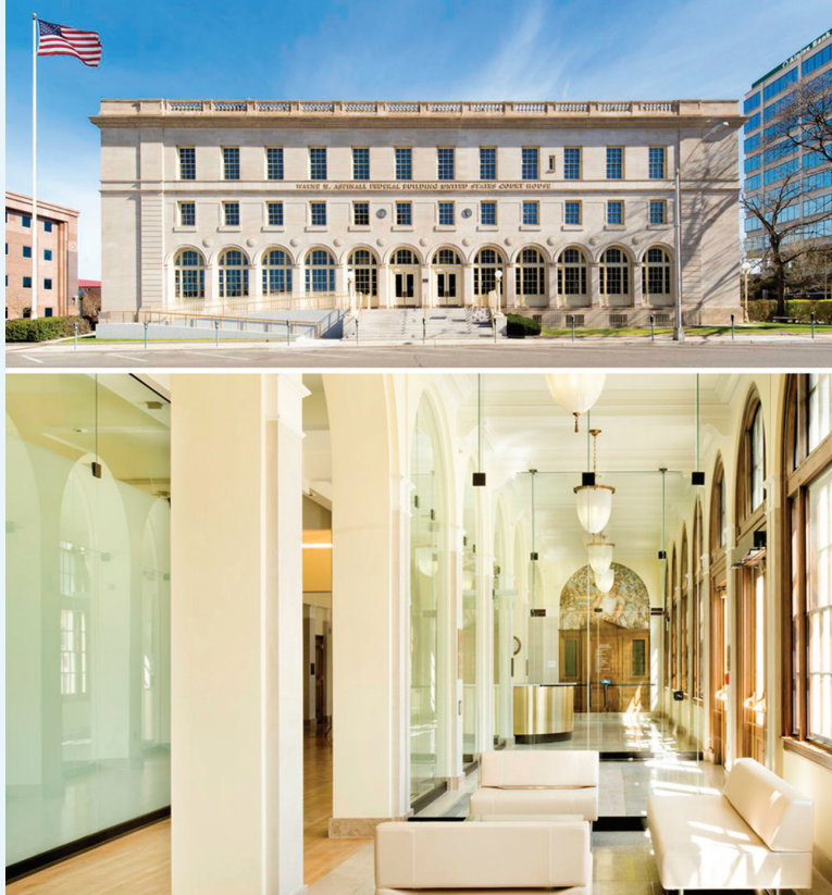
Figure 2-9 Aspinall building post-renovation Photography by Kevin G. Reeves; Courtesy of DLR Group
