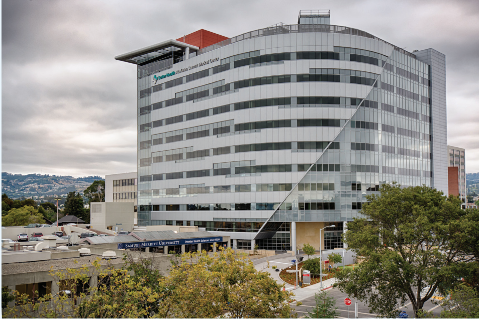
Figure 8-12 Alta Bates Summit Medical Center new patient care tower Image courtesy of Devenney Group Ltd., Architects
