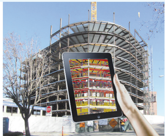
Figure 8-17 Field verification of digital model Image courtesy of Devenney Group Ltd., Architects
