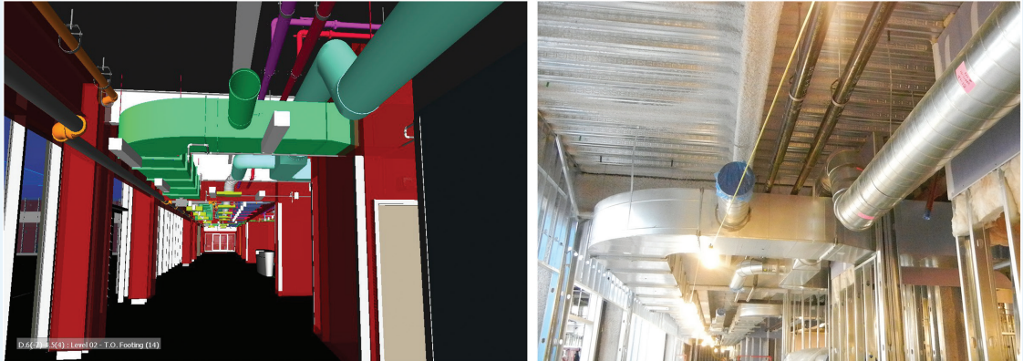
Figure 7-11 Comparison of model and installed assembly Image courtesy of CannonDesign
