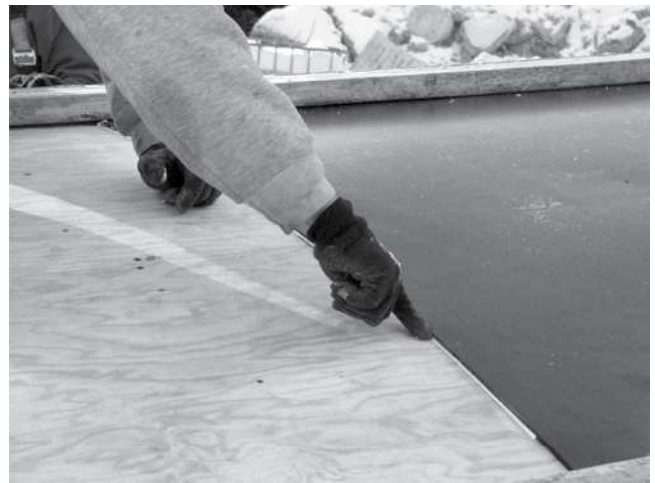
Fig. 5.5.1—Form joints sealed to prevent leakage.
