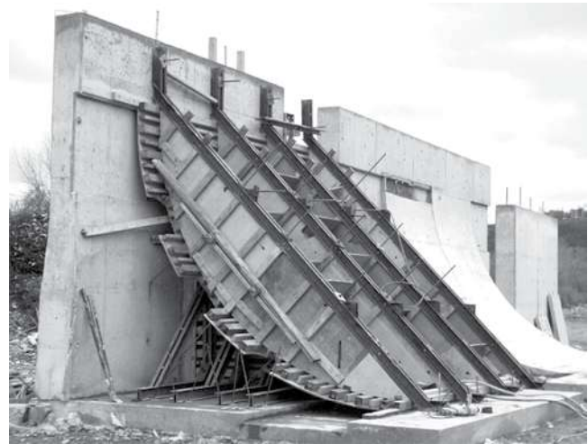
Fig. 3.5.4.a—Full-scale preconstruction mockup used for the Contemporary Arts Center, Cincinnati, OH.
