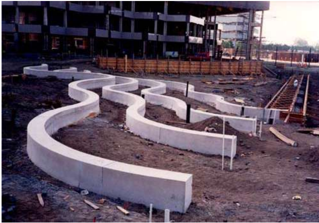
Fig. A.17—Planter walls (Shaw & Sons, Costa Mesa, CA).
