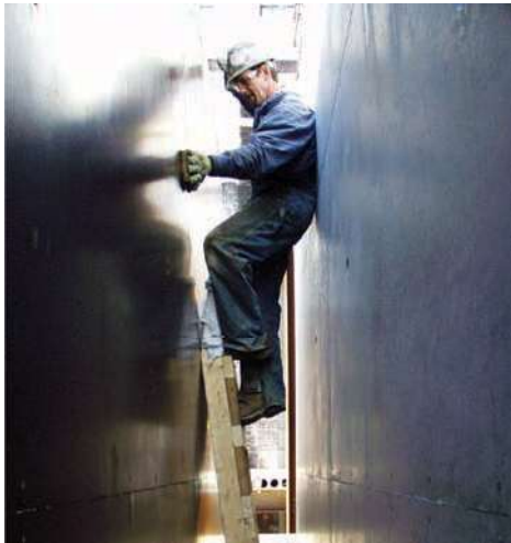
Fig. 5.9.6—Release agent applied after form erection.
