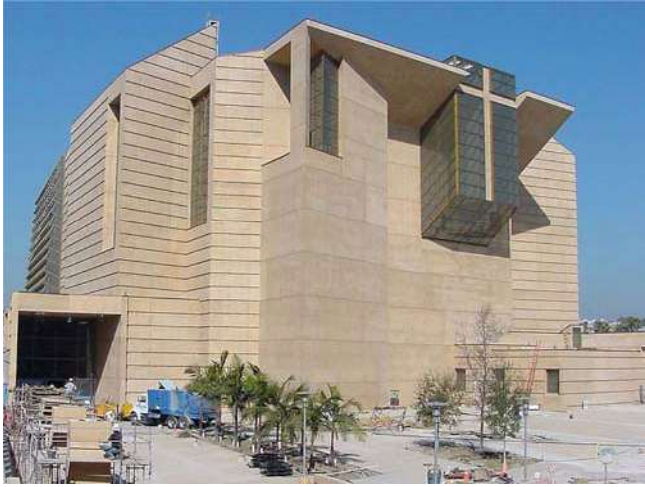
Fig. A.1—Cathedral of Our Lady of the Angels, Los Angeles, CA. (Morley Construction Co., Santa Monica, CA).
