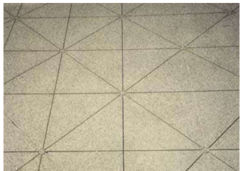
Fig. A.22—Architectural sawcut (Shaw & Sons, Costa Mesa, CA).
