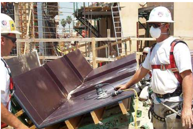
Fig. A.19—Bondo and sanding to prepare formwork for use.
