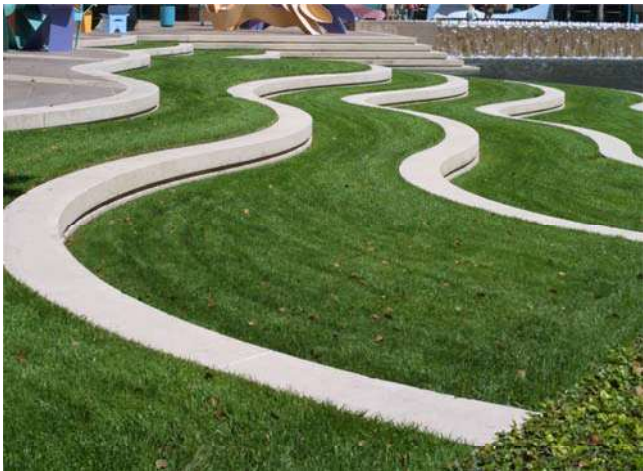
Fig. A.18—Planter walls (completed) (Shaw & Sons, Costa Mesa, CA).
