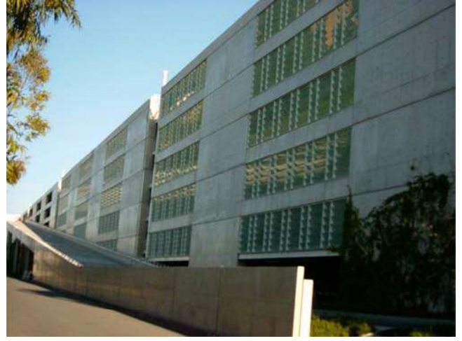
Fig. A.4—Disneyland Parking Structure.
