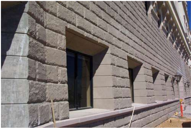
Fig. A.12—Form liner finish and tapered openings.
