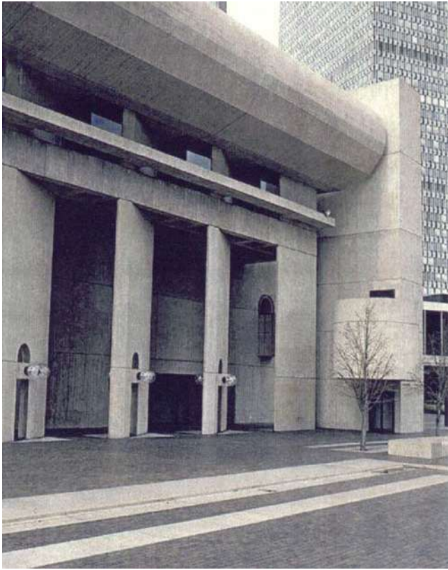
Fig. A.7—Christian Science Plaza; Colonnade Building featuring sun shade columns.
