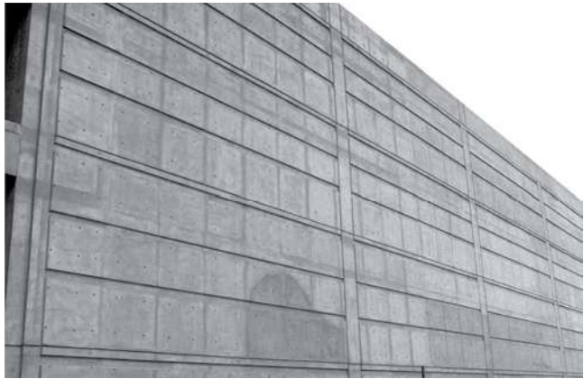
Fig. 4.4—Rustication strips used to break up a large expanse of concrete.
