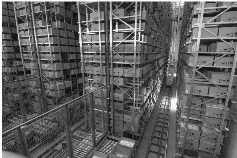
Figure 1.13 AS/RS (Source: Courtesy of Vanderlande Industries)
