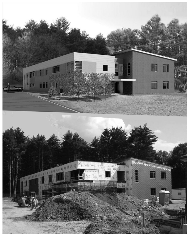
Figure 2.26 Needham PSAB entry perspective—rendering (top) and during construction (bottom). © Winter Street Architects
