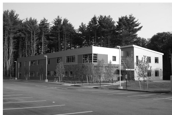
Figure 2.27 Needham PSAB completed project. © Winter Street Architects
