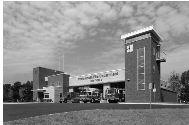
Figure 2.28 Portsmouth Fire Department Station 2, completed project. © Winter Street Architects © Damianos Photography
