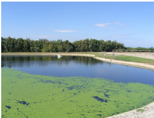
FIGURE 6 Picture showing a typical polishing pond located in the northeast Spain. Lemna sp. proliferation can be observed.
