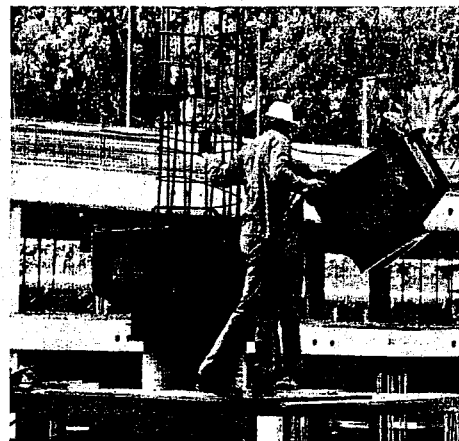
(b) Capital forms lifted by crane
