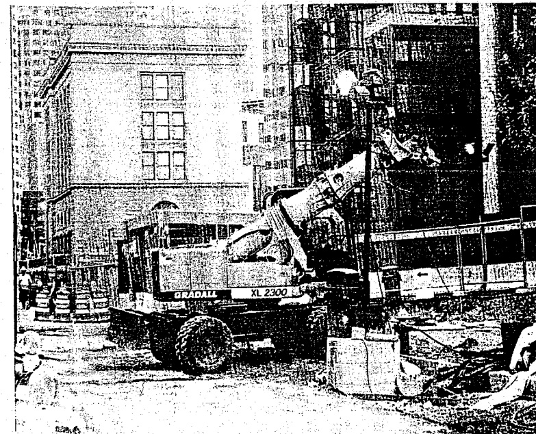
FIGURE 11.10 Gradall working on a city street project.
