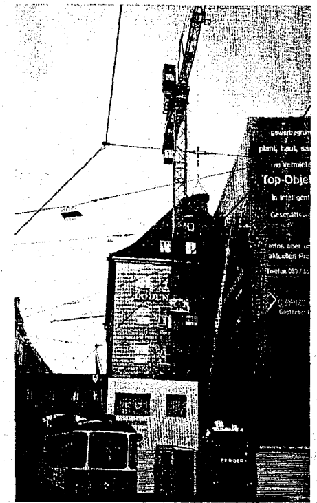
FIGURE 21.22 Enclosure around a building project.
