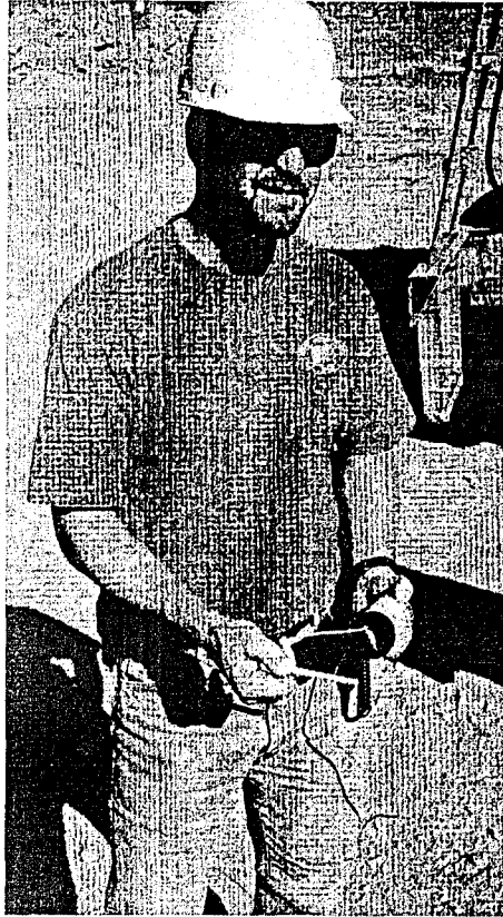
FIGURE 13.4 Placing an electric detonator in a booster.
