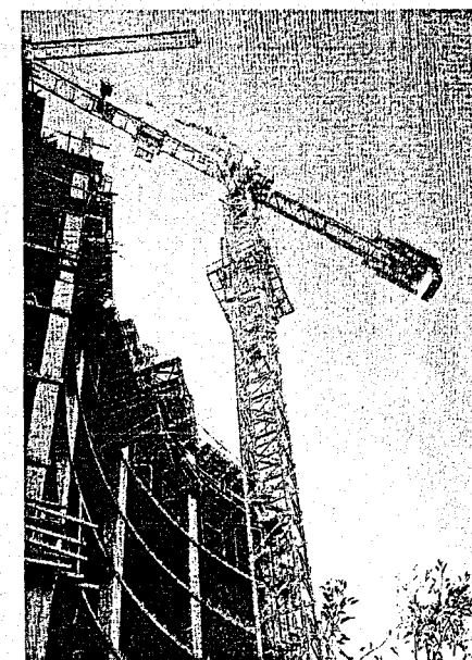
FIGURE 22.18 Table form being removed by a crane located near the façade of the building.
