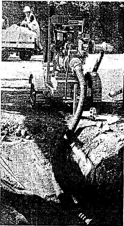
FIGURE 20.6 Wheel-mounted centrifugal pump.
