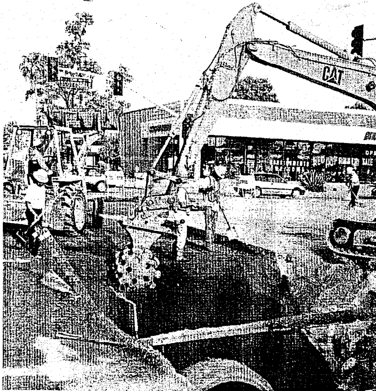
FIGURE 5.11 Compaction wheel mounted on a hydraulic excavator boom.
