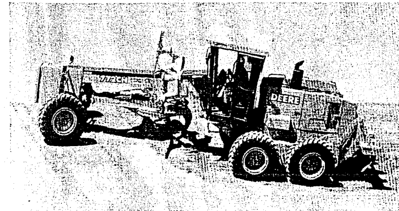
FIGURE 11.2 Grader working a slope.
