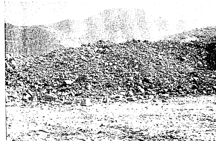
FIGURE 13.2 The result of a blast on a dam project.
