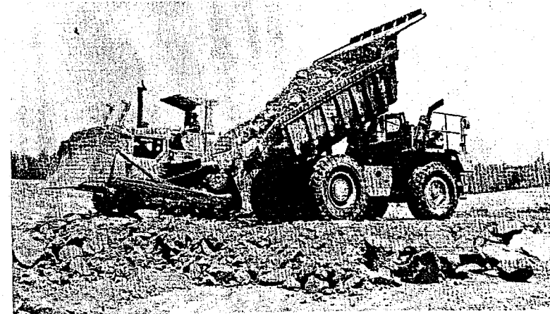
FIGURE 3.18 Spreading dumped embankment material with a dozer.
