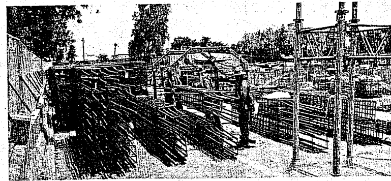
FIGURE 21.5 Reinforcing steel cages being tied at the project site.
