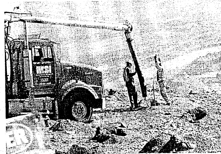
FIGURE 13.3 Loading bulk ANFO into blastholes.
