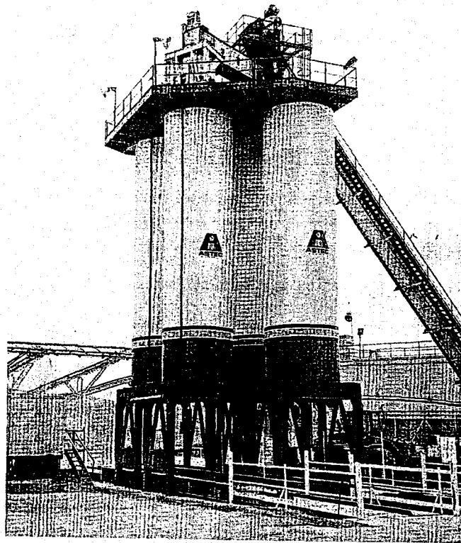
FIGURE 15.14 Storage silos at a drum mix asphalt plant.
