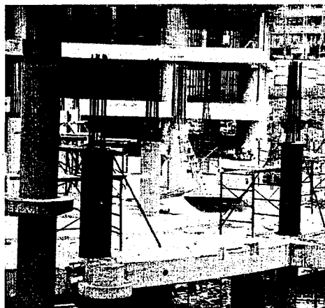
(a) Forms and finished columns
