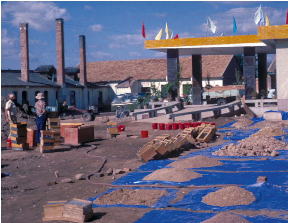
Fig. 1.4 Screening operation at the Yushe Hotel, showing tandem screen boxes, drying tarps for discrete samples, buckets to soak the dried sediment in water, and wash tubs in which the boxes are agitated (Photo by L. Flynn, Sept. 1987)
