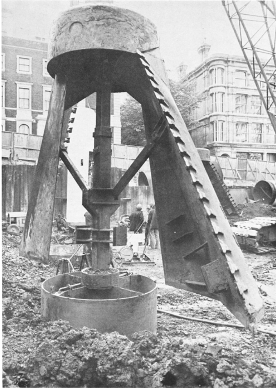
Fig. 3.30 Top-hinged under-reaming bucket
