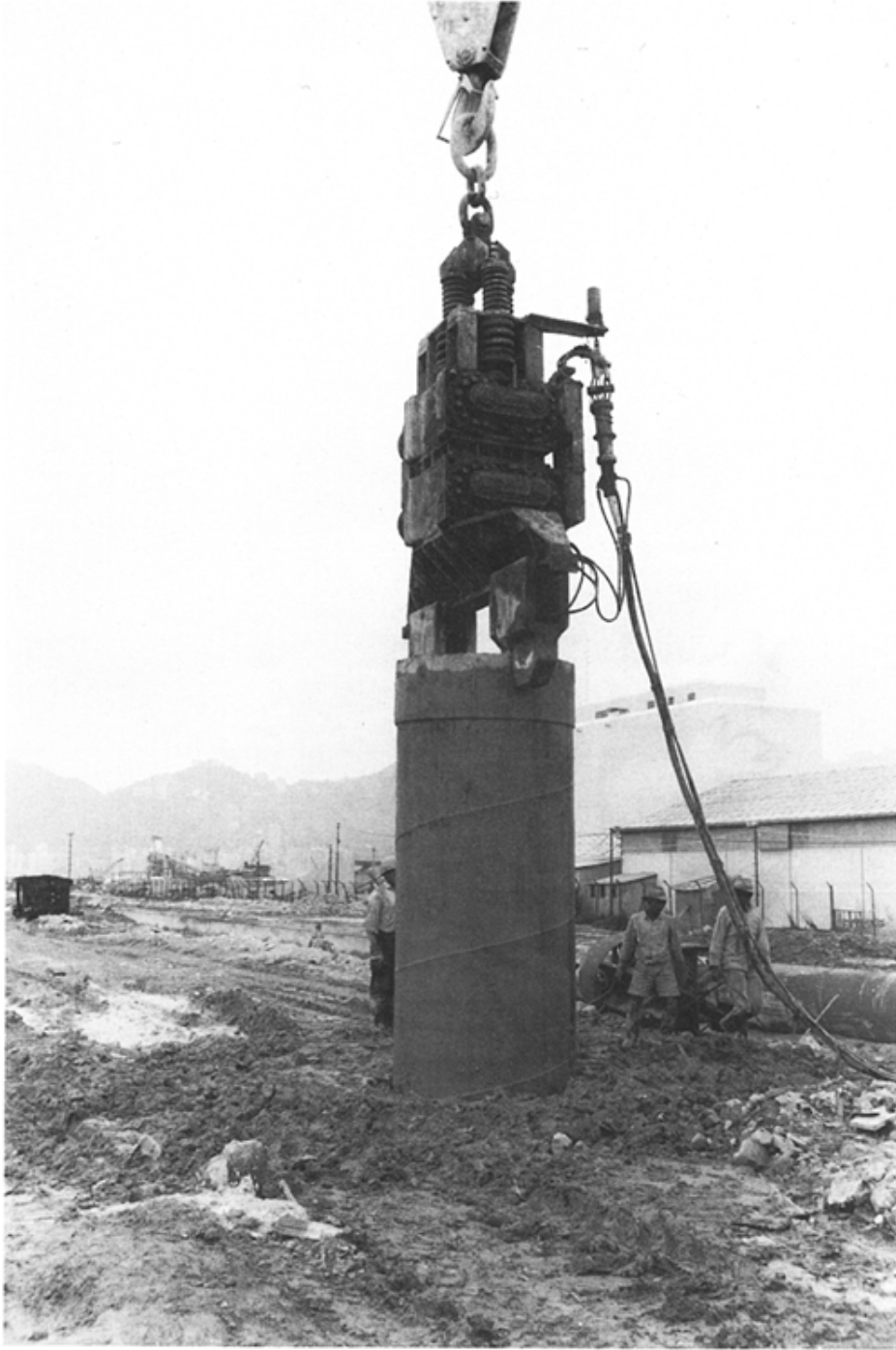
Fig. 3.17 Driving pile casing with Muller vibrator.
