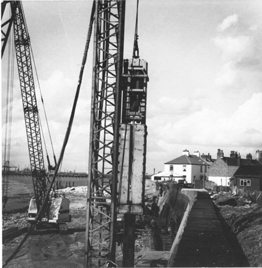
Fig. 3.14 BSP International Foundations Ltd. hydraulic piling hammer
