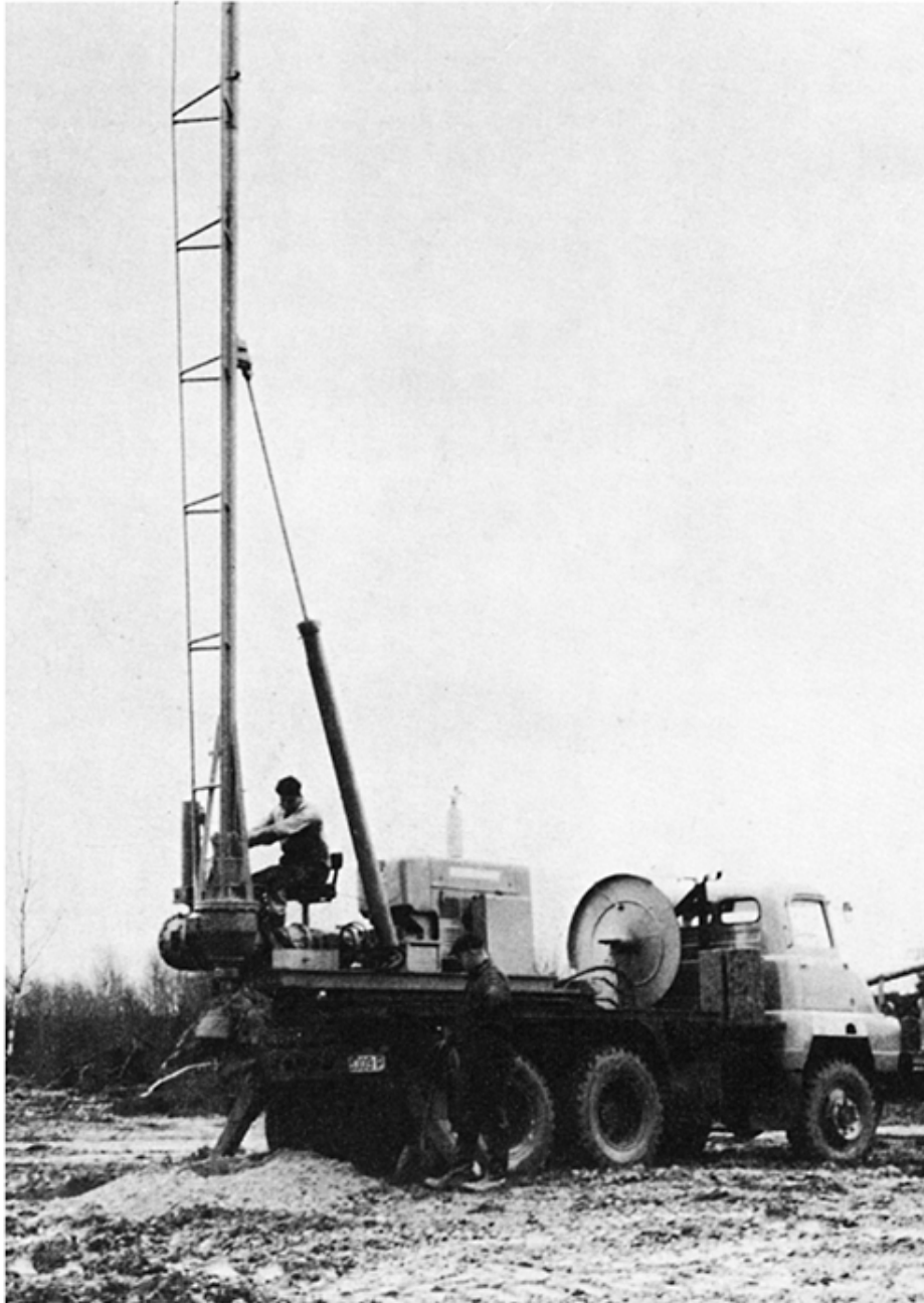
Fig. 3.26 'Highway' lorry-mounted auger drill
