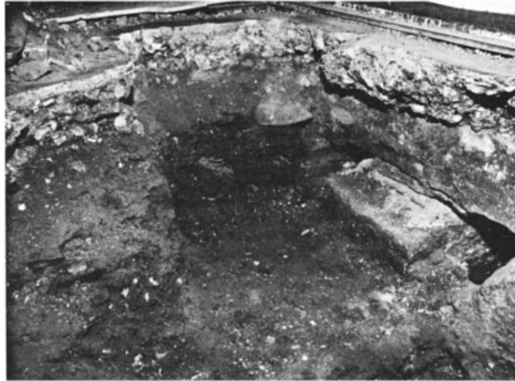
(a) Cavities left by complete decay of piles and timber capping sills
