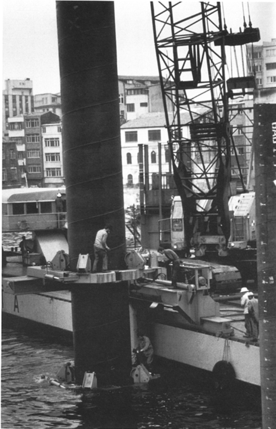
Fig. 3.8 Barge-mounted pile guides with hydraulically-operated clamps
