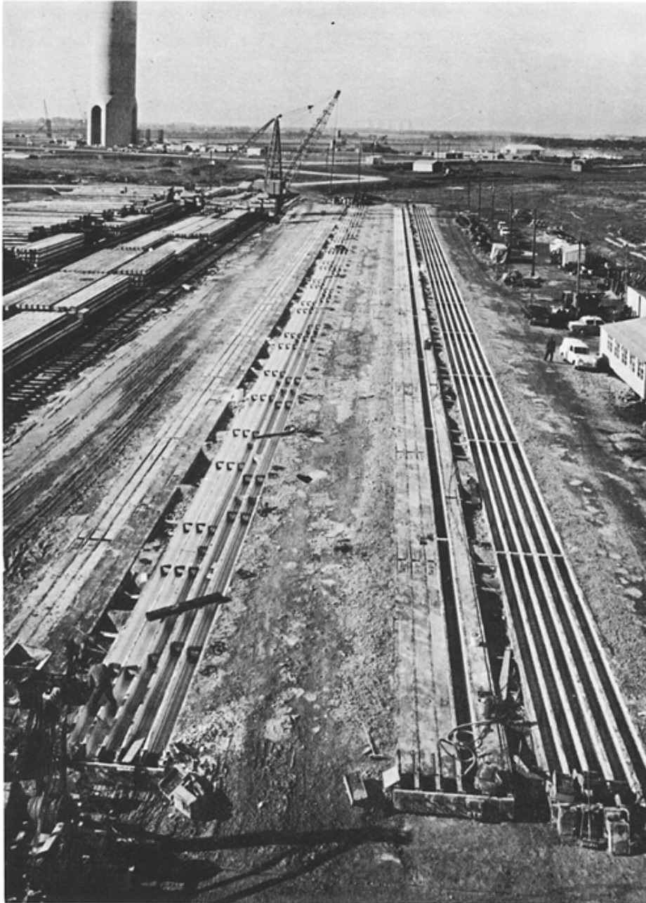
Fig. 2.11 Casting yard for prestressed concrete piles at Drax Power Station
