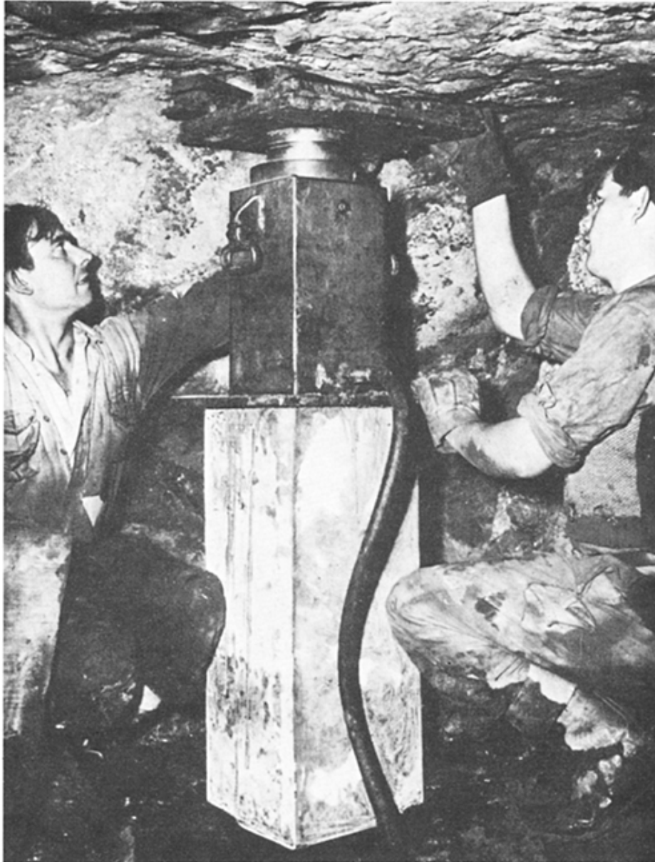
Fig. 9.6 Jacking down Franki Miga pile
