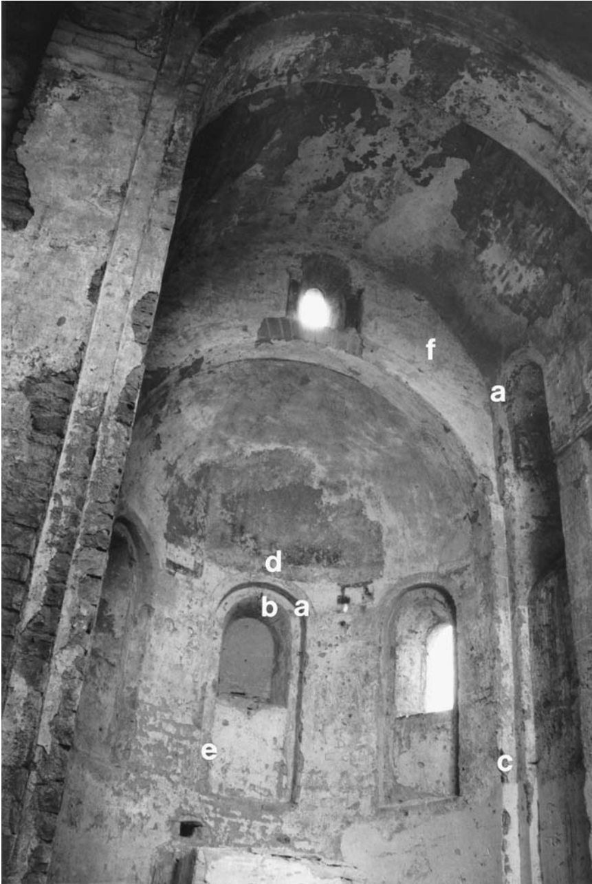
122. Saint-Hippolyte, priory church, interior, choir and apse; (a) reveal in arcade around window; (b) face of window voussoirs; (c) reveal on side of apse; (d) half dome; (e) panel beneath window; (f) vertical plane above apse reveal.
