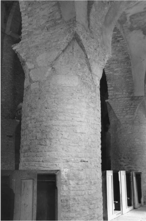
39. Chapaize, Saint-Martin, interior, nave, southern aisle, third freestanding pier.
