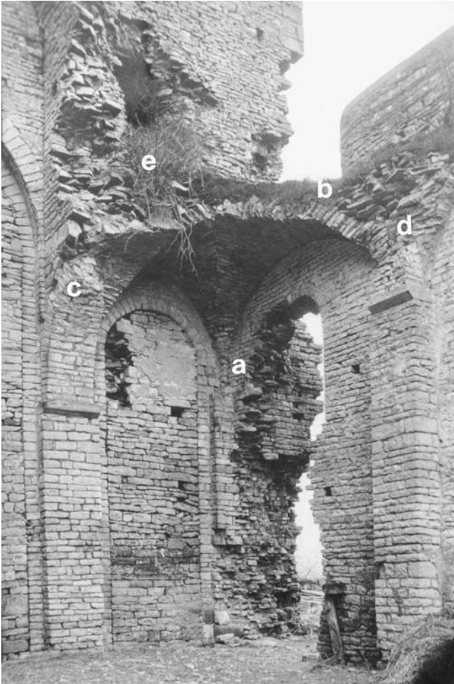
118. Saint-Hippolyte, priory church, interior, nave, southern aisle (author's detail photograph from restoration file, Caisse Nationale des Monuments Historiques); ( a ) narrow extended base beneath corbeled portion of vault; ( b ) flattened web top; ( c ) thin spandrels covering high and flat springing of vault; ( d ) horizontally coursed stones in corbel vault; ( e ) outside face of wall at base of second story.
