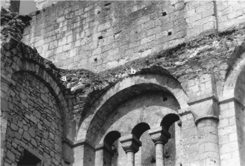
22. Jumièges, Notre-Dame, nave, southern aisle, tribune, groin vault; cross section showing coursed stones in corbel, (a) radially laid stones in true vault, and (b) semicircular webs.
