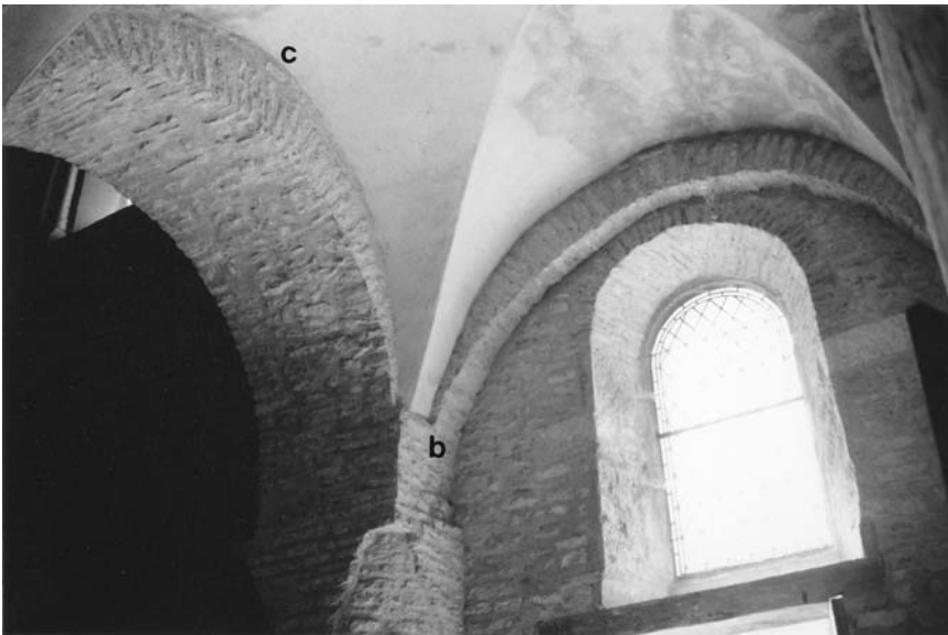
37. Chapaize, Saint-Martin, interior, nave, northern aisle, western bay, formeret , arcade, and groin web; (b) courshed stones between web and formeret ; (c) pointed groin web and horizontally laid stones in the shape of brick above extrados of the arch.
