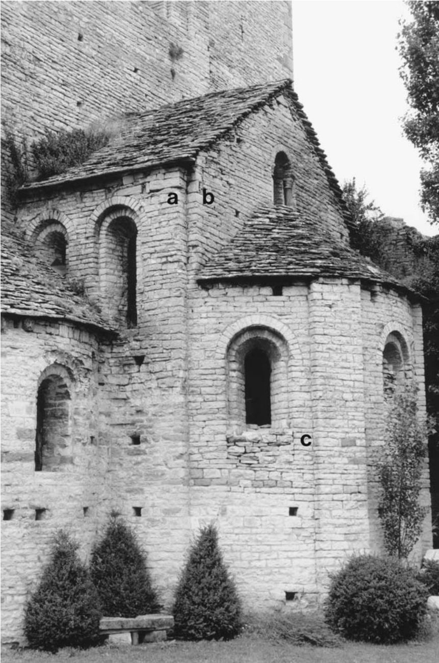
121. Saint-Hippolyte, priory church, exterior, chevet; (a) reveal on side wall of choir; (b) reveal on eastern wall of choir; (c) band on apse.
