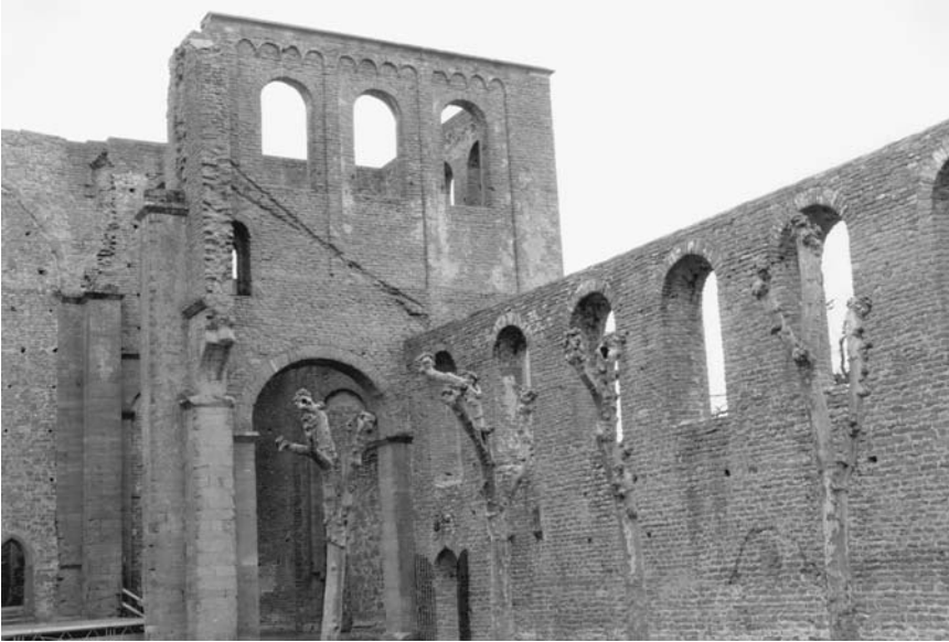
81. Limburg an der Haardt, abbey church, nave, crossing and transept, with ashlar piers and Lombard corbel tables.
