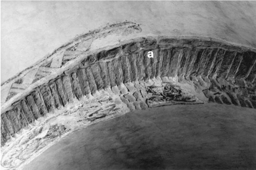
34. Tournus, Saint-Philibert, interior, lower narthex, central bay, detail of southern arcade; (a) stones in the shape of bricks, placed horizontally between the extrados of the arcade and the web of the groin vault.
