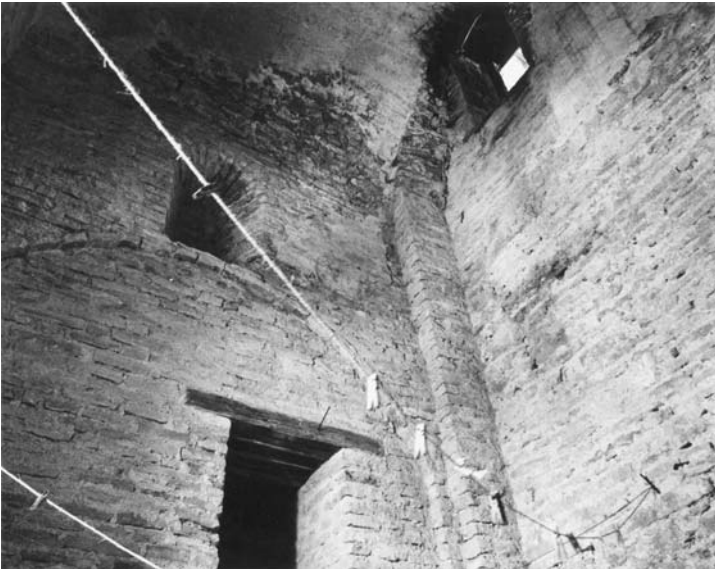
86. Châtillon-sur-Seine, Saint-Vorles, interior, westwork, upper story, wall arch.
