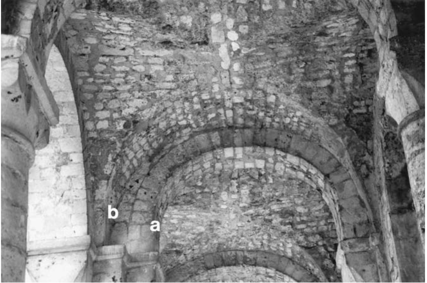
23. Jumièges, Notre-Dame, nave, interior, northern aisle, groin vault, with (a) stilted transverse arch and (b) narrow wall at the springing.
