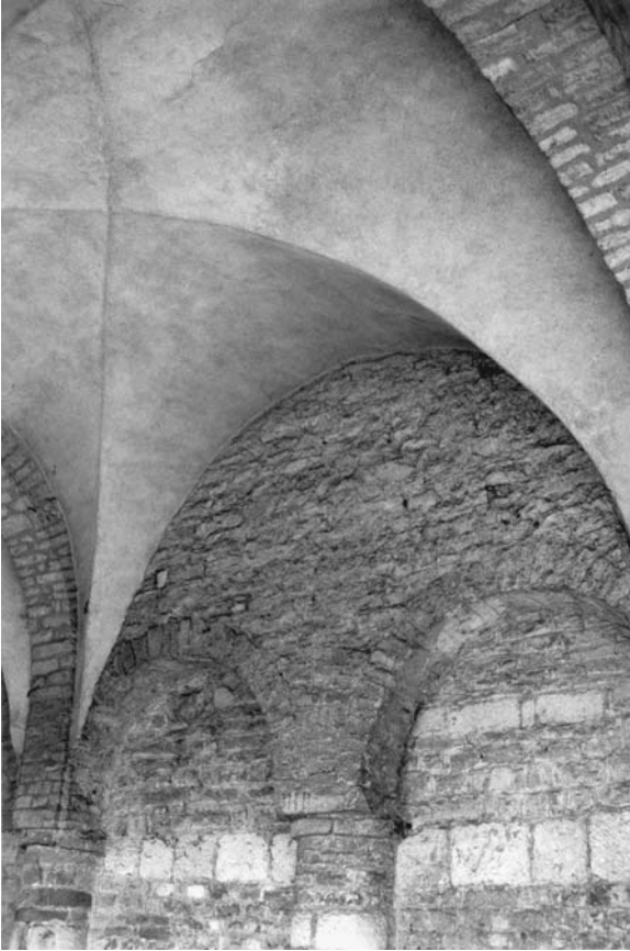
49. Tournus, Saint-Philibert, interior, cloister, northern wall, with pointed web.
