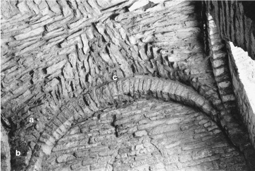
36. Chapaize, Saint-Martin, interior, nave, southern aisle, western bay, formeret and groin web; (a) corbel vault; (b) coursed stones between web and formeret ; (c) radial stones of true web rest above the extrados of formeret .
