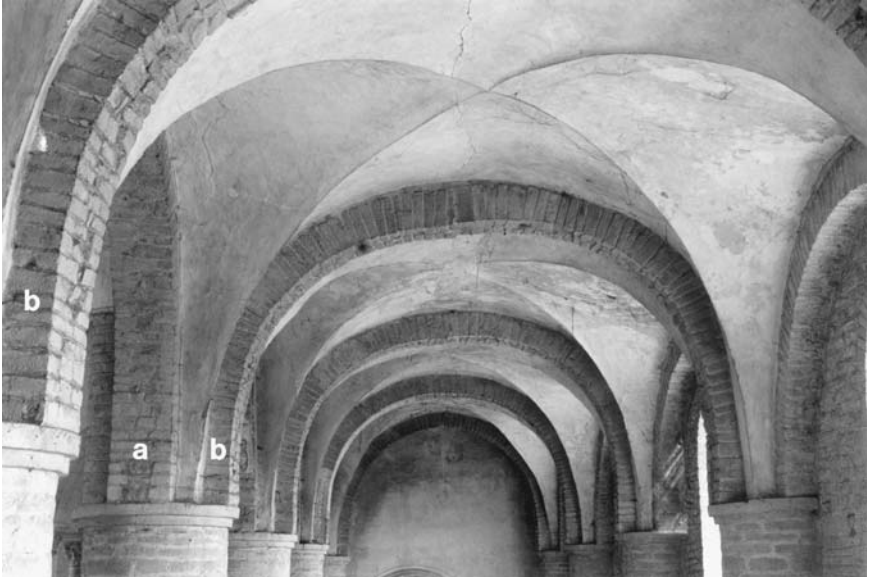
46. Tournus, Saint-Philibert, interior, nave, southern aisle, vaults; (a) stilted springing of arcade; (b) stilted springing of transverse arch.
