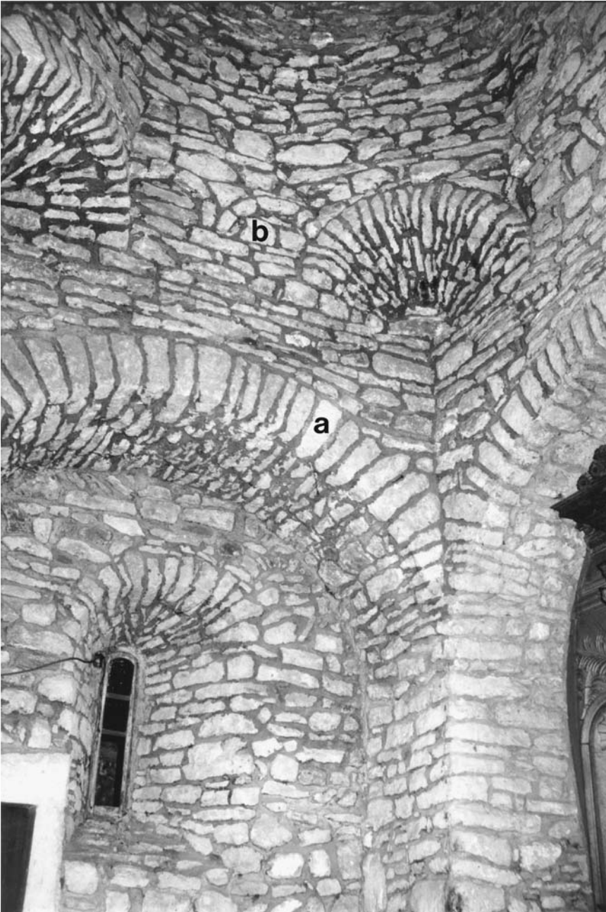
89. Bray, village church, interior, crossing; (a) wall arcade; (b) squinches and corbel table.
