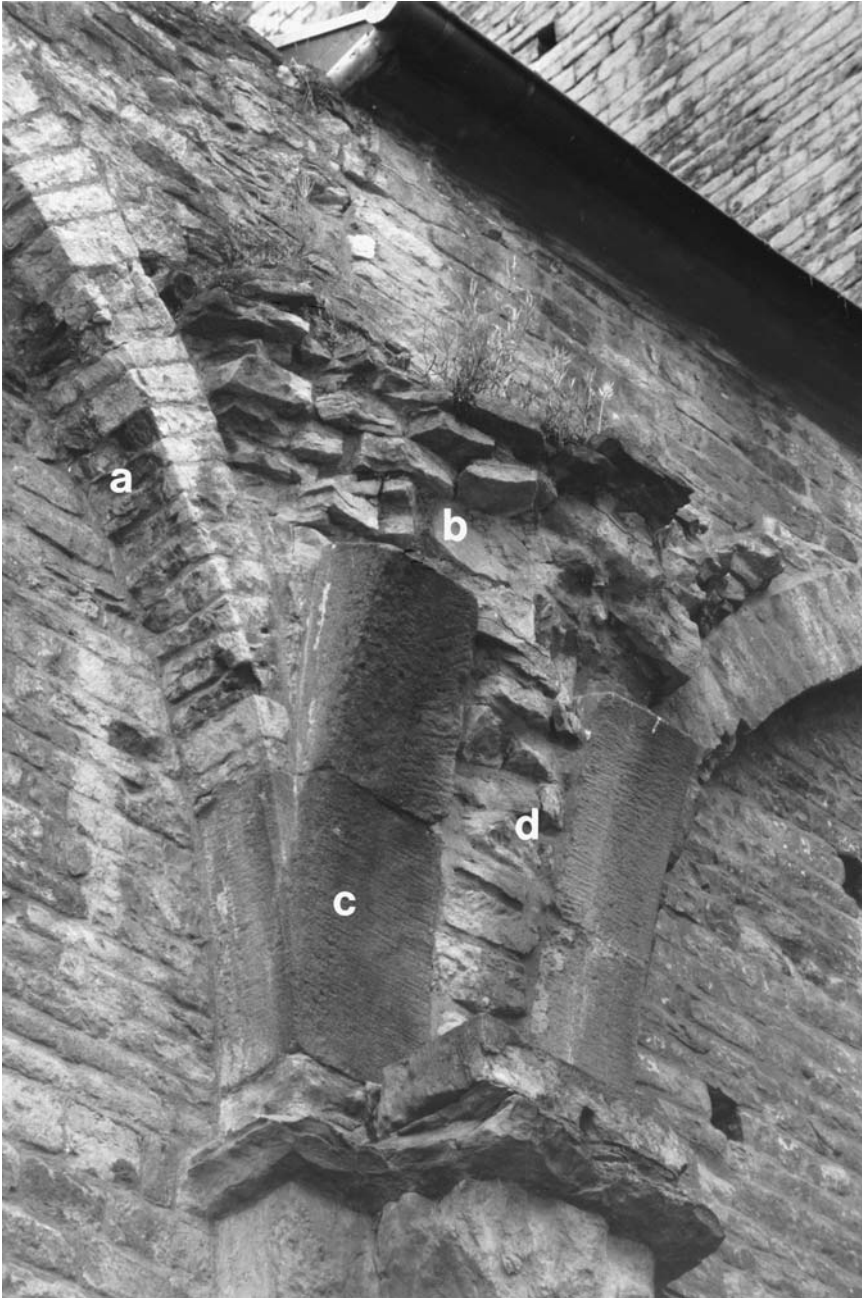
60. Cluny III, interior, choir, southern aisle, ruined central transverse arch and formerets (detail of Fig. 58); (a) brick-shaped formeret stones; (b) horizontally coursed stones in corbeled portion of groin vault; (c) ashlar tas-de-charge at base of formeret and transverse arch; (d) horizontally coursed brick-shaped stones in center of springing of transverse arch.
