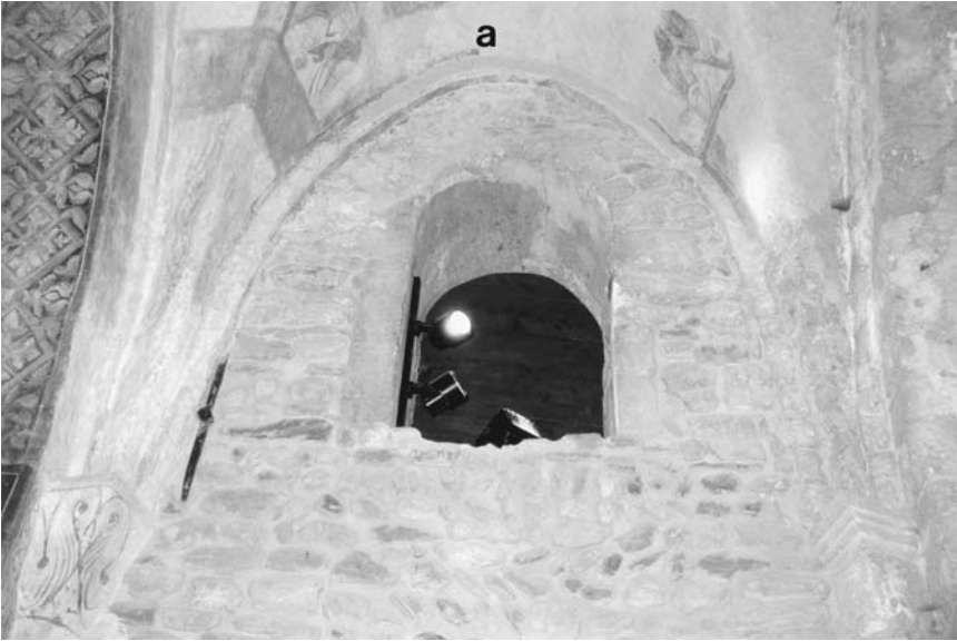
29. Aime, Saint-Martin, interior, choir, northern wall; (a) pointed web.
