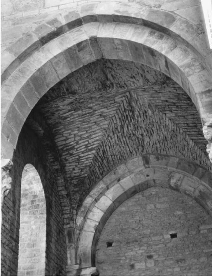
63. Cluny III, interior, nave, southern aisle, eastern bay, groin vault.
