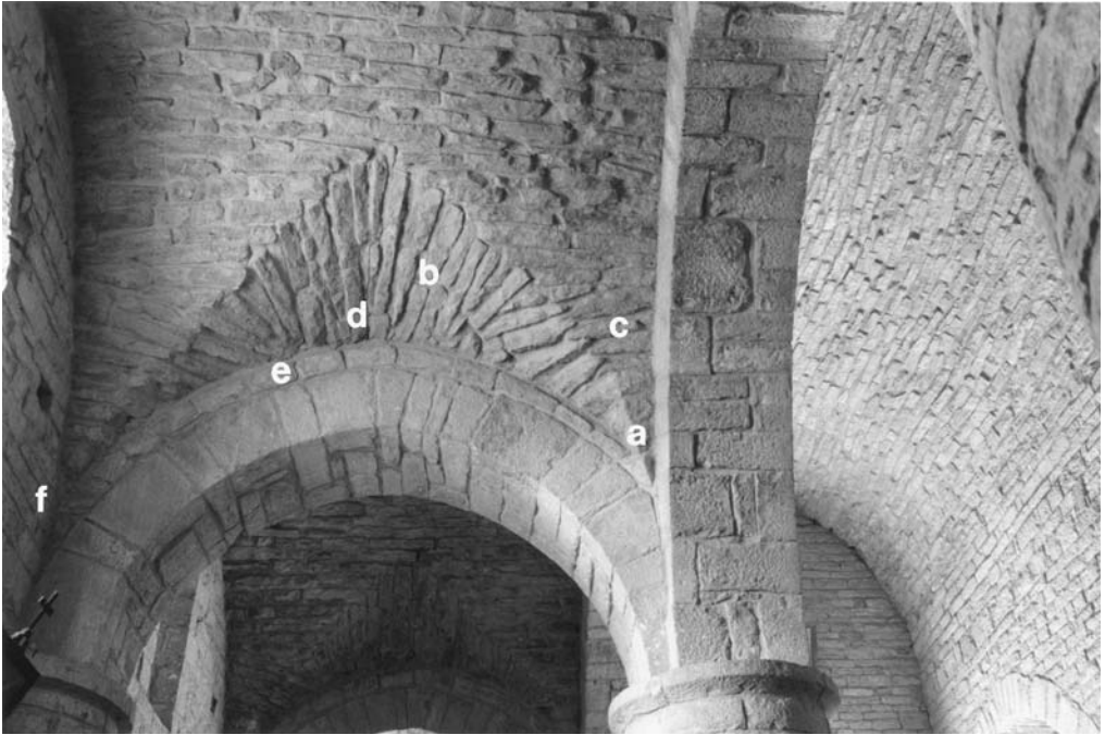
45. Farges, Saint-Barthélemy, interior, nave, southern aisle, third bay, detail of arcade, transverse arch, and broken barrel vault; (a) intersection of ashlar arcade and transverse arch; (b) radially laid brick-shaped stones of true vault; (c) coursed brick-shaped stones of corbel vault; (d) flattened web; (e) horizontally placed brick-shaped stones above the extrados of transverse arch; (f) low springing of outside web.
