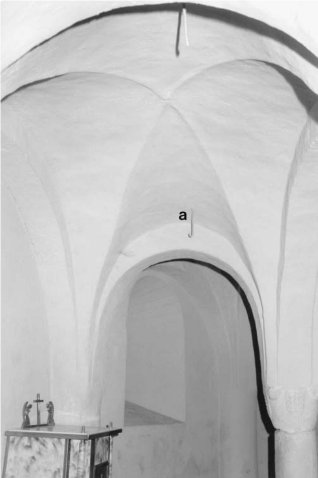
5. Agliate, San Pietro, interior, crypt, eastern end, central and southern aisles; (a) pointed web.
