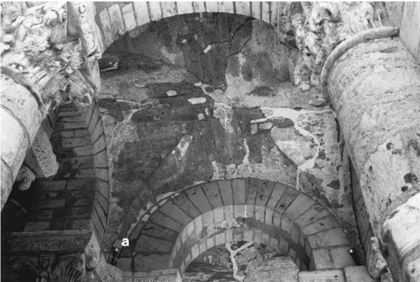
25. Saint-Benoît-sur-Loire, abbey church, interior, narthex, ground floor; (a) narrow wall of stones inserted next to springing of transverse arch.
