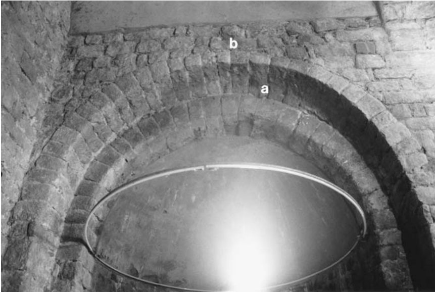
54. Sant Cugat de Salou, interior, transept, northern apse, arcade; (a) undercut voussoirs in center of arch; (b) narrow fascia of central voussoirs.
