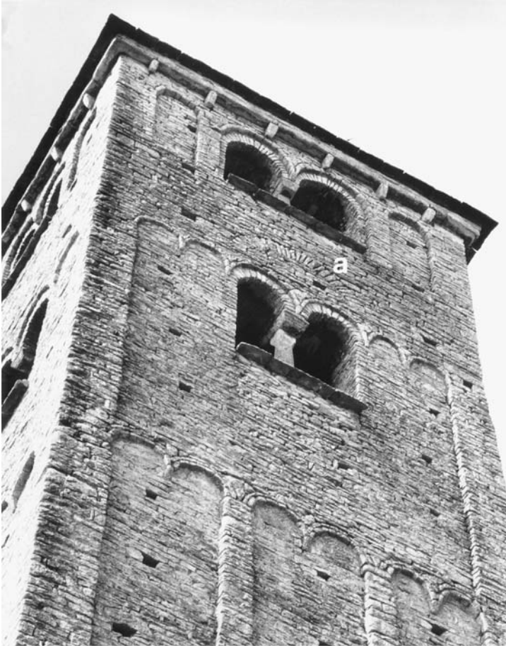
57. Chapaize, Saint-Martin, exterior, crossing tower; (a) relieving arch.
