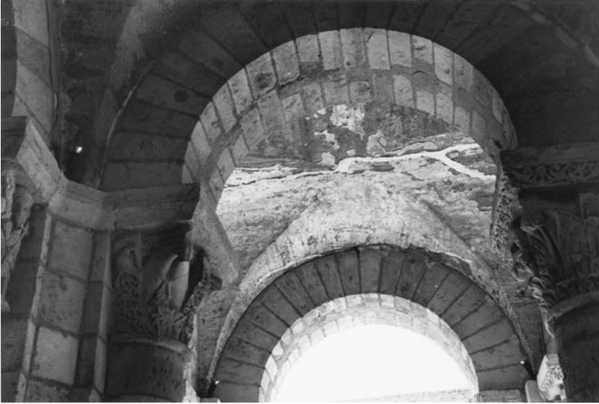
24. Saint-Benoît-sur-Loire, abbey church, interior, narthex, ground floor, groin vault with steeply corbeled base and short-segmented groins.
