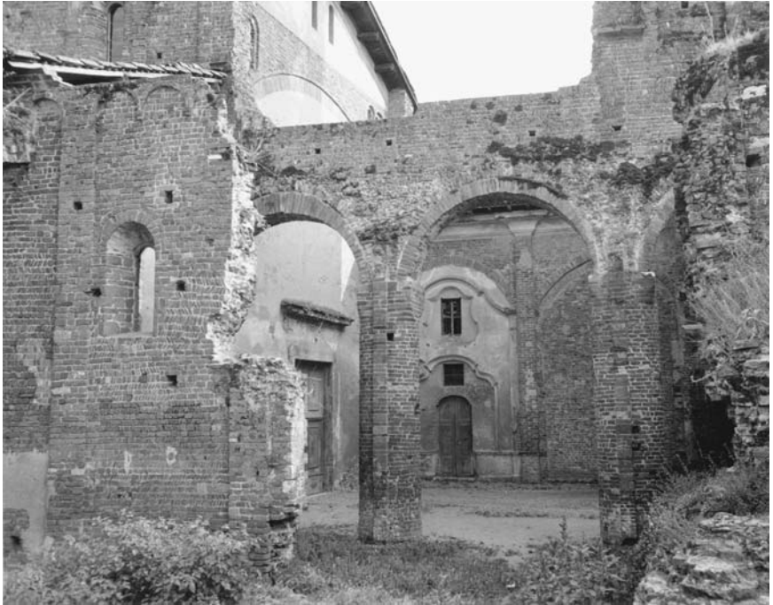
15. Lomello, Santa Maria Maggiore, nave, northern aisle, three western bays.
