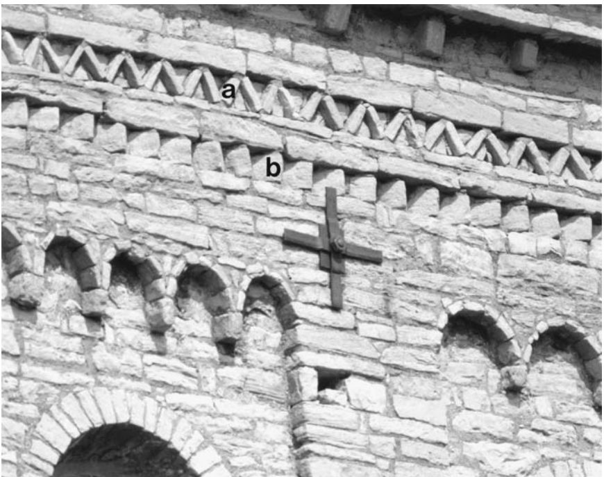
13. Tournus, Saint-Philibert, exterior, upper narthex, southern clerestory, stones shaped like brick placed in (a) diagonal and (b) projecting teeth patterns.
