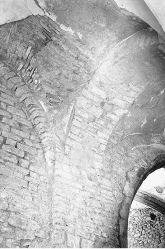
93. Saint-Martin-de-Laives, interior, nave, southern aisle, detail of formeret , transverse arch, and groin vault.
