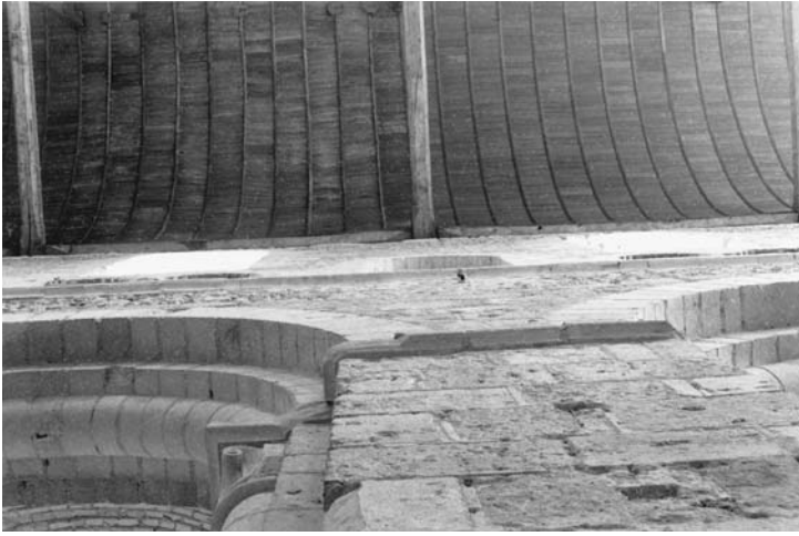
6. Bernay, Notre-Dame, interior, nave, southern elevation, string-courses between stories, column, capital, and impost.
