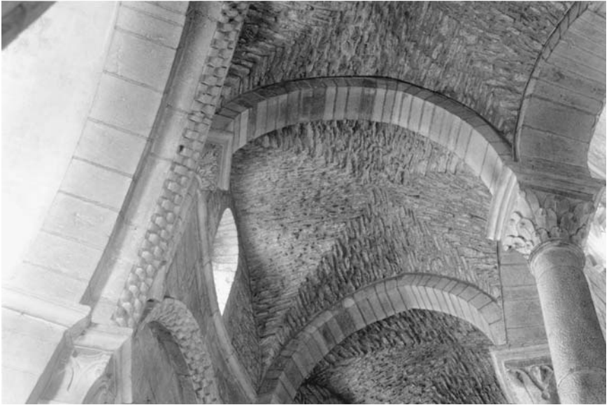
50. Paray-le-Monial, priory church, interior, ambulatory, vaults.
