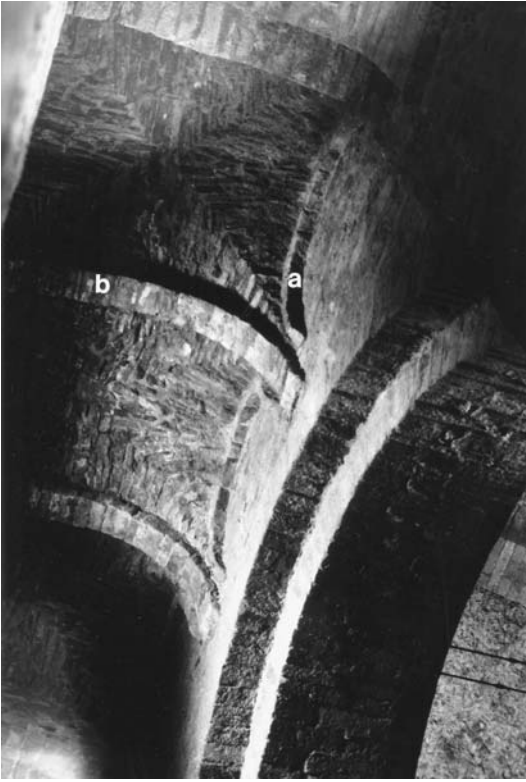
79. Cardona, Sant Vicenç, interior, nave, southern aisle; (a) formerets; (b) transverse arches.
