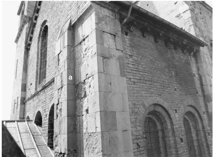
106. Cluny III, exterior, southern transept, southeast corner; (a) buttress extension.
