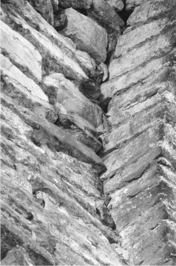
67. Tournus, Saint-Philibert, interior, upper narthex, first bay, northern wall, detail of transverse arch and barrel vault; corbel vault overlaps side of transverse arch.
