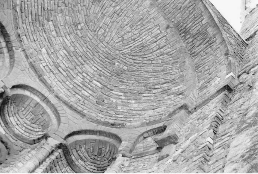
83. Ager, Sant Pere, interior, central apse, half dome and wall niches.
