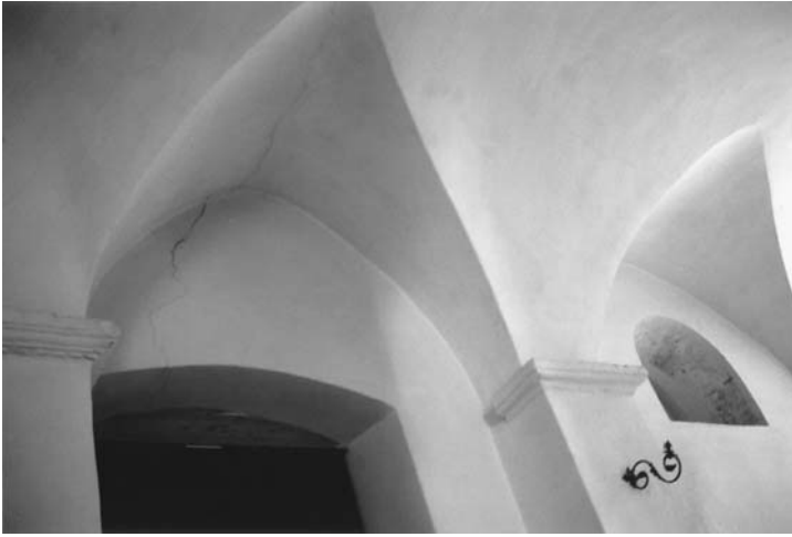
20. Corvey, abbey church, interior, westwork, ground floor, northern wall, pointed webs.
