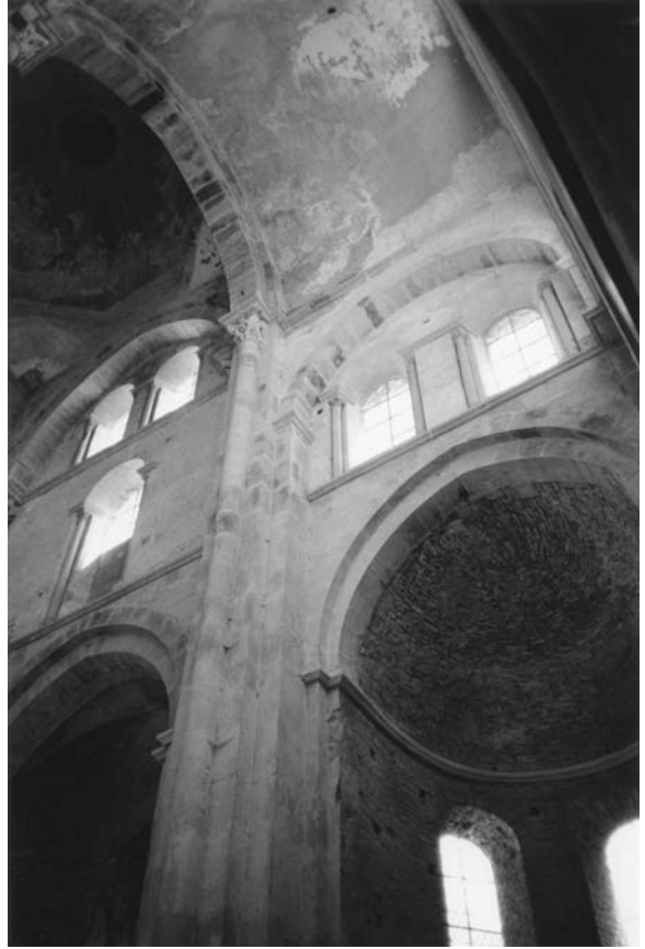
105. Cluny III, interior, southern transept, eastern wall, southern bay.
