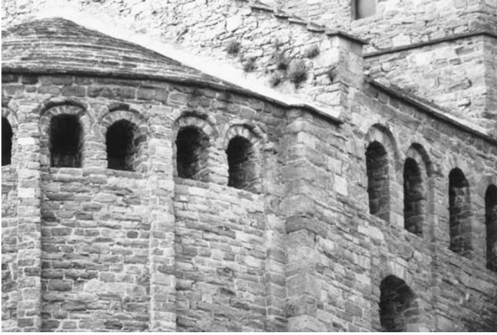
78. Cardona, Sant Vicenç, exterior, intersection of apse and northern choir wall; spur buttresses, voussoirs, and relieving cover stones.
