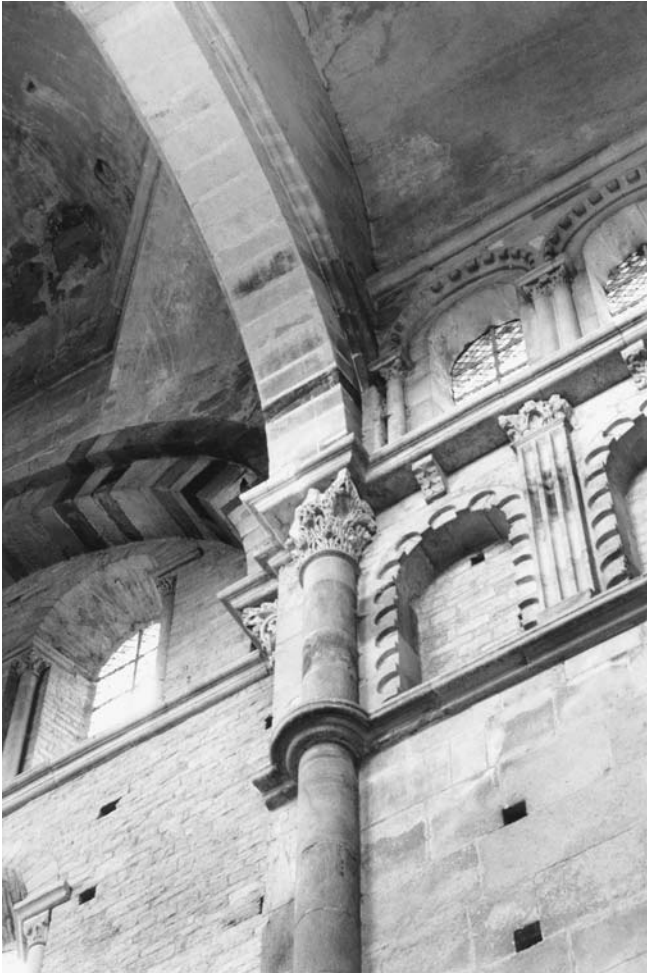
103. Cluny III, interior, southern transept, western wall, tower and northern bay, detail of squinch, transverse arch, and wall arches.
