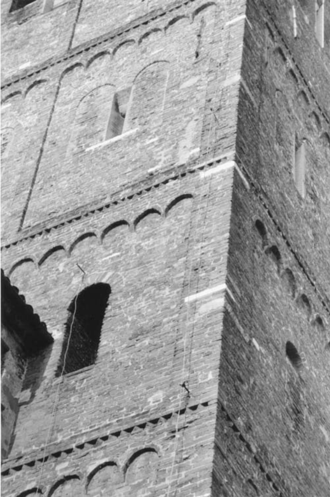
3. Novara, cathedral, exterior, northern transept tower, brickwork.
