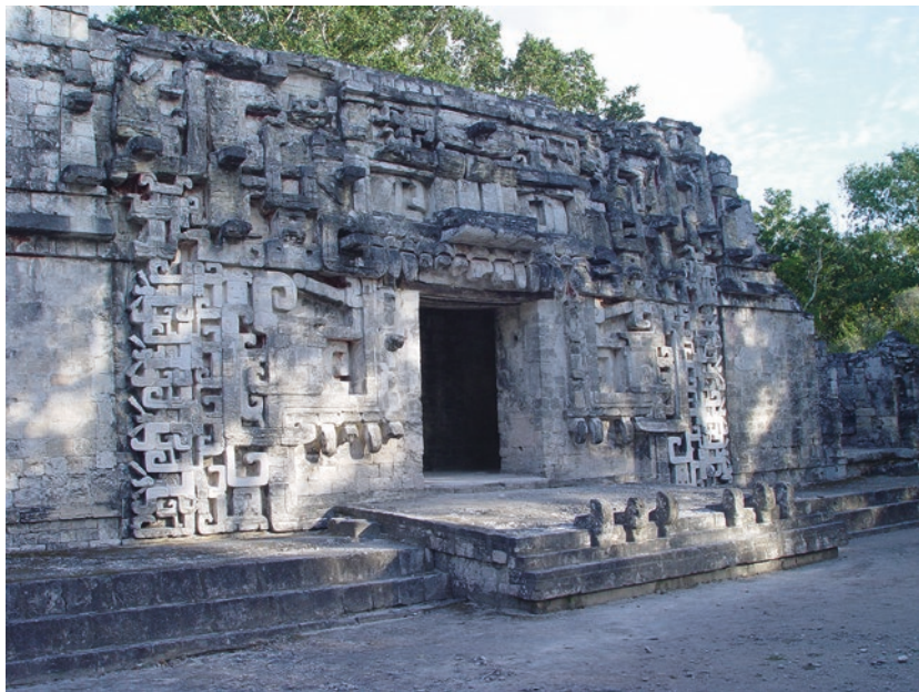
Fig. 3 Doorway in form of reptile mouth, Structure 2, Chicanná. Photo by John S. Henderson
