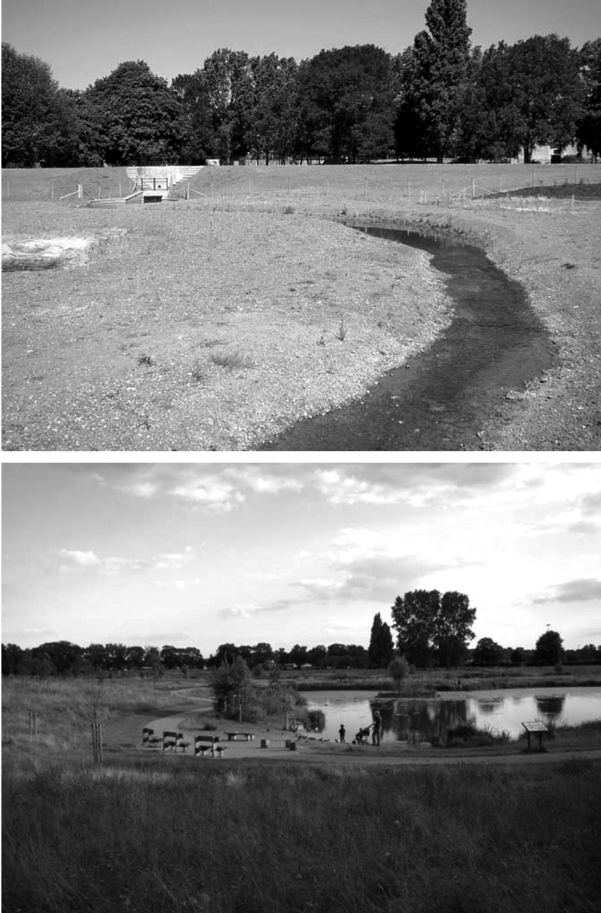
Figure 11.7 Daylighting Sutcliffe Park, south-east London, UK
