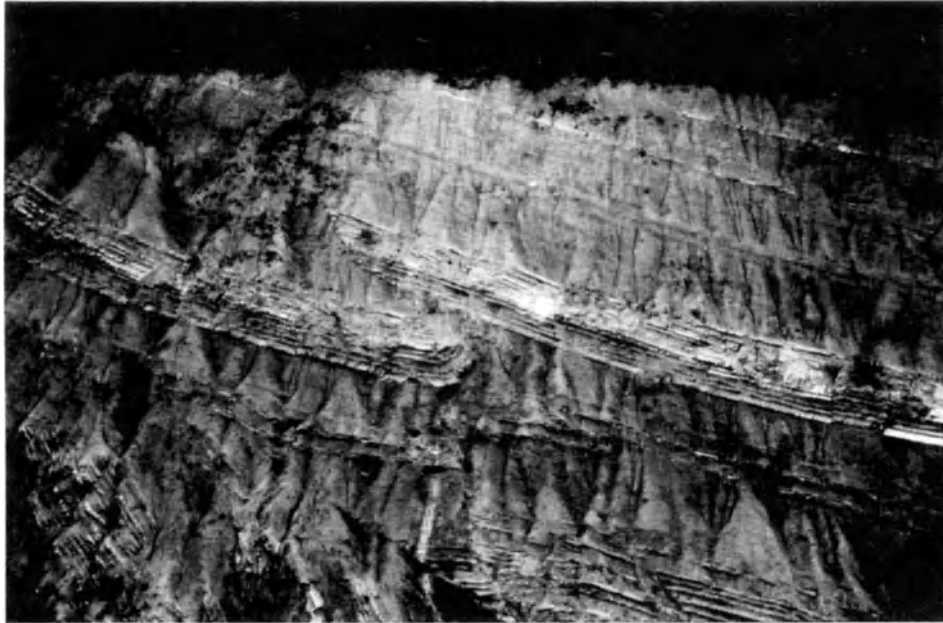
Figure 4. Thrust structures seen in a quarry face of limestones and marls at Holderbank (30 km WNW Zürich, Switzerland) with passive hanging wall and deformed footwall (cf Fig. 2B, Model 2).
